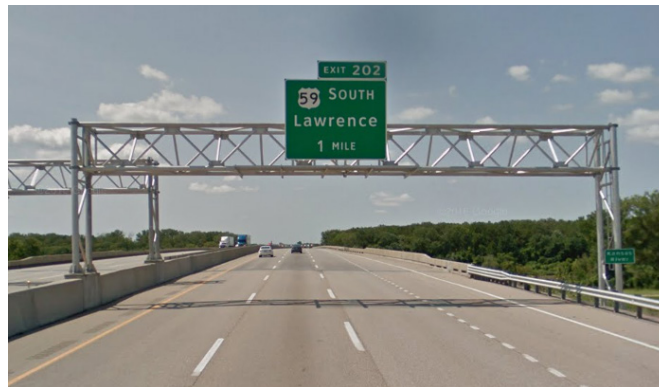
Figure 1.1: Bridge-Type Overhead Truss Sign Structure (OHTSS)
