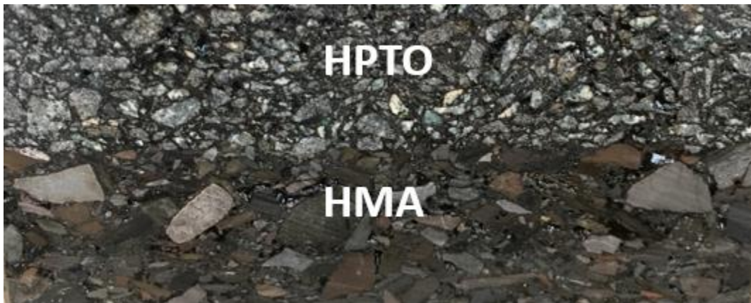
Figure 3. Thin-Overlay Applied to HMA.
