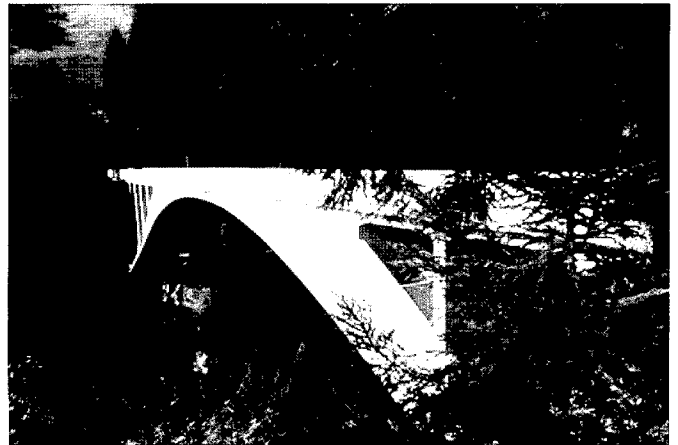
Figure 1. The Salginatobel Arch Bridge, with its reinforced concrete arch, was built in 1929 in Switzerland by Robert Maillart.
