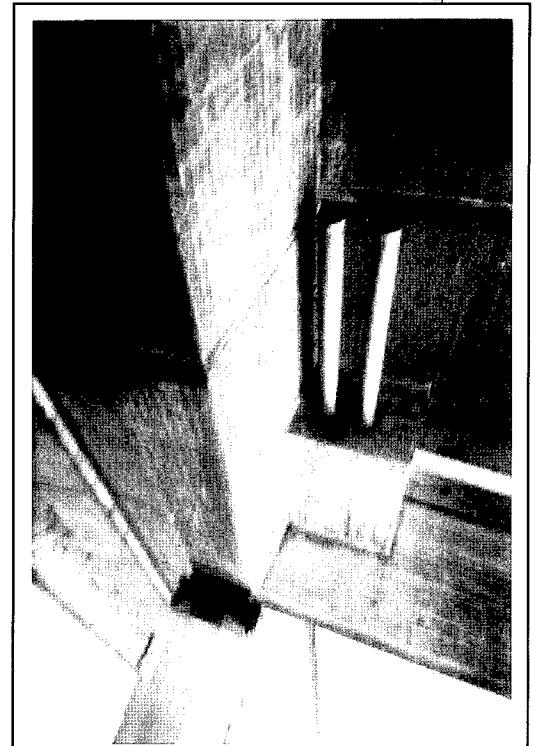
Figure 24. Anchor block for external tendon retrofit to continuous, post-tensioned concrete viaduct (L124 extension of A59), near Cologne, originally built with tendon coupling joints at the quarter points.
