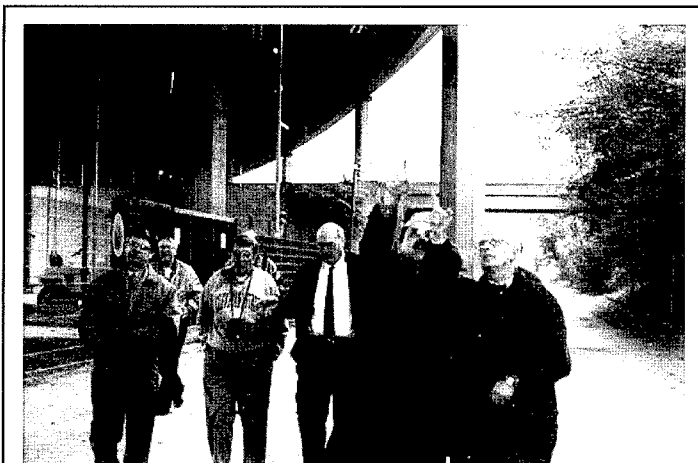
Figure 25. German hosts and members of the scan team examine the external tendon retrofit to the L124 viaduct near Cologne.
