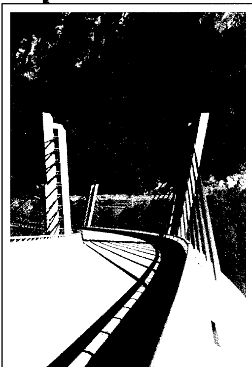
Figure 6. On the Sunniberg Bridge, short pylons rise away from the deck to accommodate the curve of the highway.
