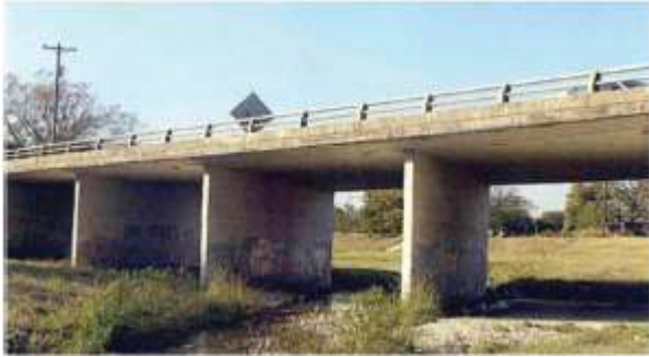
Figure 1-Slab Bridge
