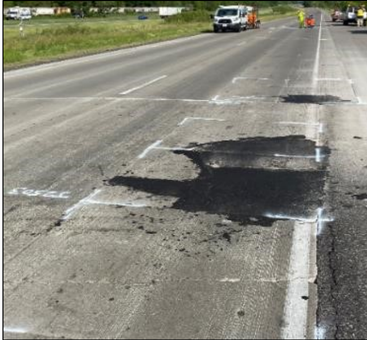
Figure 3-11. Cell 506 before replacement on June 2020.
