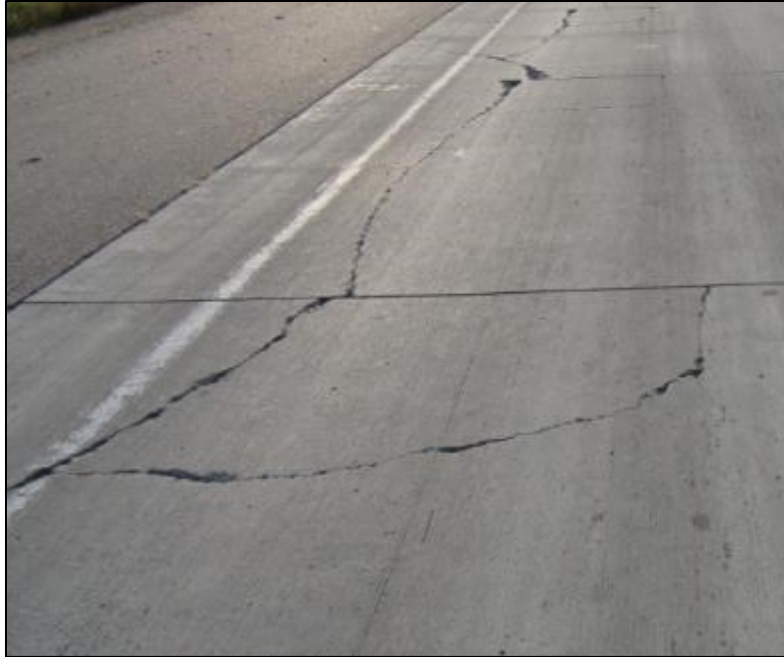
Figure 3-21. Photograph of Cell 705 before replacement on September 2020.
