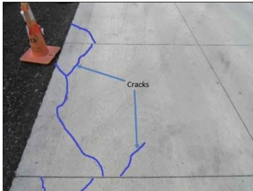
Figure 3-1. Cell 139 after exposure to construction trucks.
