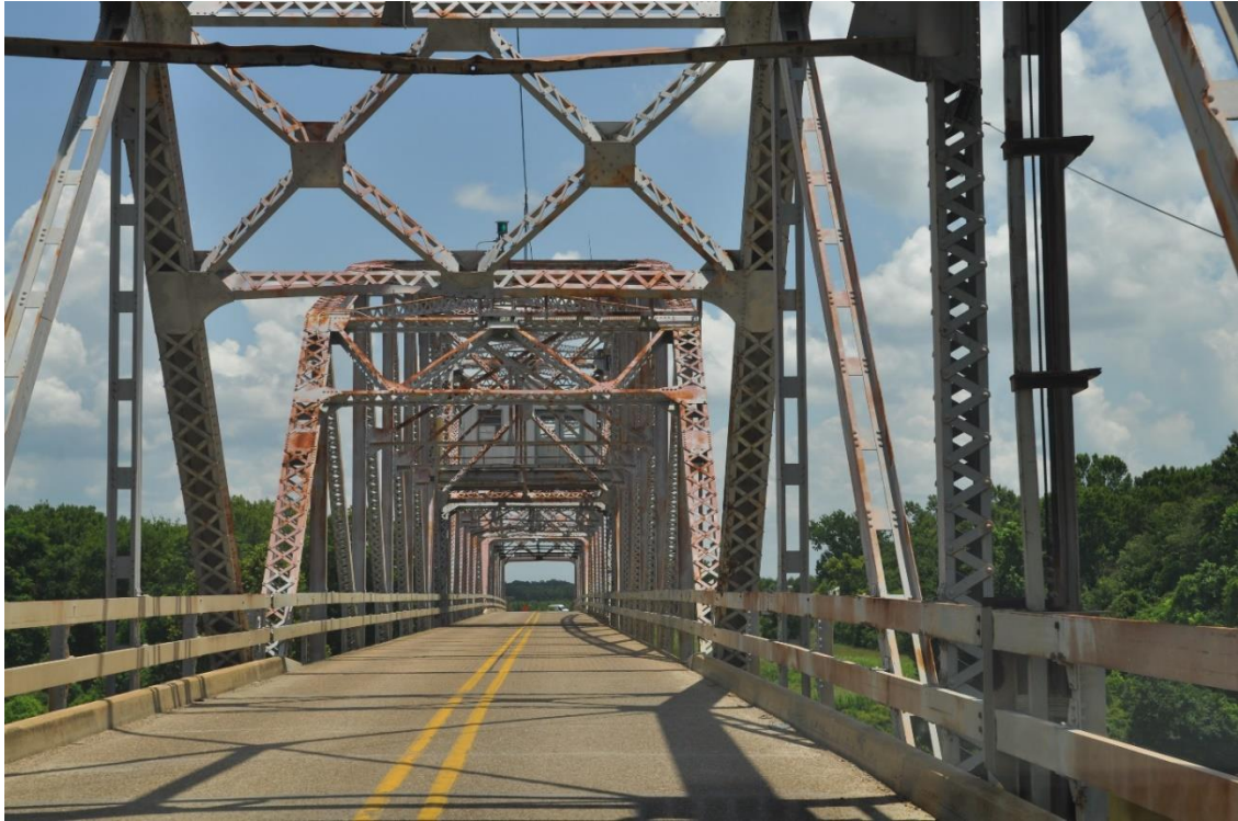
Figure 6. Existing LA-8 bridge
