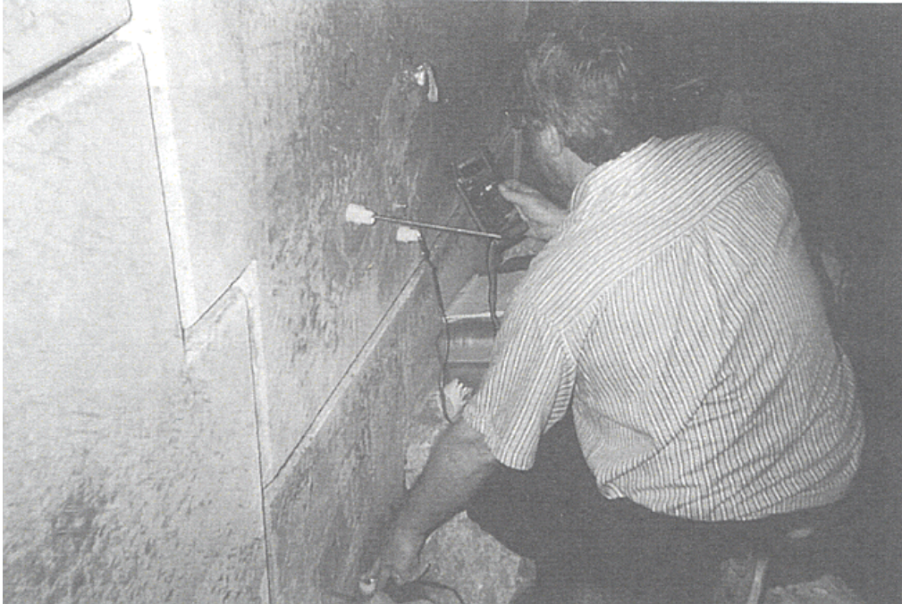
Figure 9. A portable Copper/Copper Sulfate half cell is hand held on the soil at the base of the wall as a reference electrode for multi-meter testing of electric potential.
