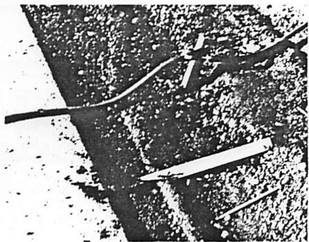
Figure 3. Roadtube Installation, Near Side Without Curbs
