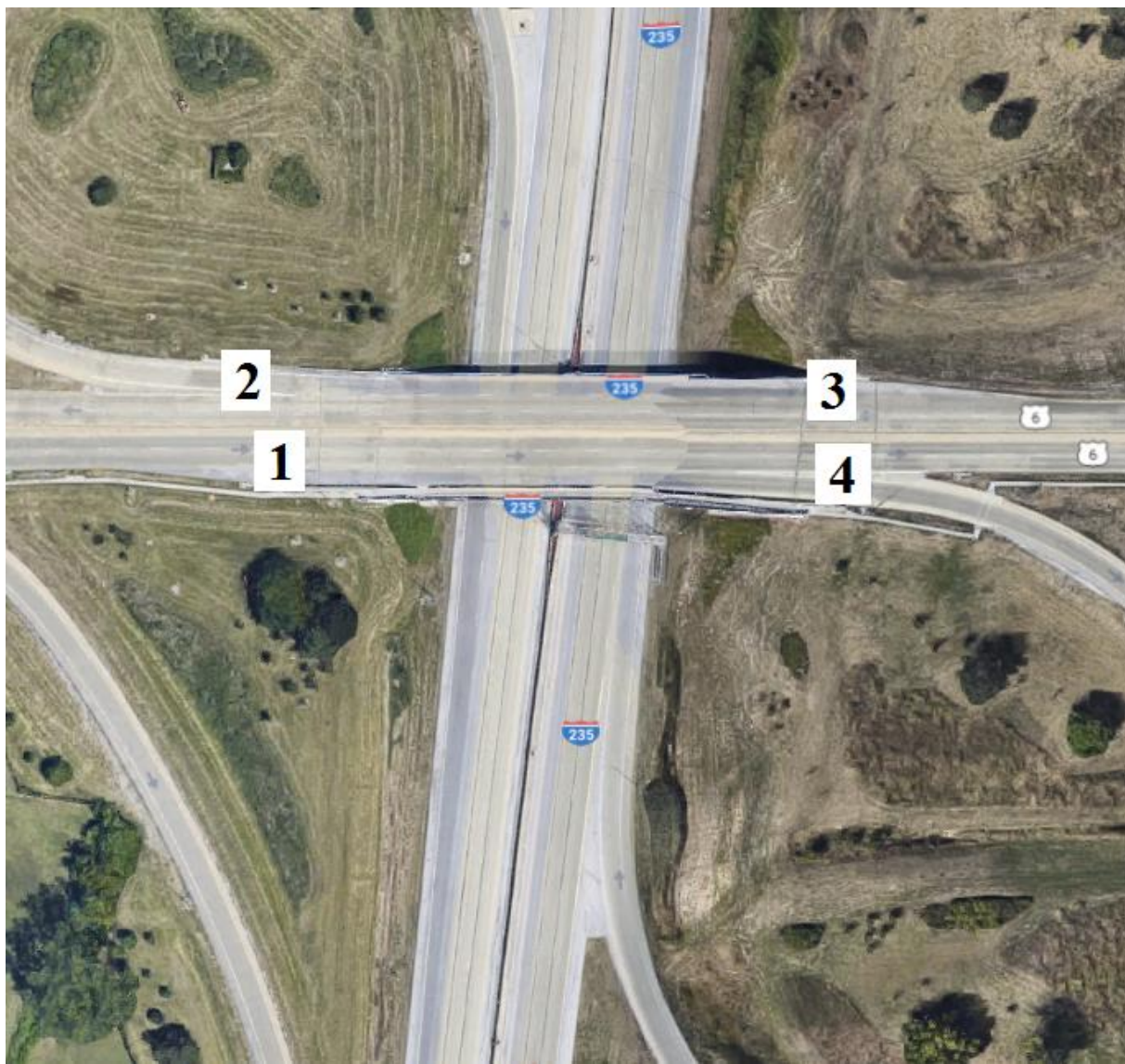
Figure B-144. Bridge No. 7738.9S006 [1]
