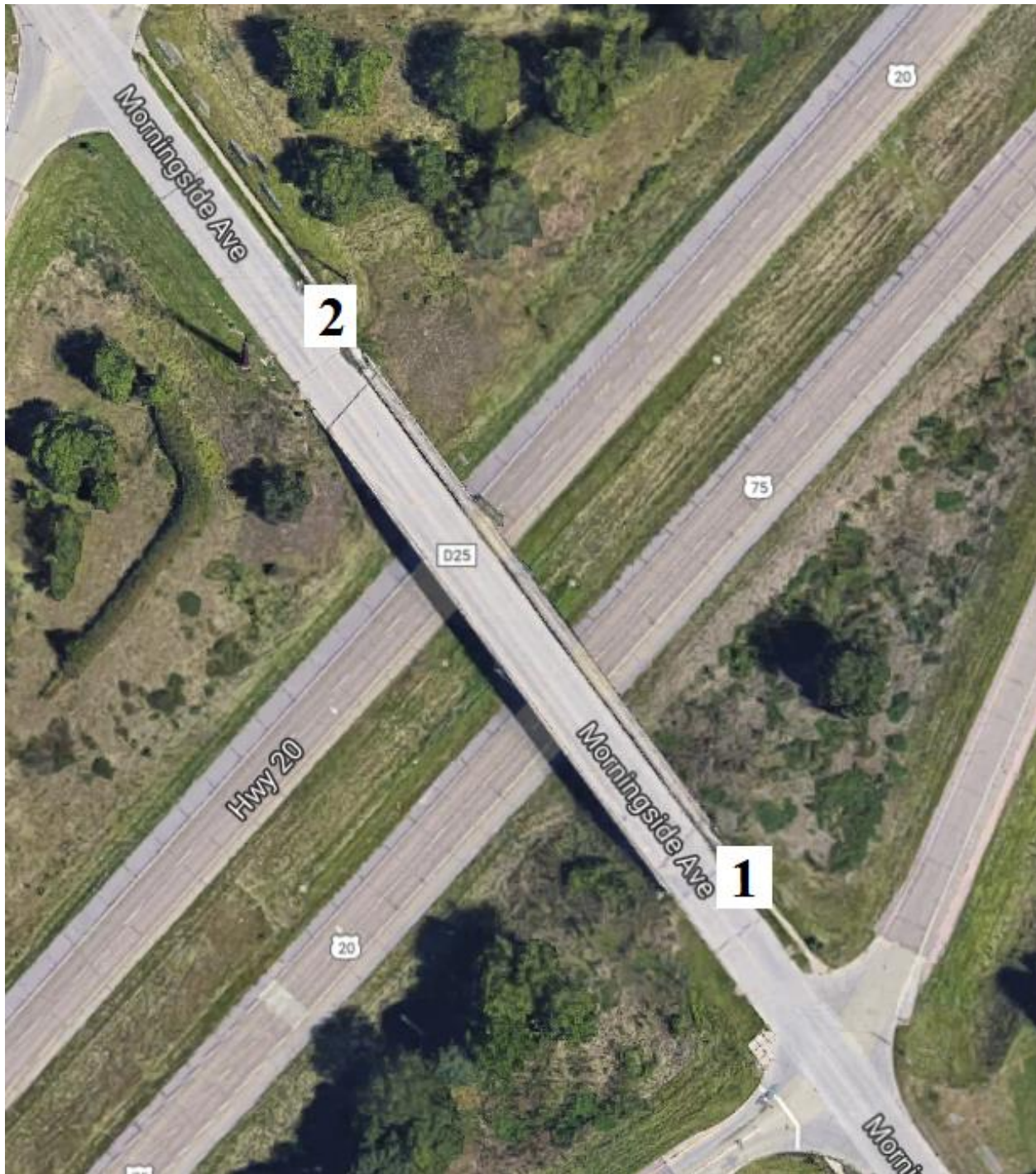
Figure B-180. Bridge No. 9703.4O020 [1]
