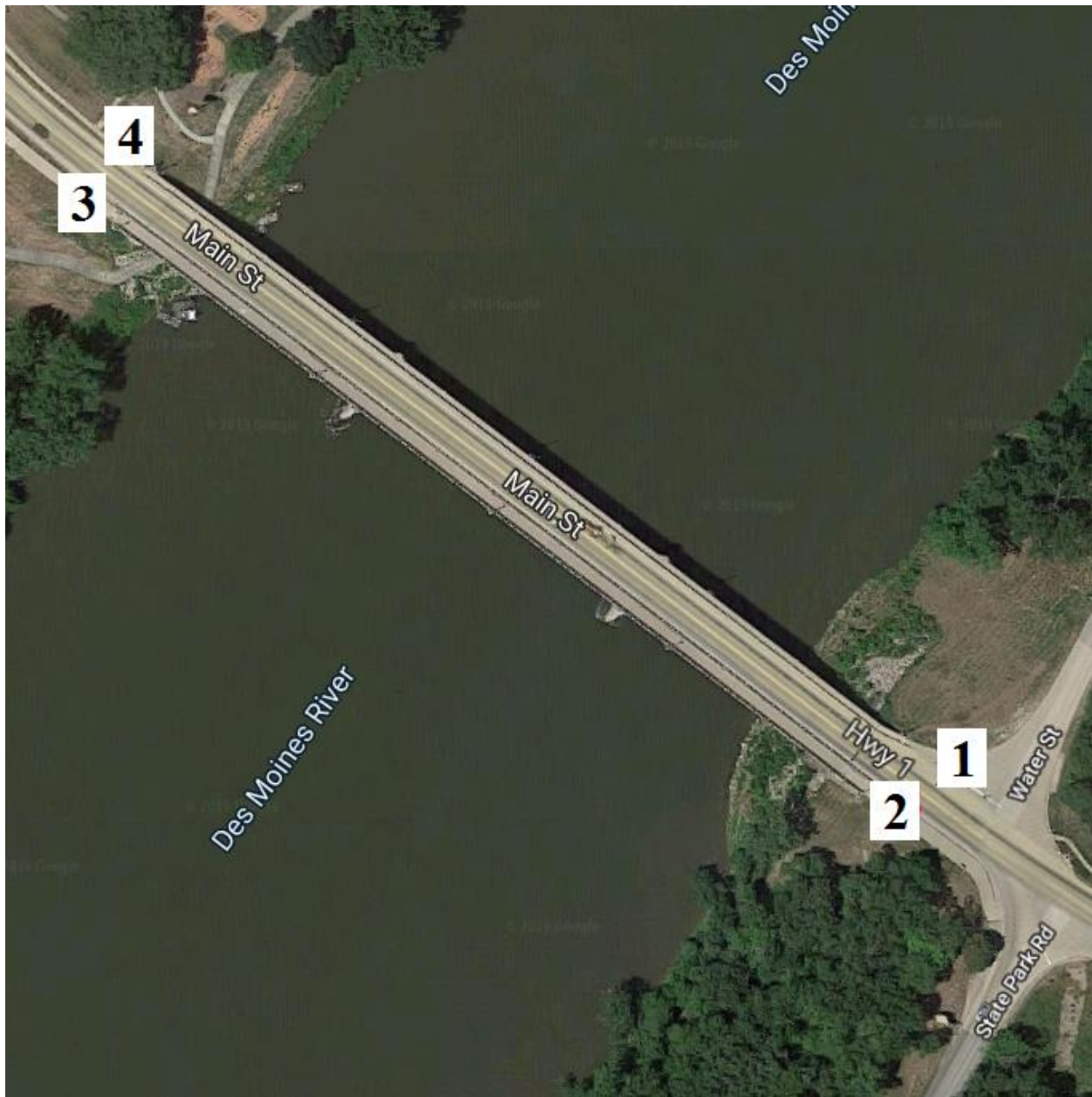
Figure B-168. Bridge No. 8903.8S001 [1]
