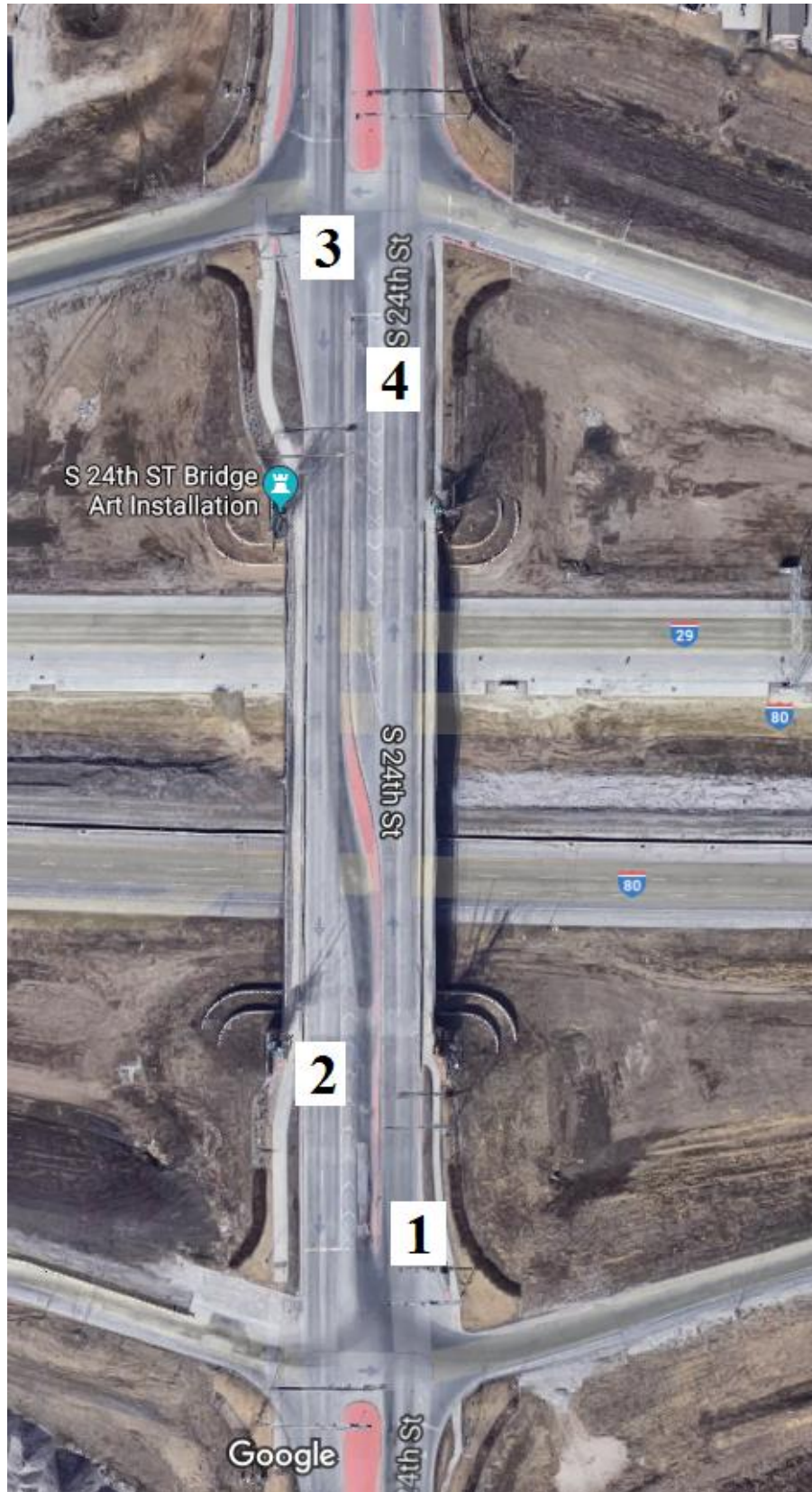
Figure B-148. Bridge No. 7801.7O080 [1]
