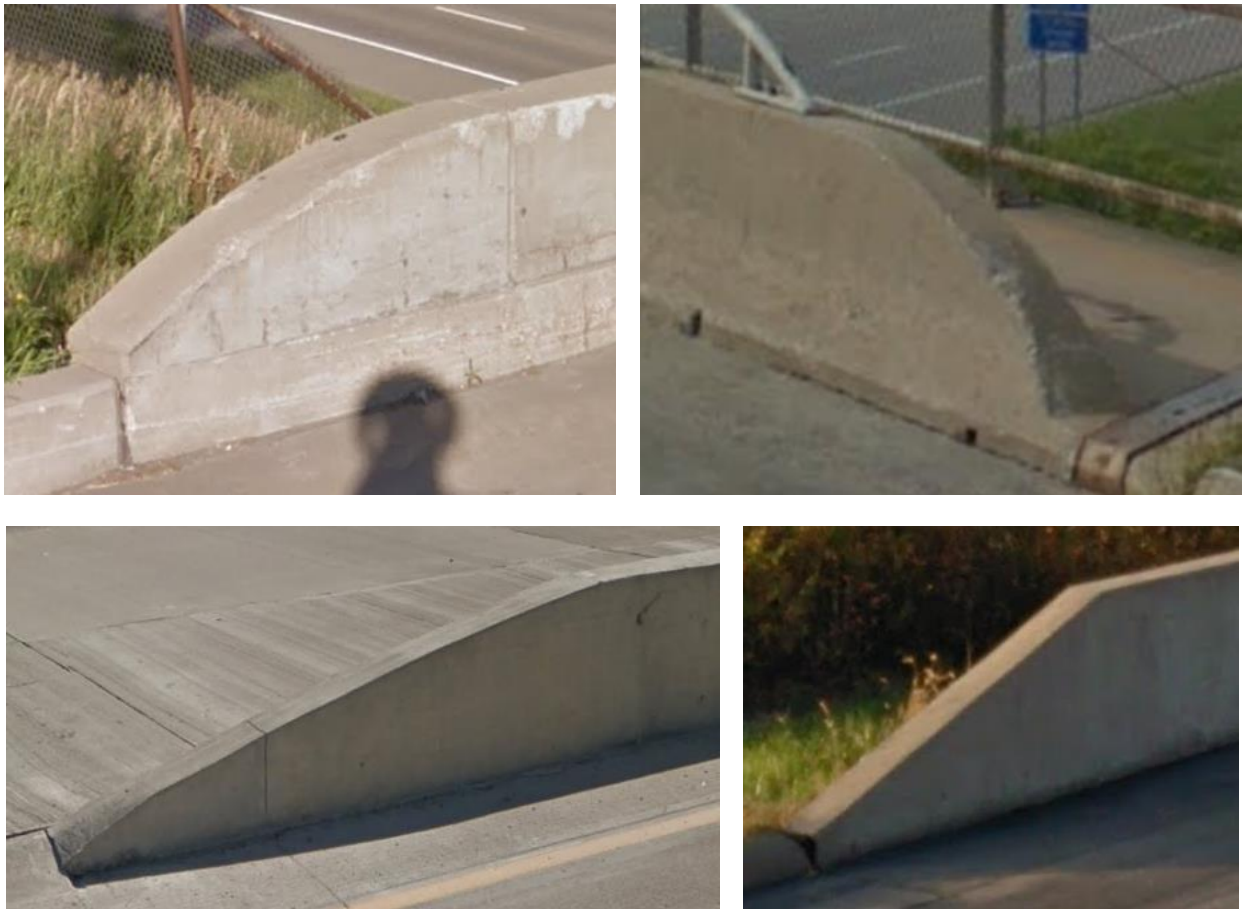
Figure 1. Examples of Concrete Sloped End Treatments in Iowa [1]
