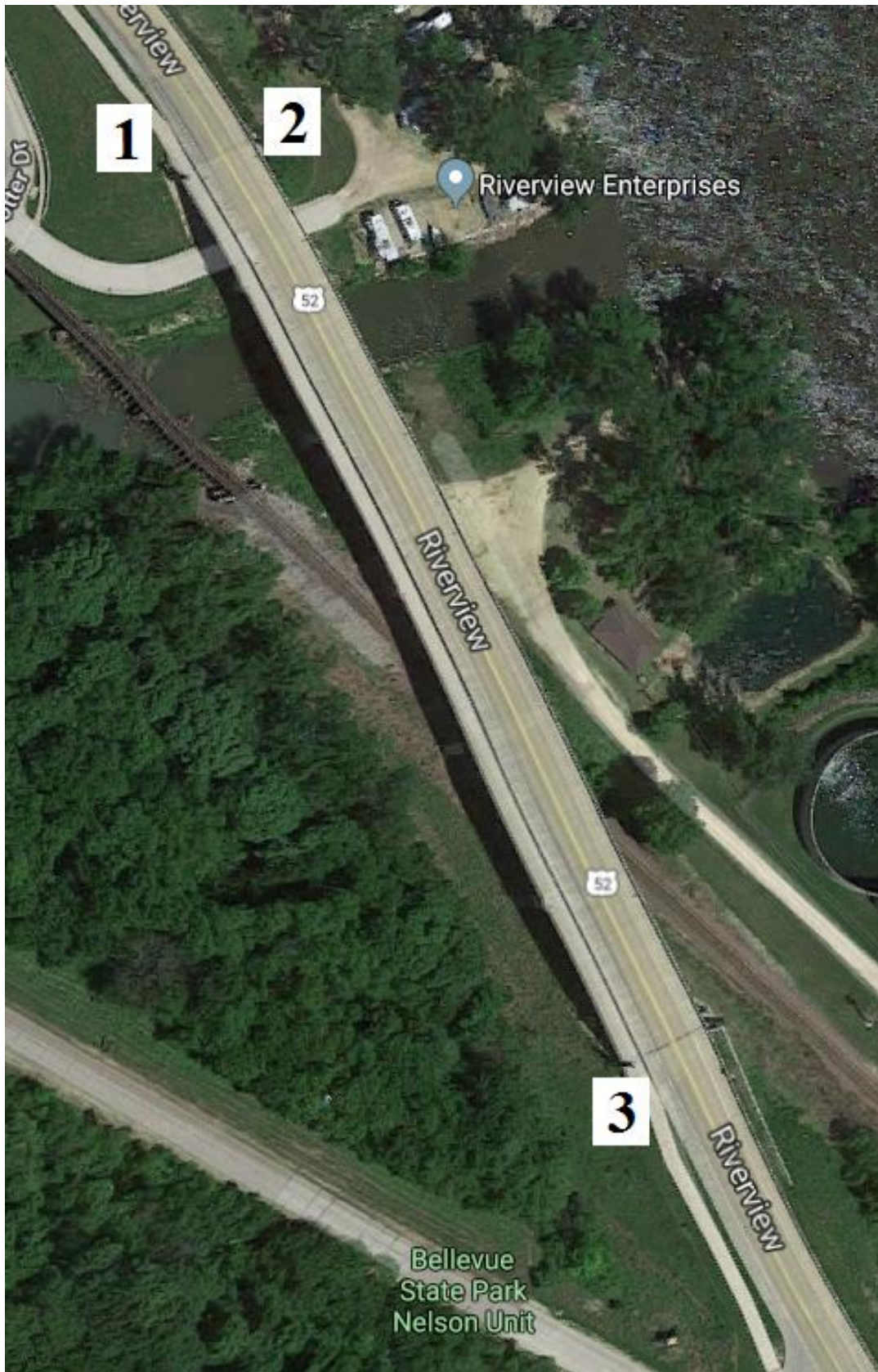
Figure B-73. Bridge No. 4922.8S052 [1]
