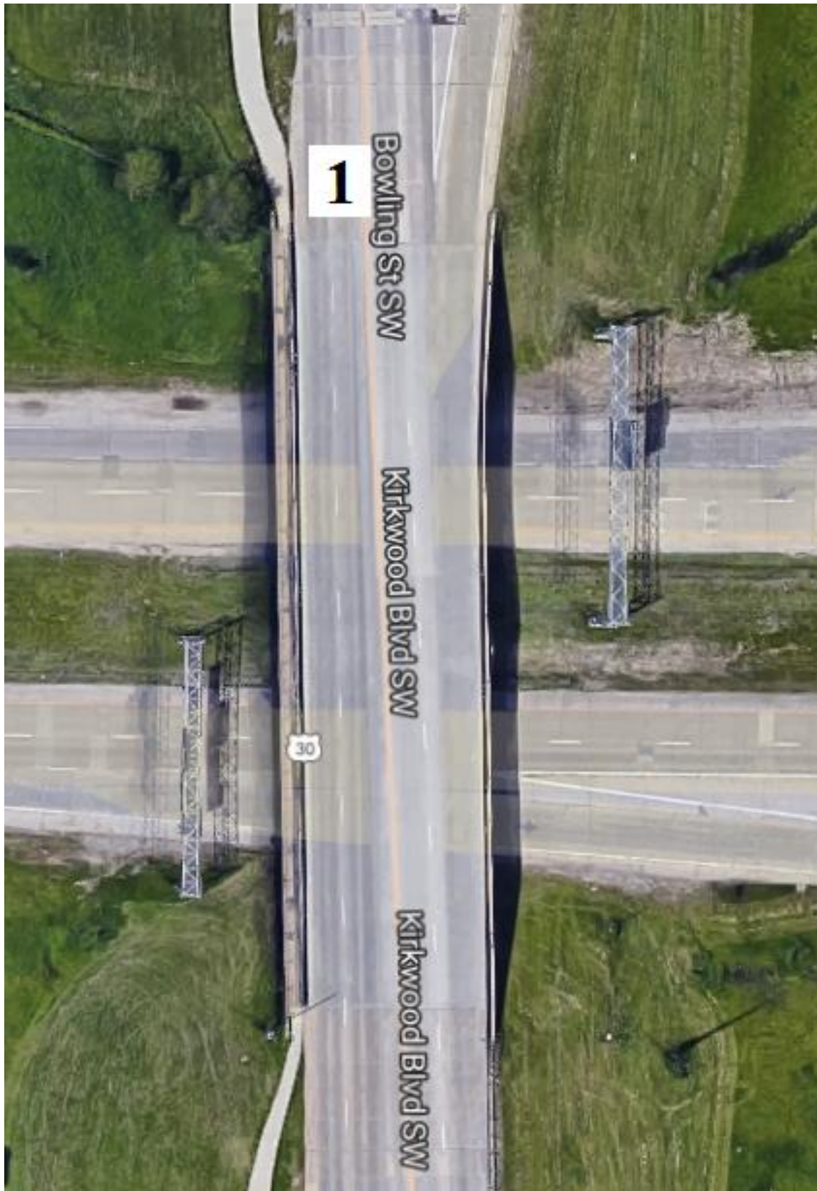
Figure B-100. Bridge No. 5753.4O030 [1]
