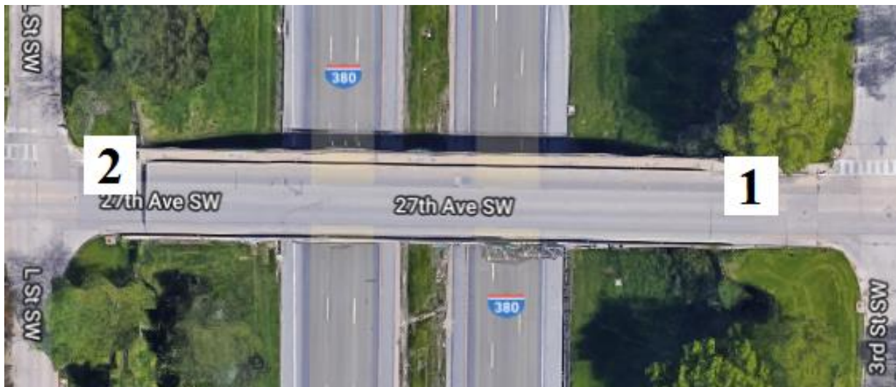
Figure B-90. Bridge No. 5718.0O380 [1]
