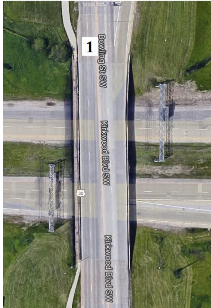
Figure 71. Bridge No. 5753.4O030 [1]
