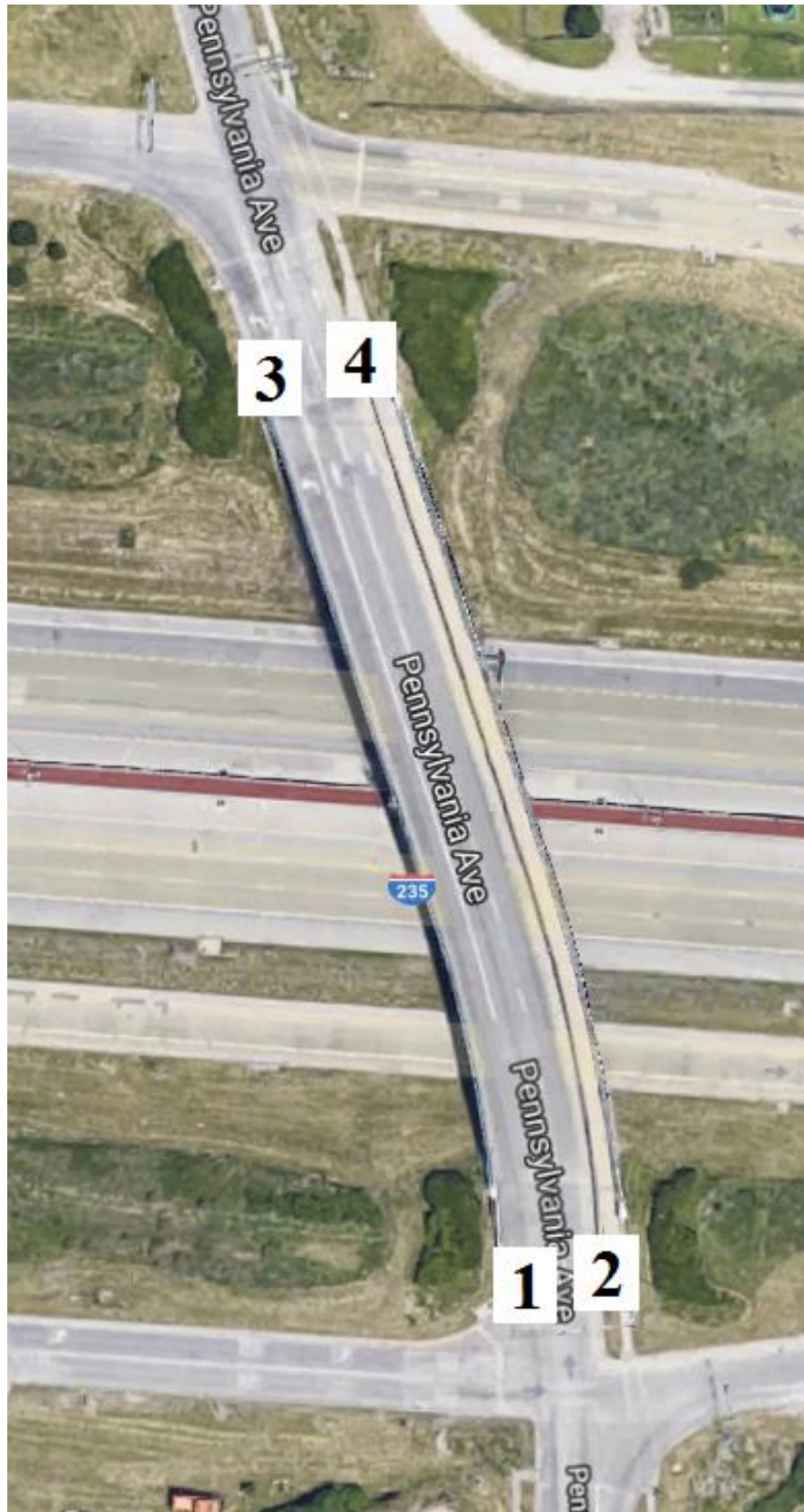
Figure B-132. Bridge No. 7708.9O235 [1]
