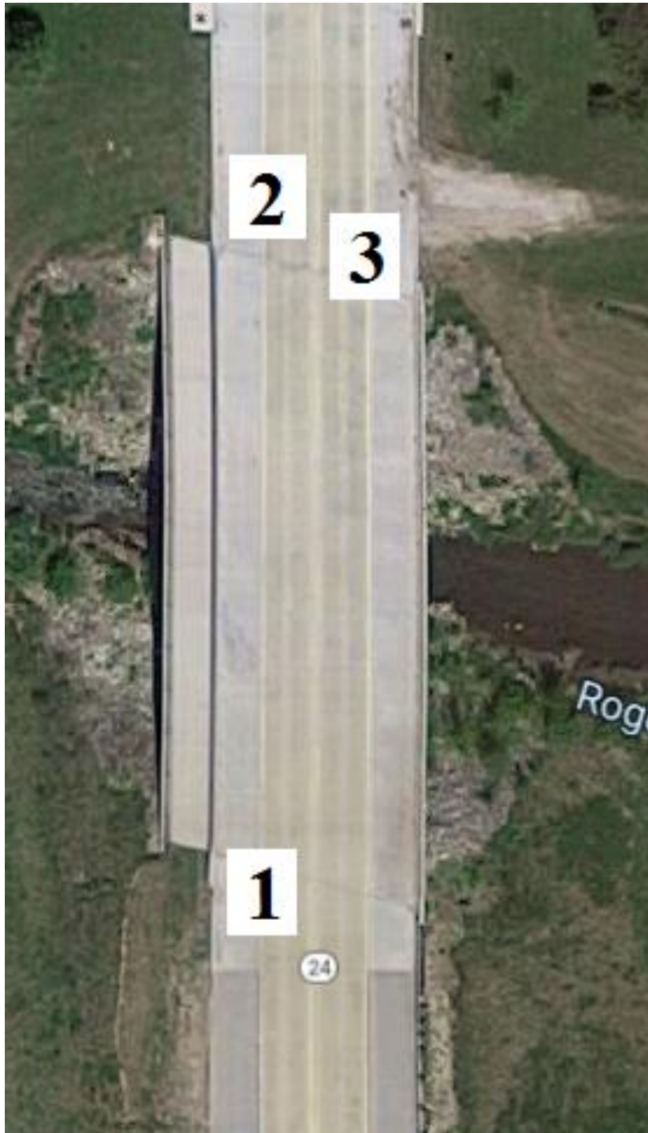
Figure B-176. Bridge No. 9621.3S024 [1]
