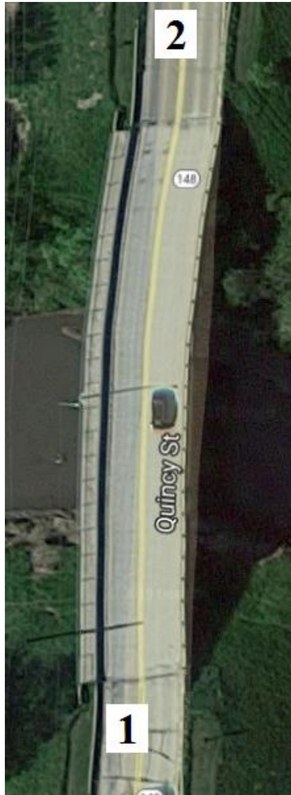
Figure B-1. Bridge No. 0230.3S148 [1]
