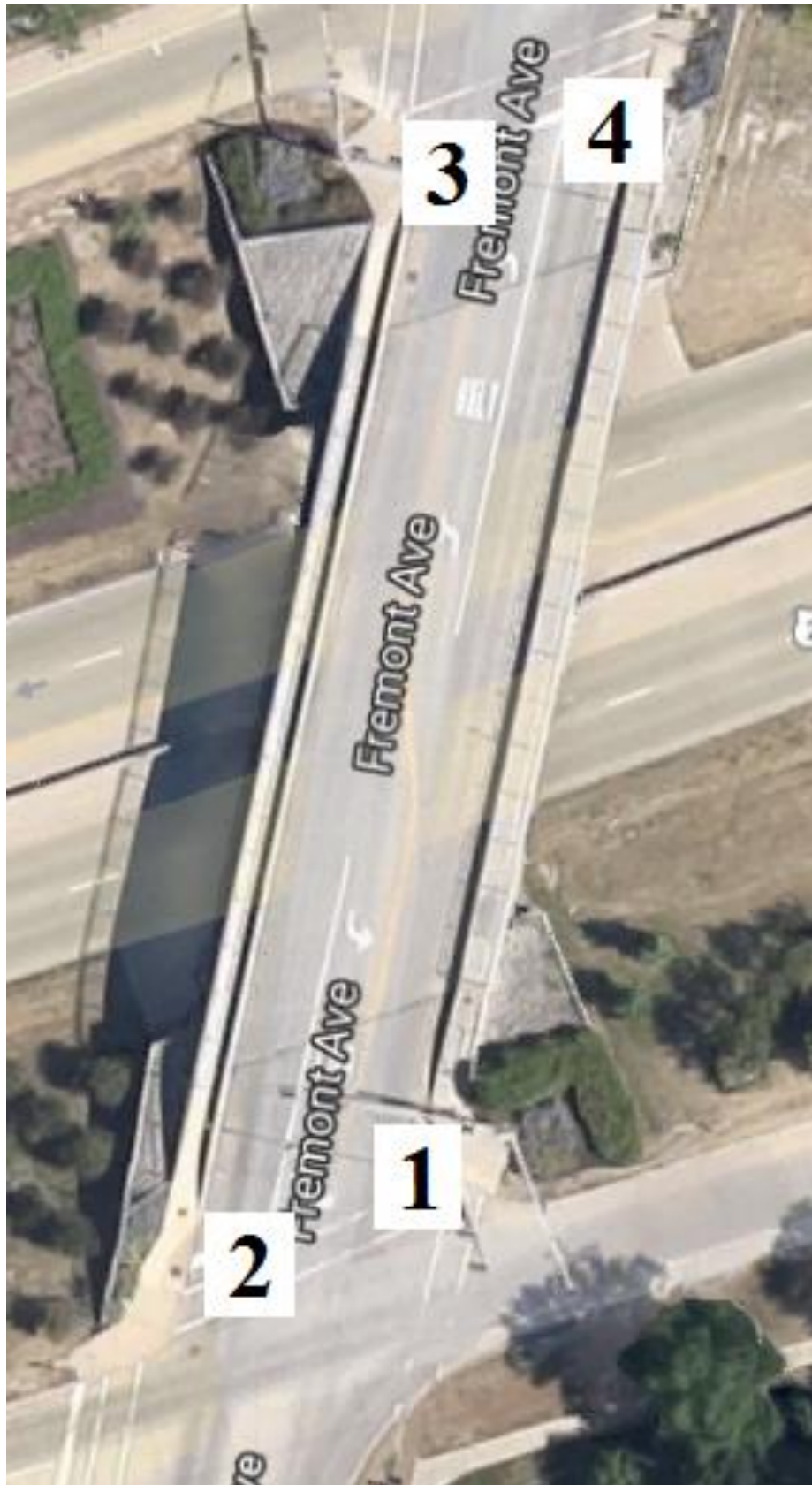
Figure B-49. Bridge No. 3118.4O020 [1]
