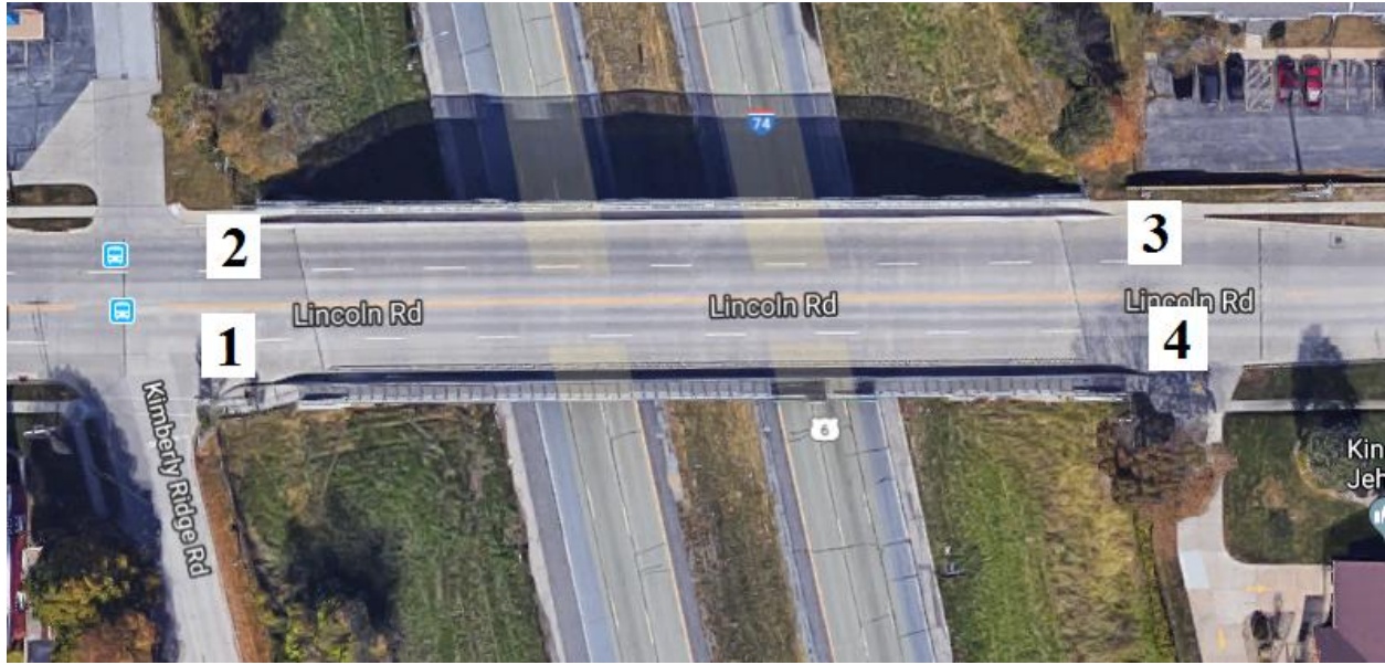
Figure B-151. Bridge No. 8203.8O074 [1]
