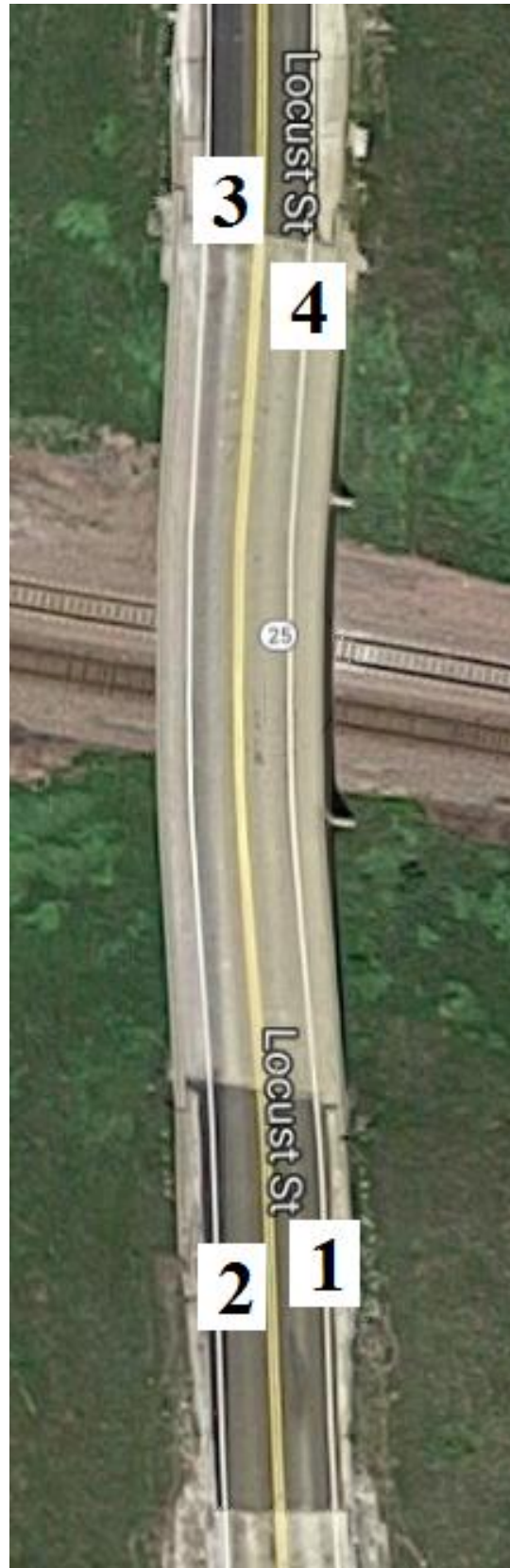
Figure B-62. Bridge No. 3712.2S025 [1]
