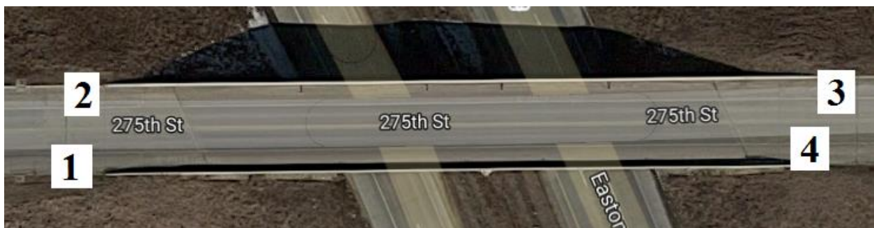
Figure B-15. Bridge No. 0995.4O218 [1]
