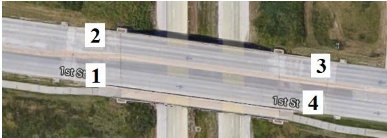
Figure B-183. Bridge No. 9741.2O029 [1]
