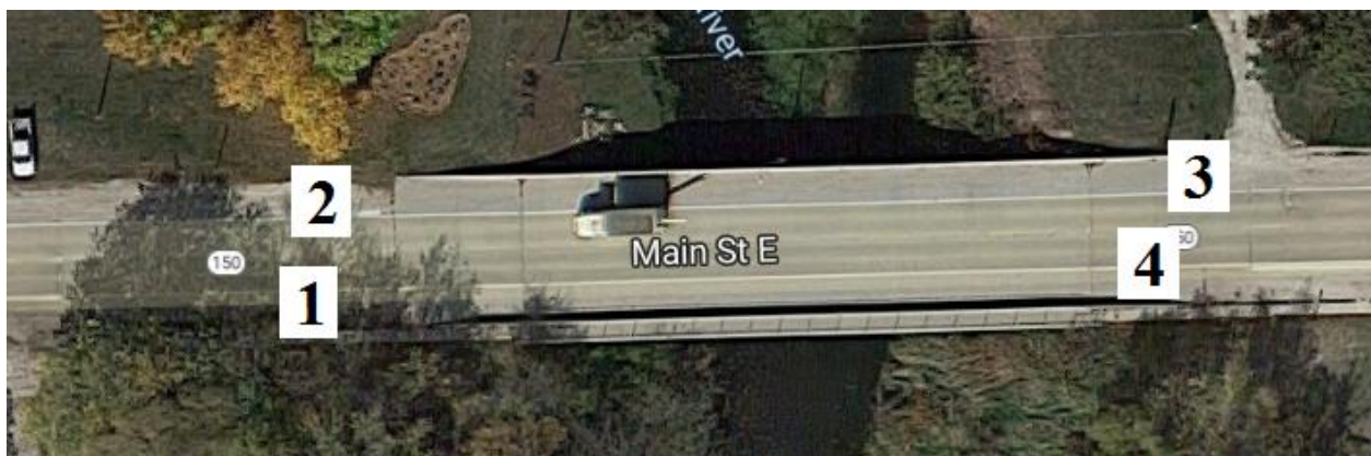
Figure B-58. Bridge No. 3364.6S150 [1]
