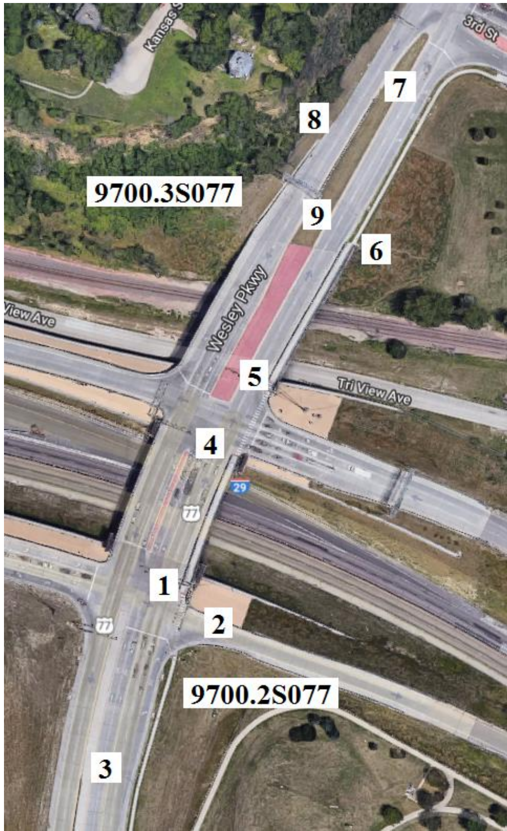
Figure B-178. Bridge Nos. 9700.2S077 and 9700.3S077[1]
