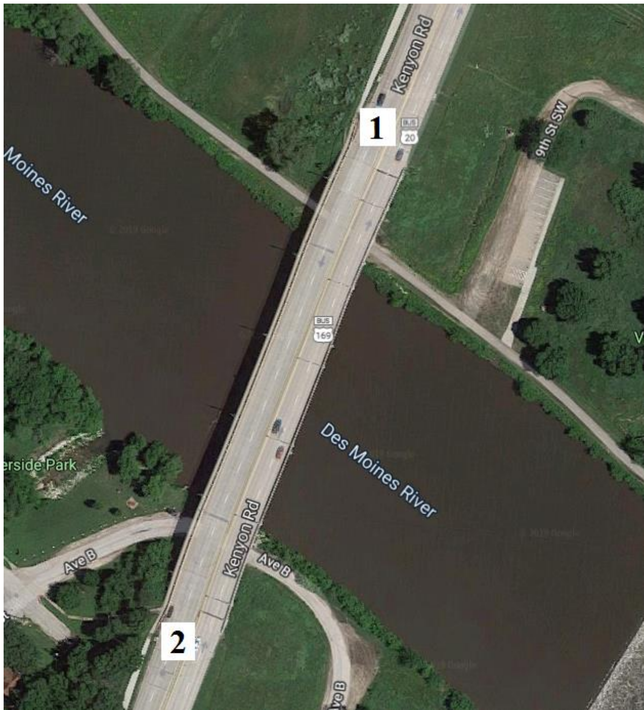
Figure B-173. Bridge No. 9401.3L926 [1]
