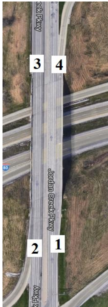
Figure B-32. Bridge No. 2521.4O080 [1]
