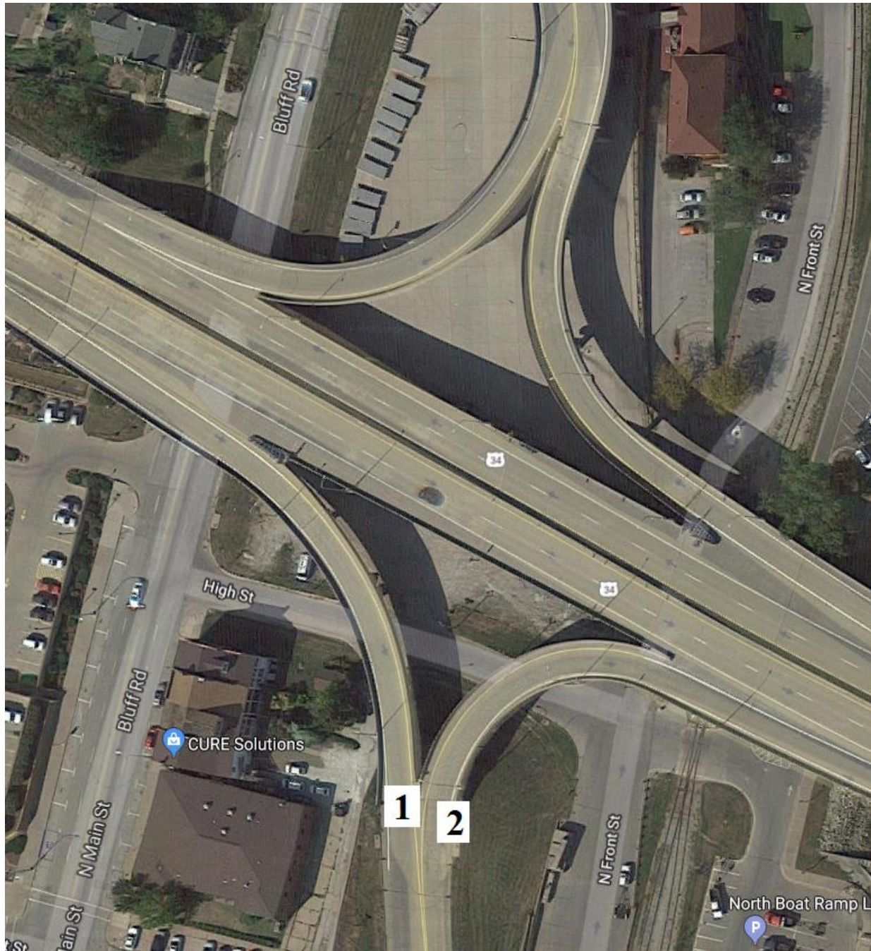
Figure 85. Bridge No. 2963.7A034 [1]
