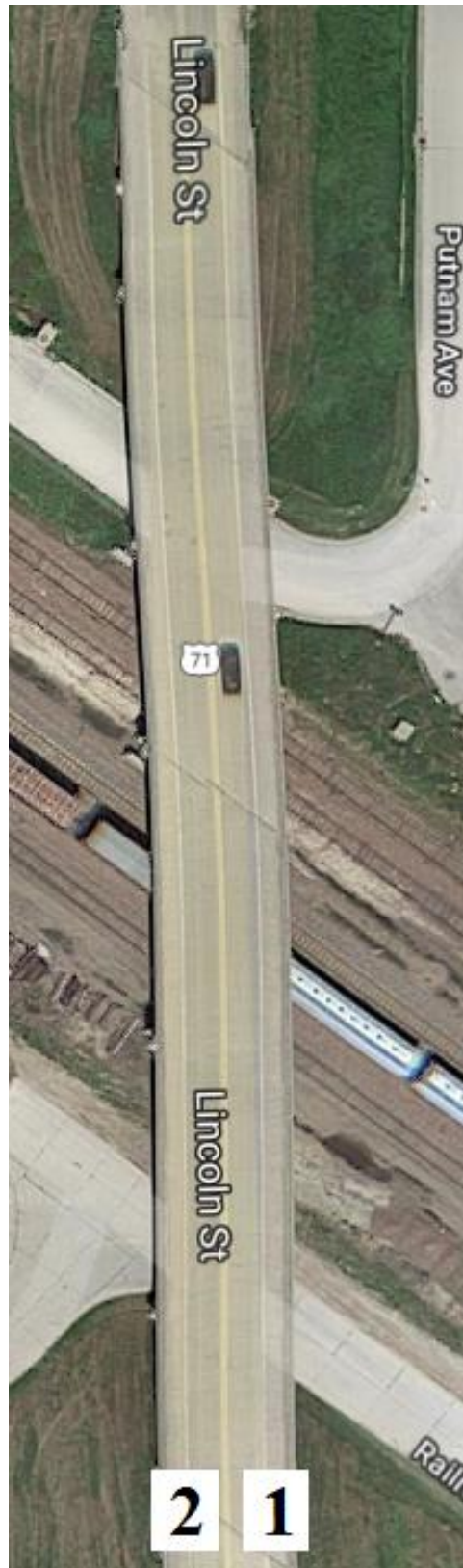
Figure B-18. Bridge No. 1412.0S071 [1]
