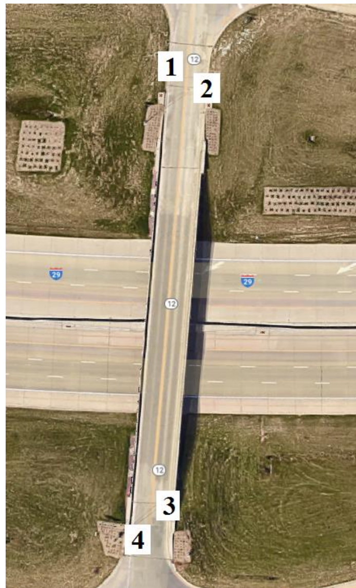
Figure B-182. Bridge No. 9708.1S012 [1]
