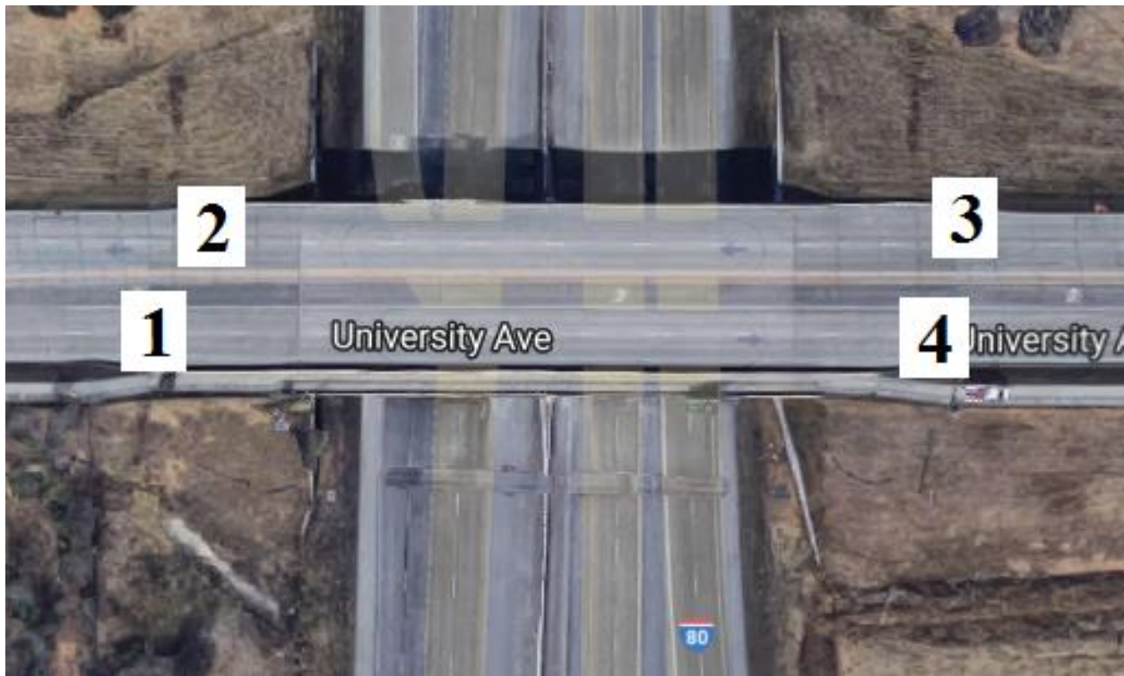
Figure B-140. Bridge No. 7724.1O080 [1]
