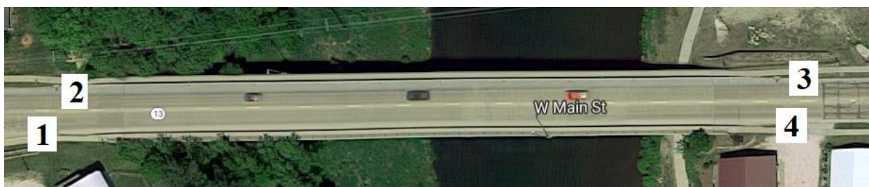
Figure B-38. Bridge No. 2841.6S013 [1]
