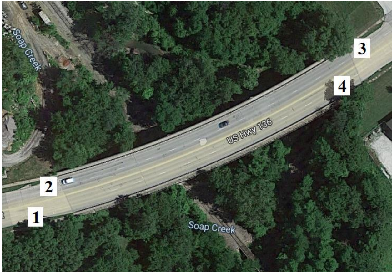
Figure B-89. Bridge No. 5602.4S136 [1]
