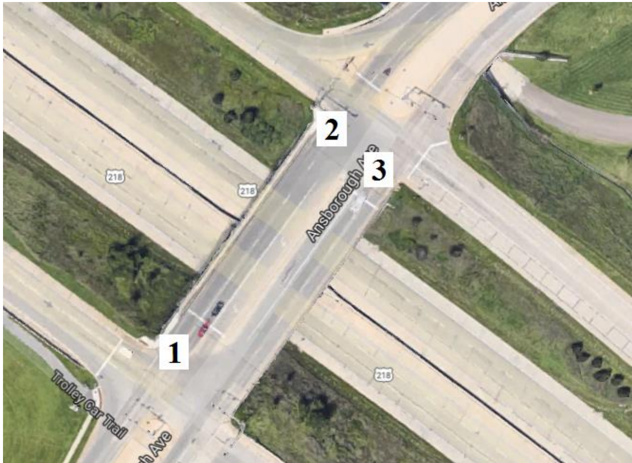
Figure B-14. Bridge No. 0783.2O218 [1]
