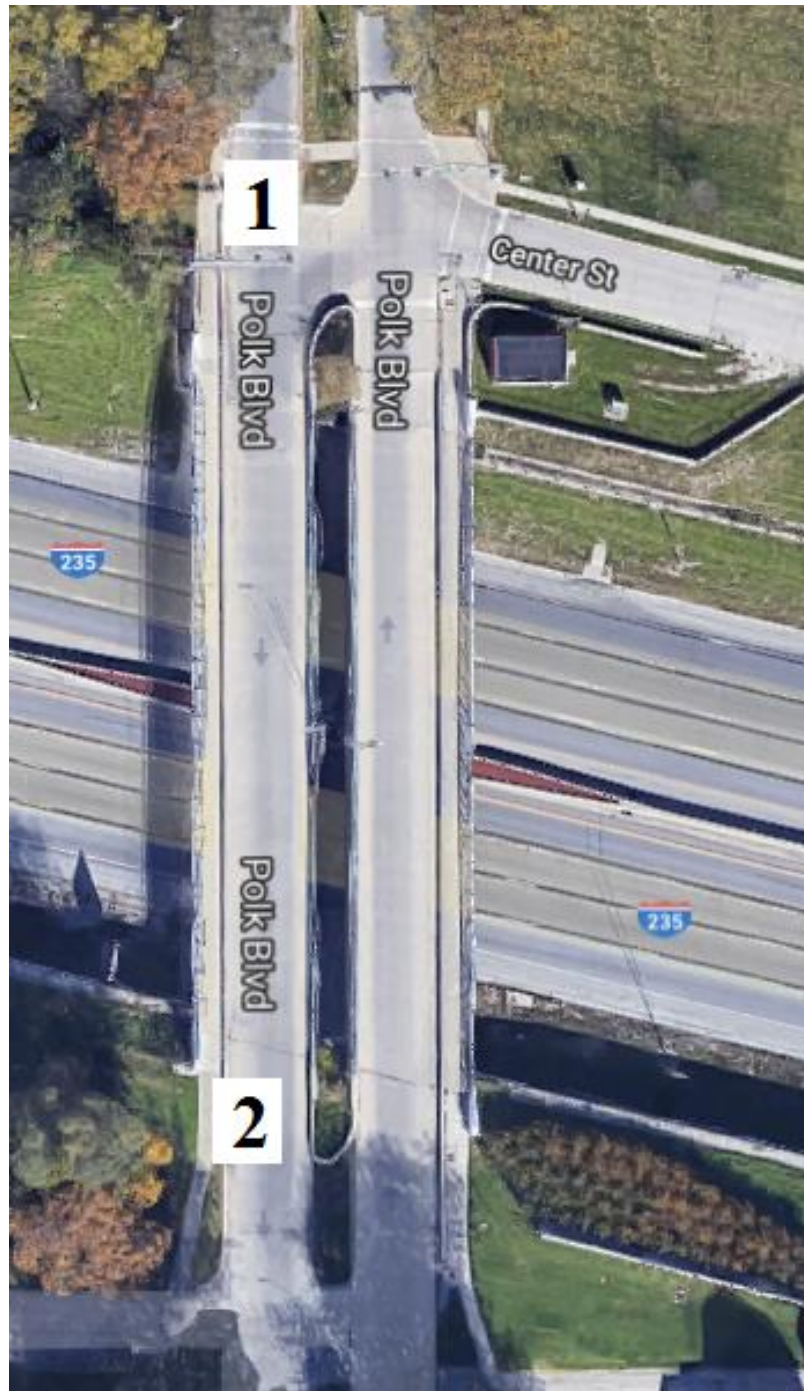
Figure 159. Bridge No. 7705.00235 with Sloped End Treatments Labeled [1]
