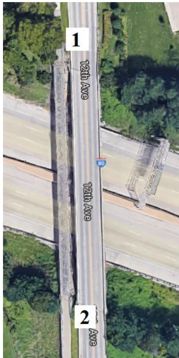
Figure 157. Bridge No. 5242.1O080 with Sloped End Treatments Labeled [1]
