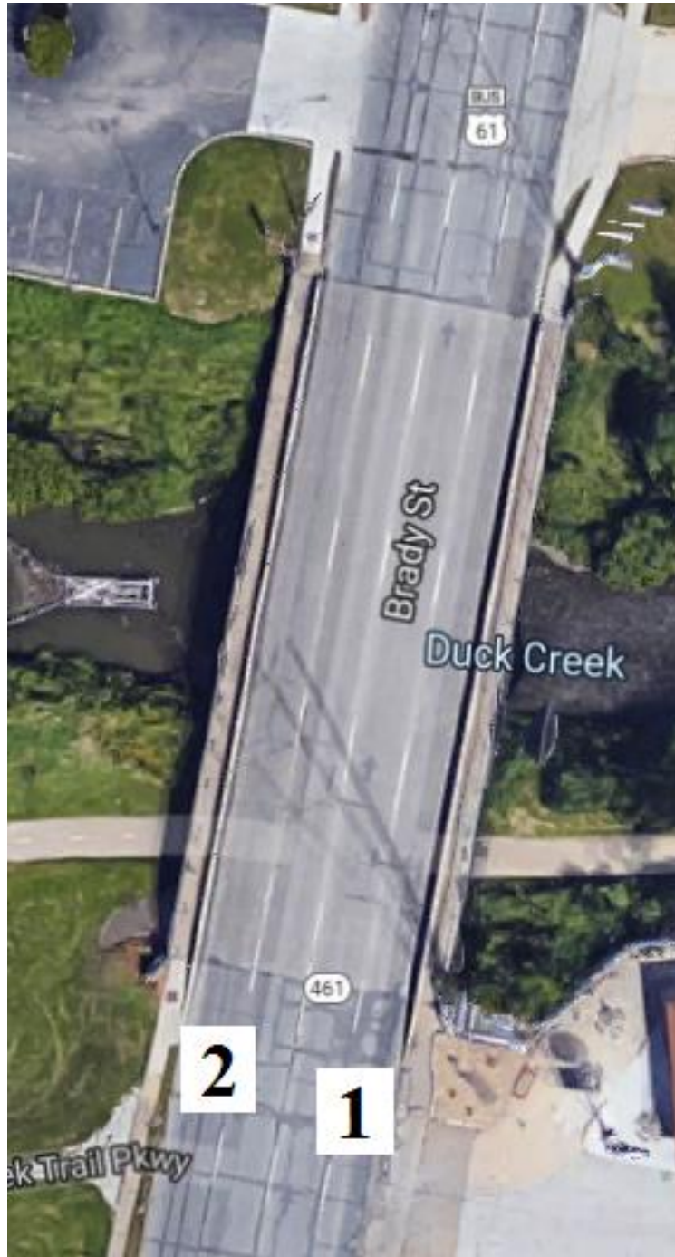
Figure 84. Bridge No. 8220.1R061 [1]
