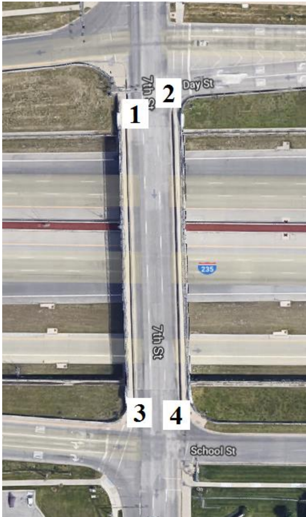
Figure B-126. Bridge No. 7707.9O235 [1]
