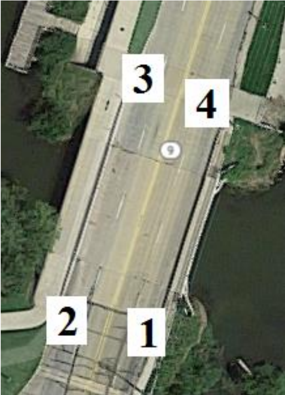
Figure B-48. Bridge No. 3026.6S071 [1]
