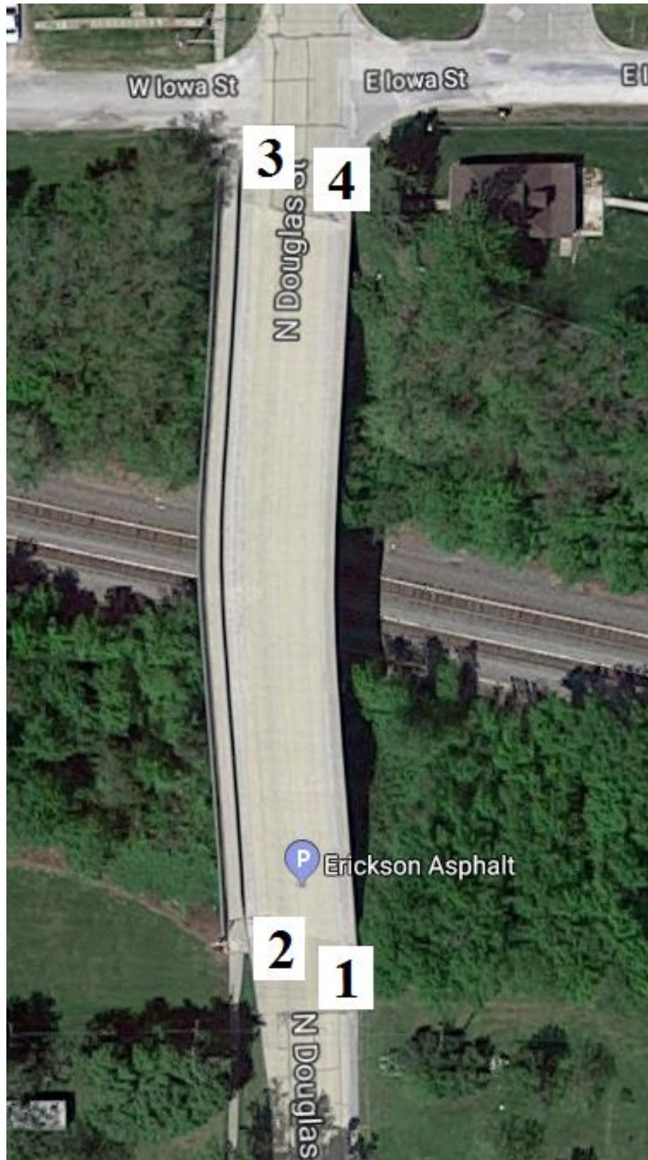
Figure B-167. Bridge No. 8840.0S169 [1]
