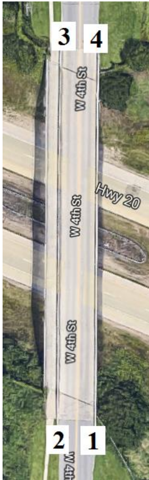
Figure B-6. Bridge No. 0728.00020 [1]
