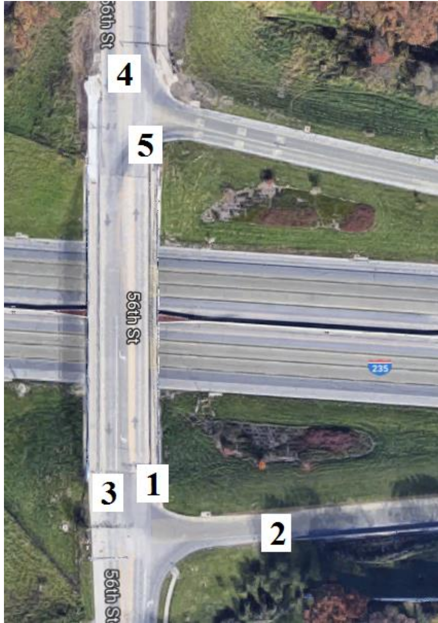
Figure 76. Bridge No. 7704.4O235 [1]
