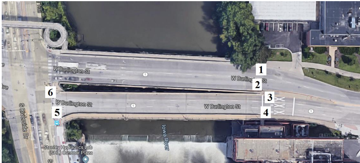
Figure 80. Bridge No. 5285.9L001 [1]
