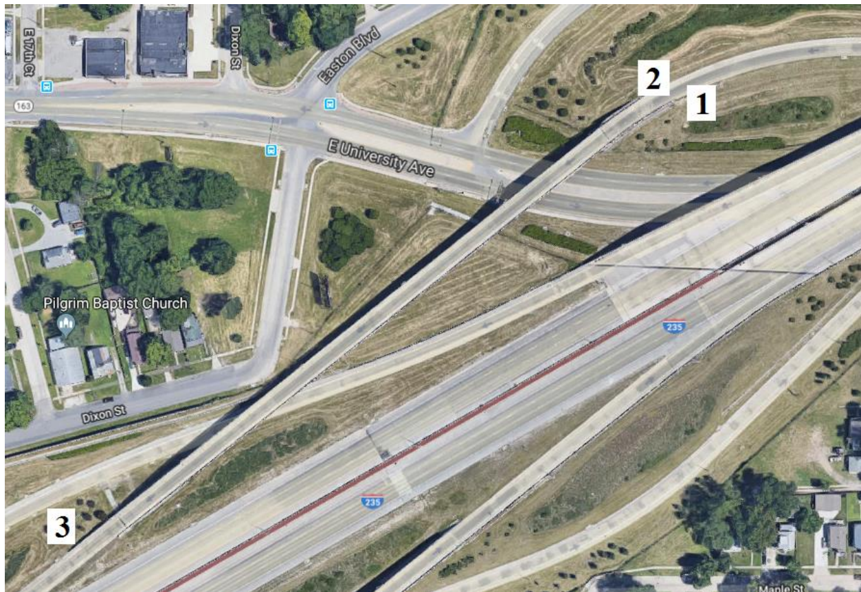
Figure B-135. Bridge No. 7710.0A235 [1]
