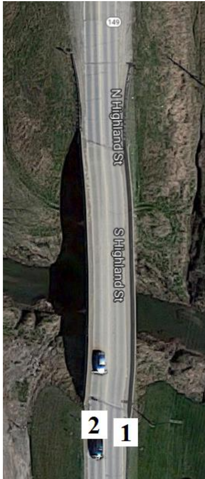
Figure B-71. Bridge No. 4864.8S149 [1]
