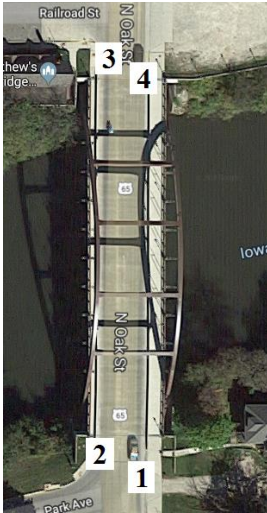
Figure B-67. Bridge No. 4249.6S065 [1]
