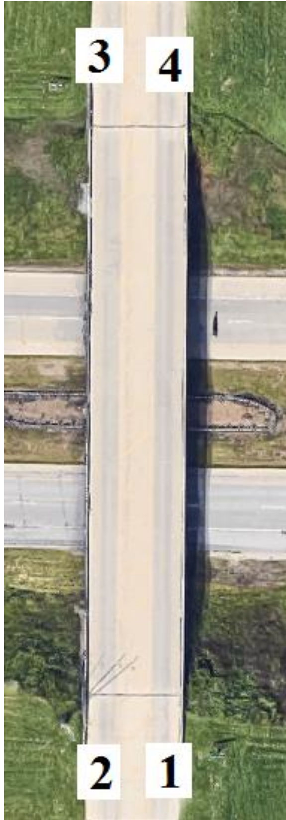
Figure B-7. Bridge No. 0729.00020 [1]
