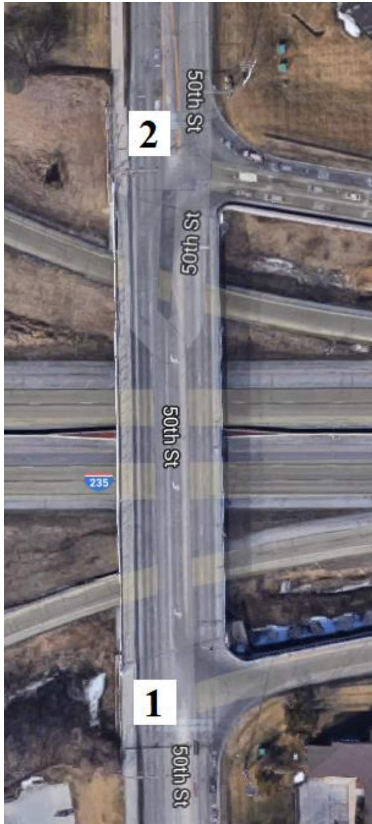
Figure B-114. Bridge No. 7700.3O235 [1]
