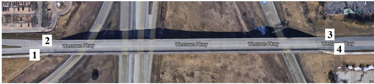
Figure B-139. Bridge No. 7723.8O080 [1]
