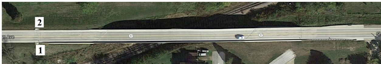
Figure B-65. Bridge No. 4208.0S057 [1]
