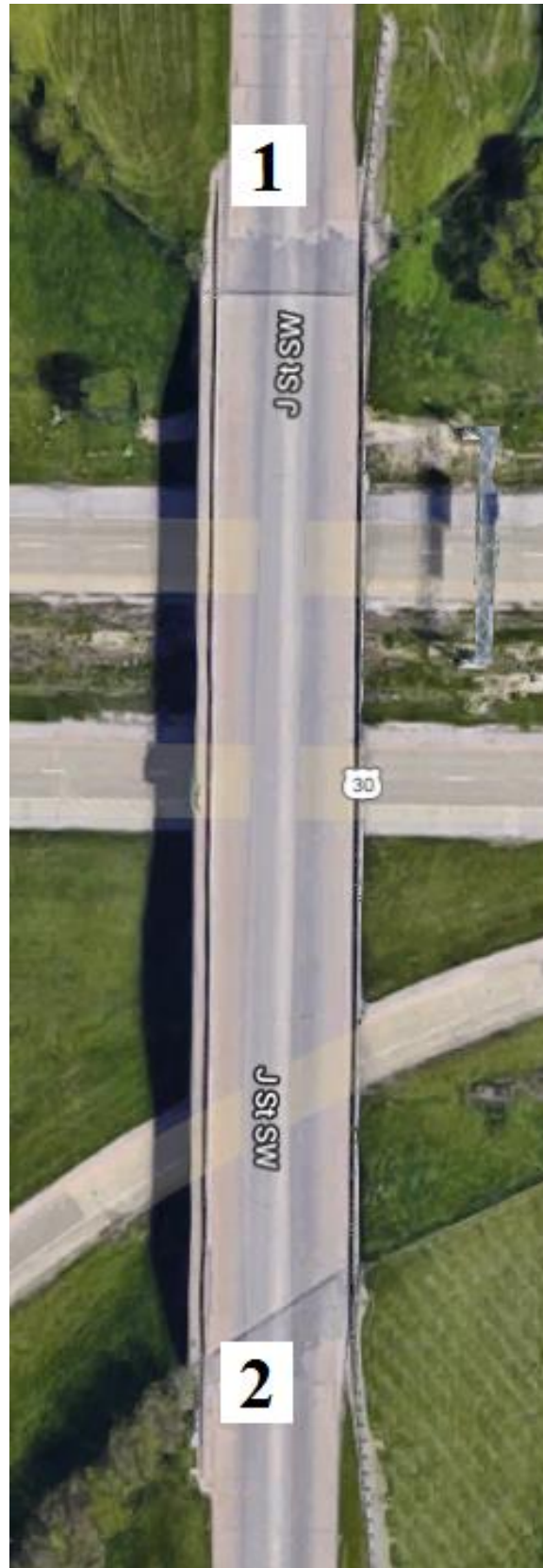
Figure B-99. Bridge No. 5752.9O030 [1]
