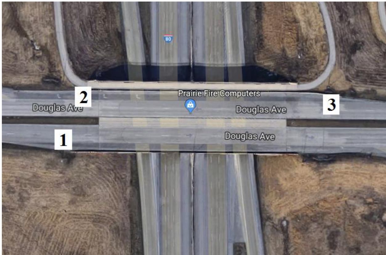
Figure B-141. Bridge No. 7726.1O080 [1]
