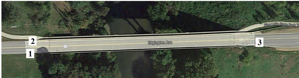
Figure B-68. Bridge No. 4287.7S175 [1]
