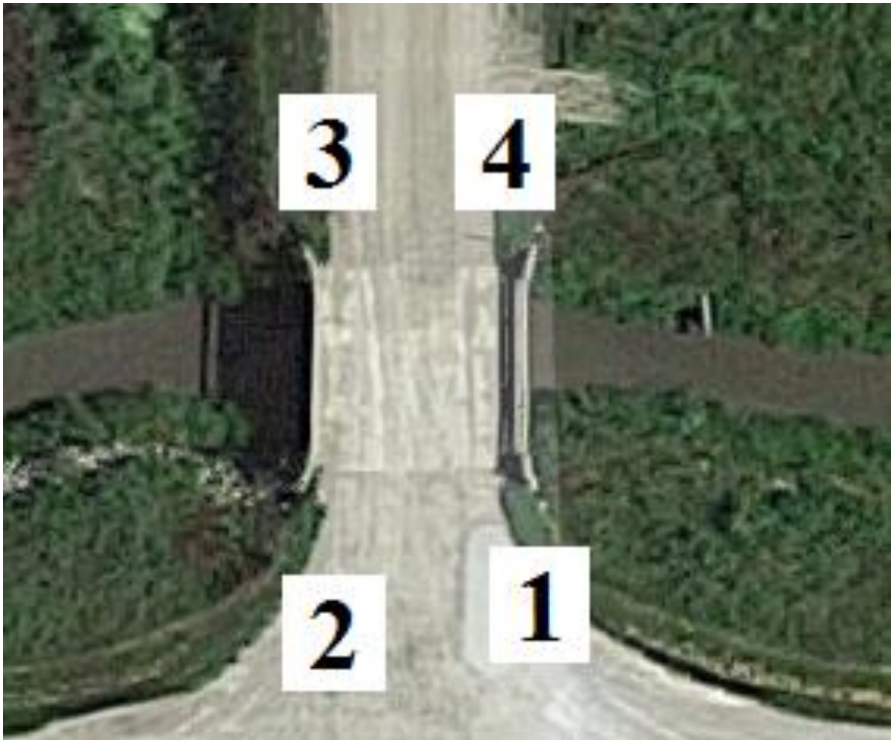
Figure B-110. Bridge No. 7403.2A018 [1]
