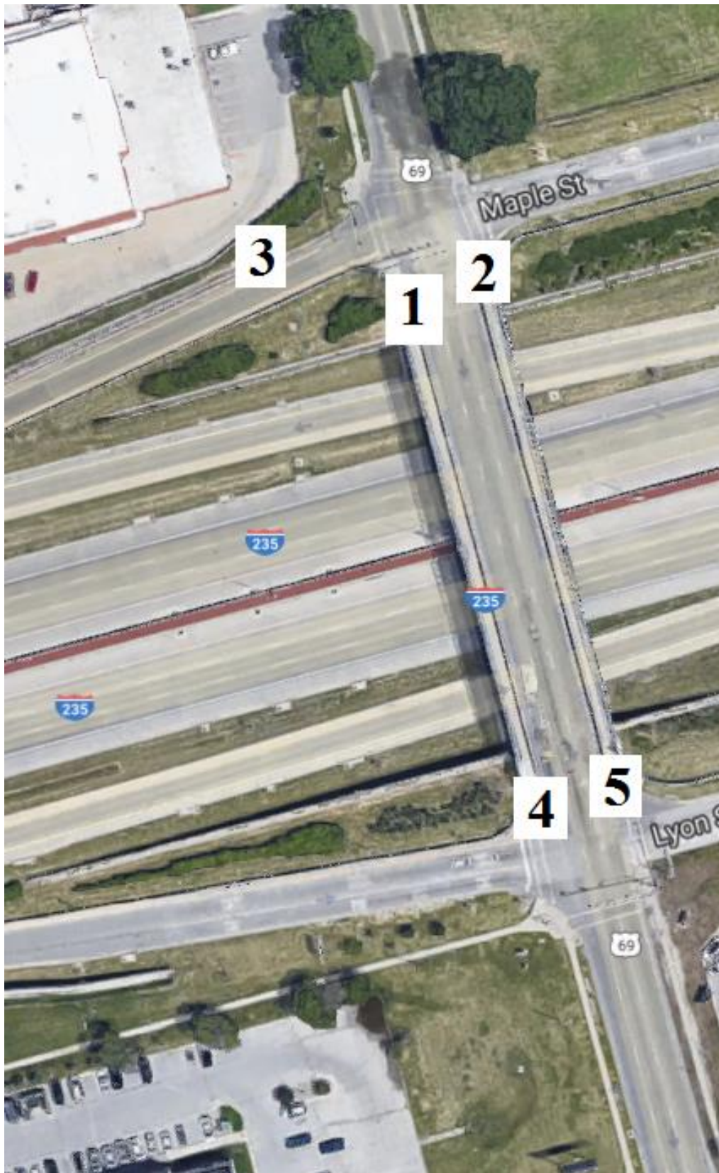
Figure B-147. Bridge No. 7785.5S069 [1]
