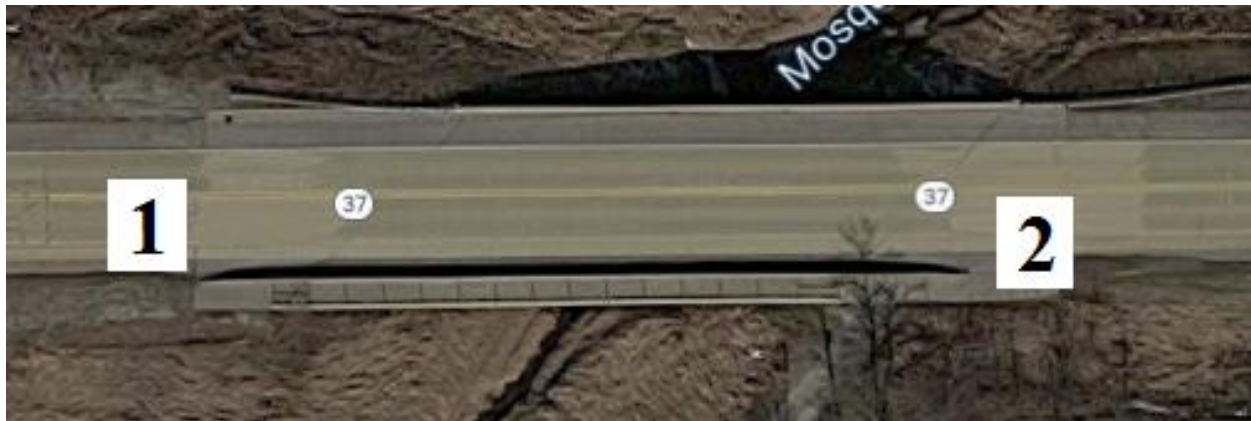
Figure 70. Bridge No. 8336.8S037 [1]
