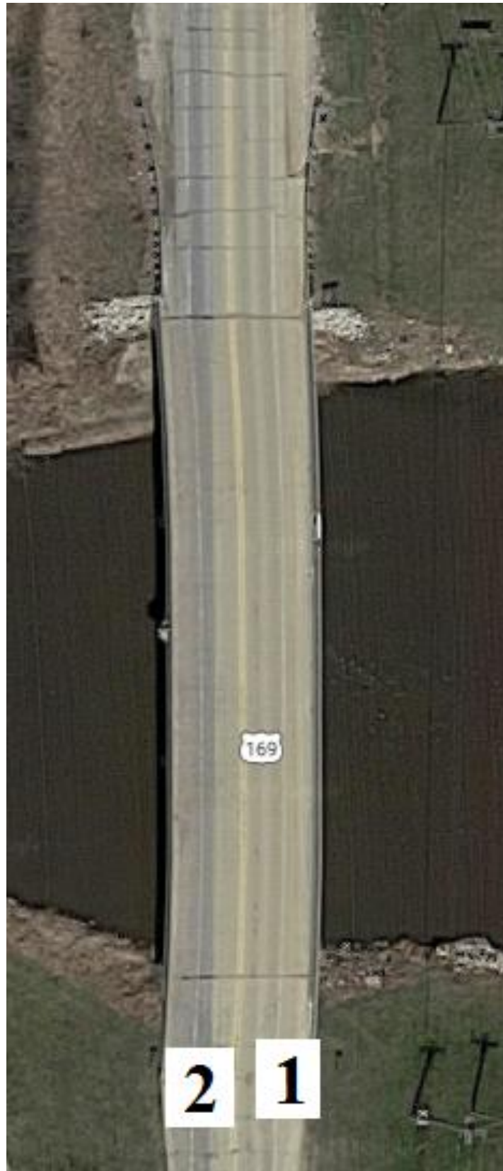
Figure B-33. Bridge No. 2589.1S169 [1]
