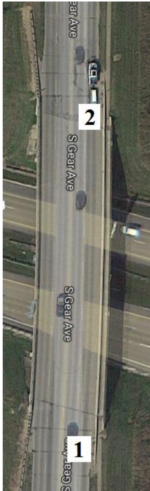
Figure B-40. Bridge No. 2959.6O034 [1]
