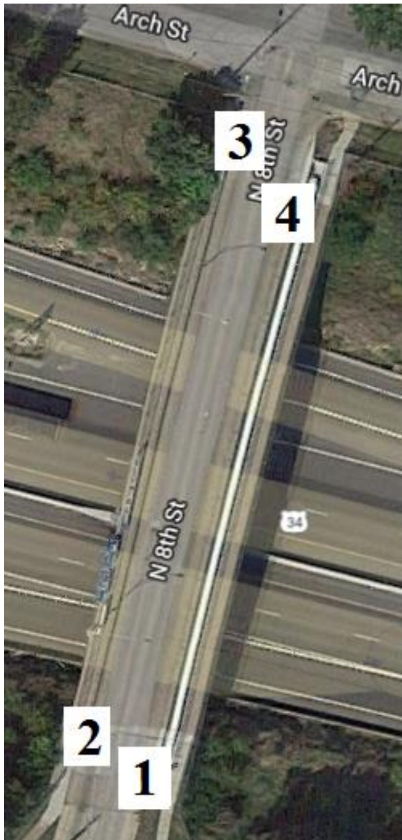
Figure B-43. Bridge No. 2963.00034 [1]
