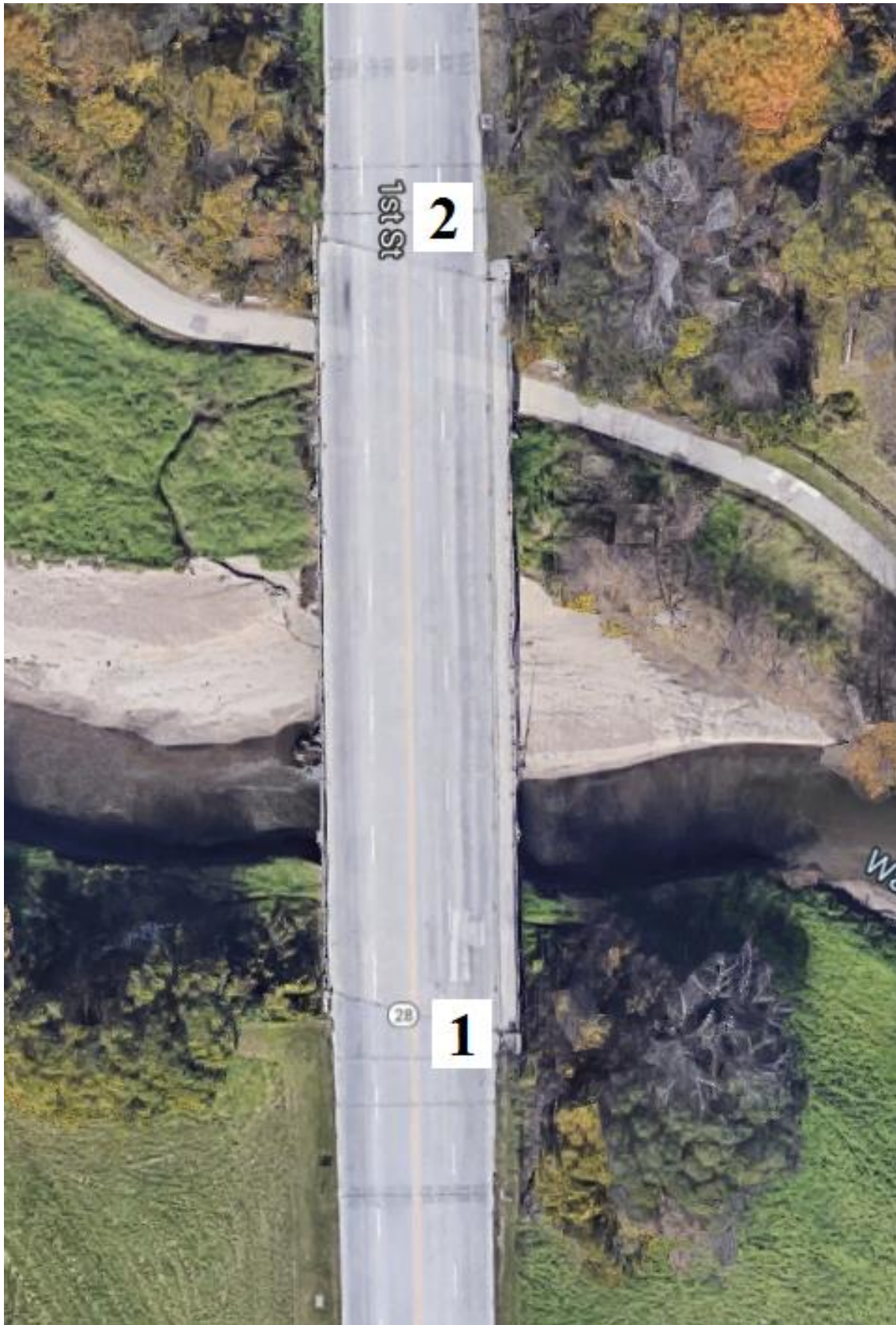
Figure B-136. Bridge No. 7717.8S028 [1]
