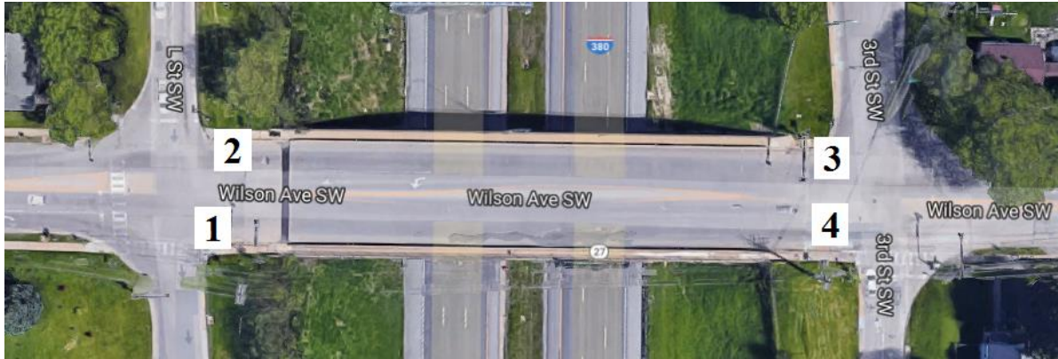
Figure B-91. Bridge No. 5718.40380 [1]
