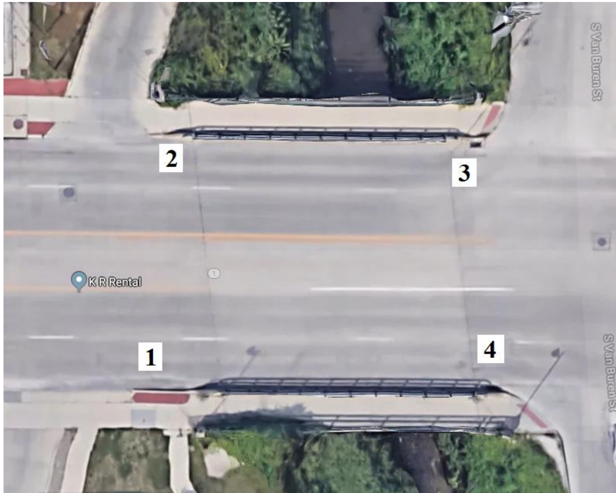
Figure B-82. Bridge No. 5286.5S001 [1]
