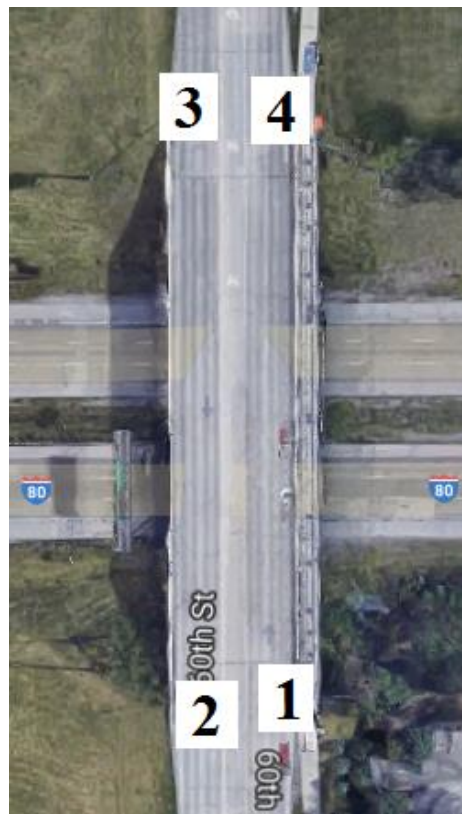
Figure B-138. Bridge No. 7722.4O080 [1]
