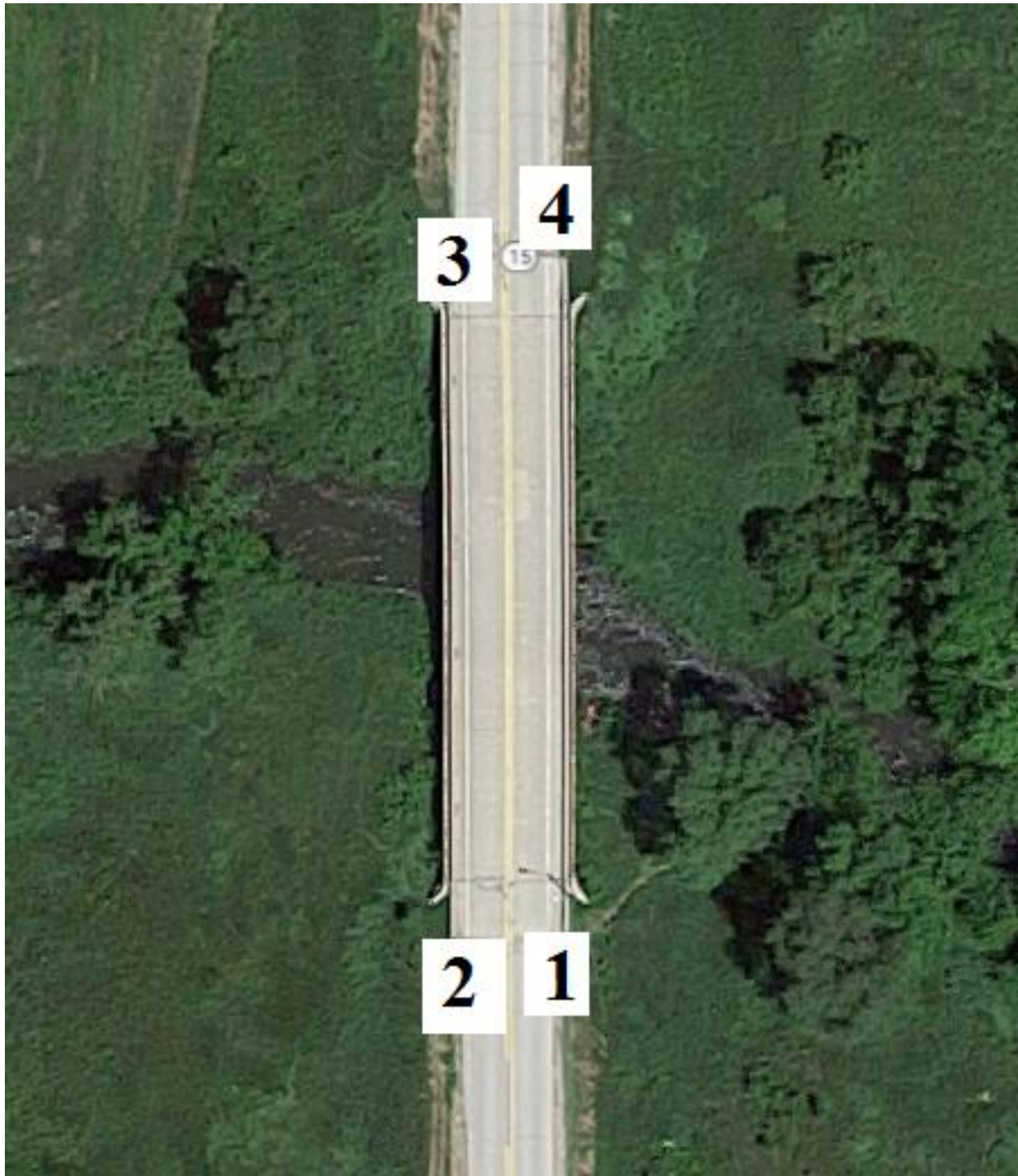
Figure B-112. Bridge No. 7606.6S015 [1]
