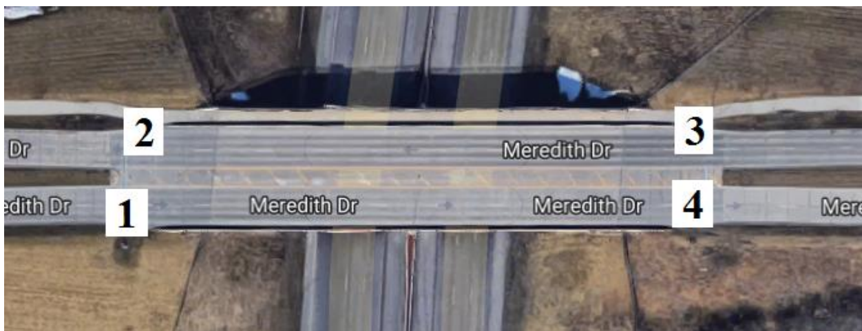
Figure B-142. Bridge No. 7727.1O080 [1]
