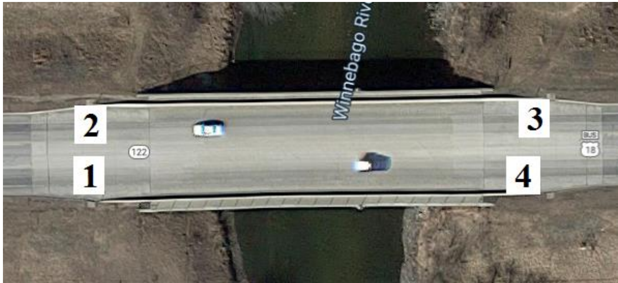
Figure B-23. Bridge No. 1710.2S122 [1]
