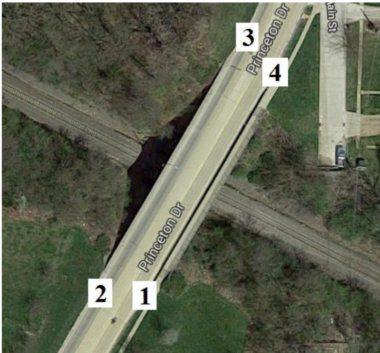
Figure B-108. Bridge No. 6834.5S005 [1]
