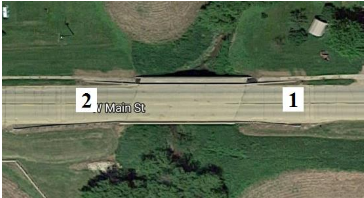
Figure B-72. Bridge No. 4922.0S064 [1]
