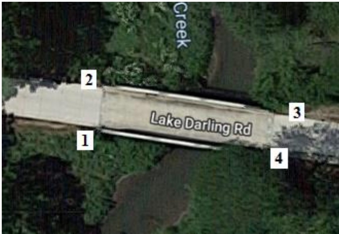
Figure B-171. Bridge No. 9200.4S612 [1]
