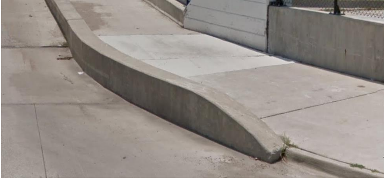
Figure 155. Special Case Sloped End Treatment [1]
