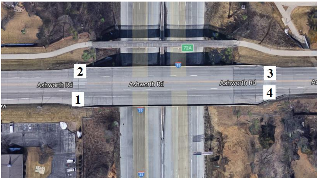
Figure B-146. Bridge No. 7772.2O035 [1]
