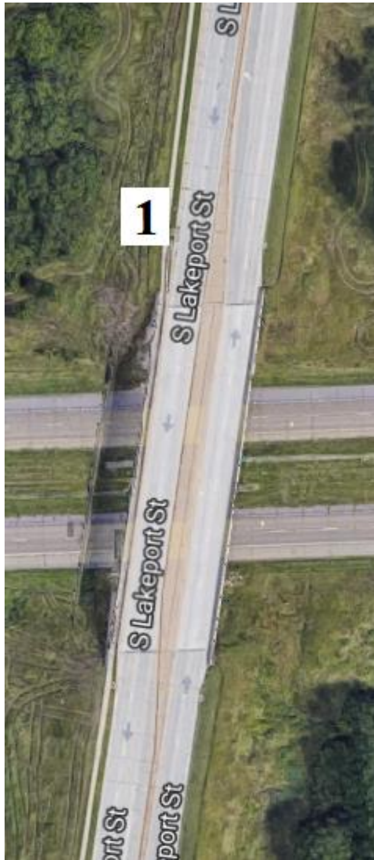
Figure B-179. Bridge No. 9701.8O020 [1]
