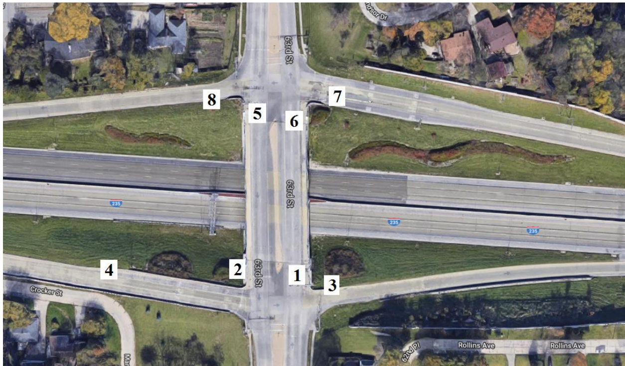
Figure B-137. Bridge No. 7718.3S028 [1]
