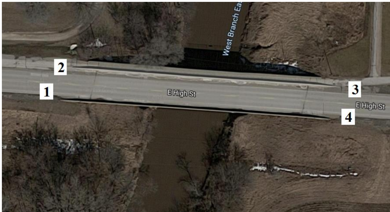
Figure B-149. Bridge No. 7815.0S083 [1]
