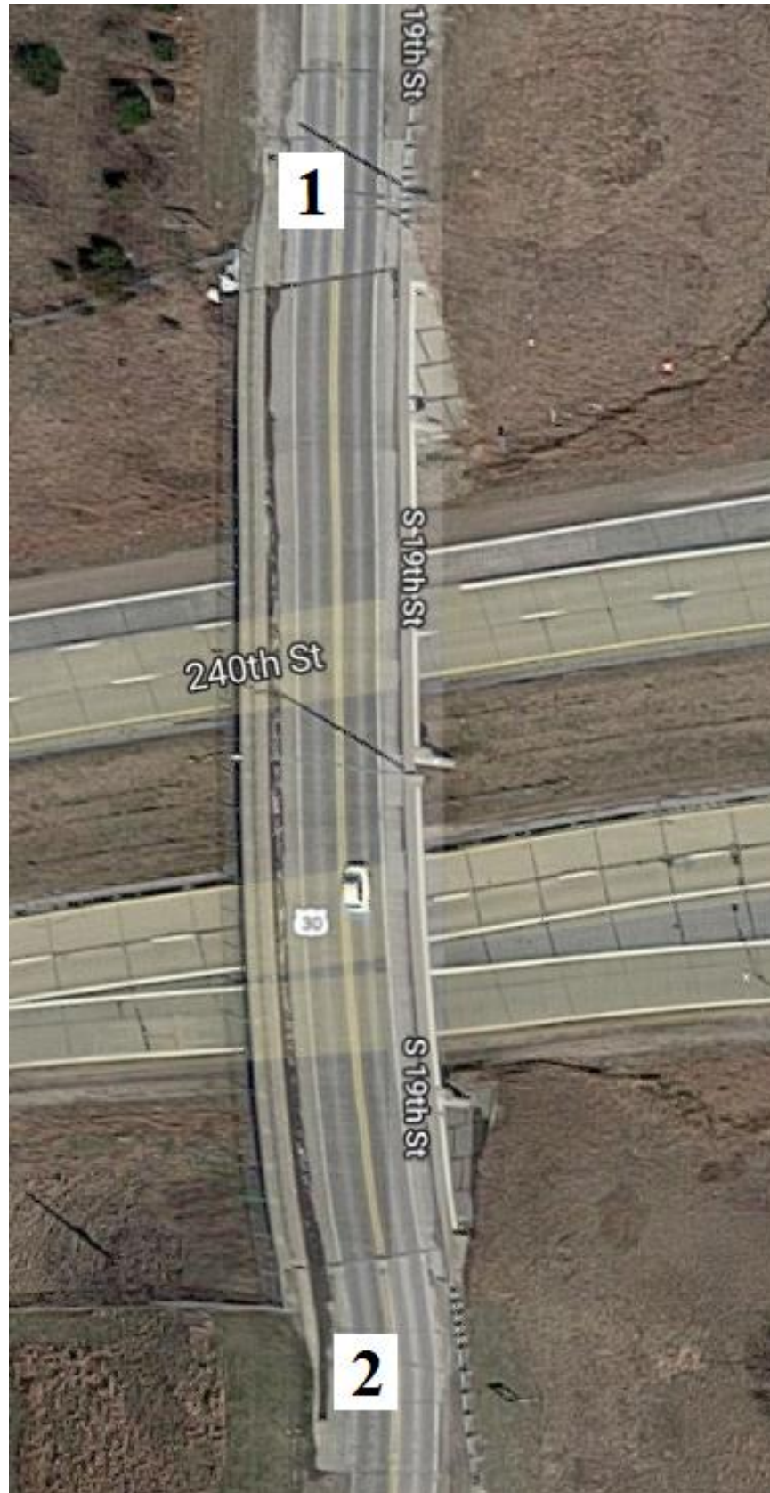
Figure B-163. Bridge No. 8558.4O030 [1]
