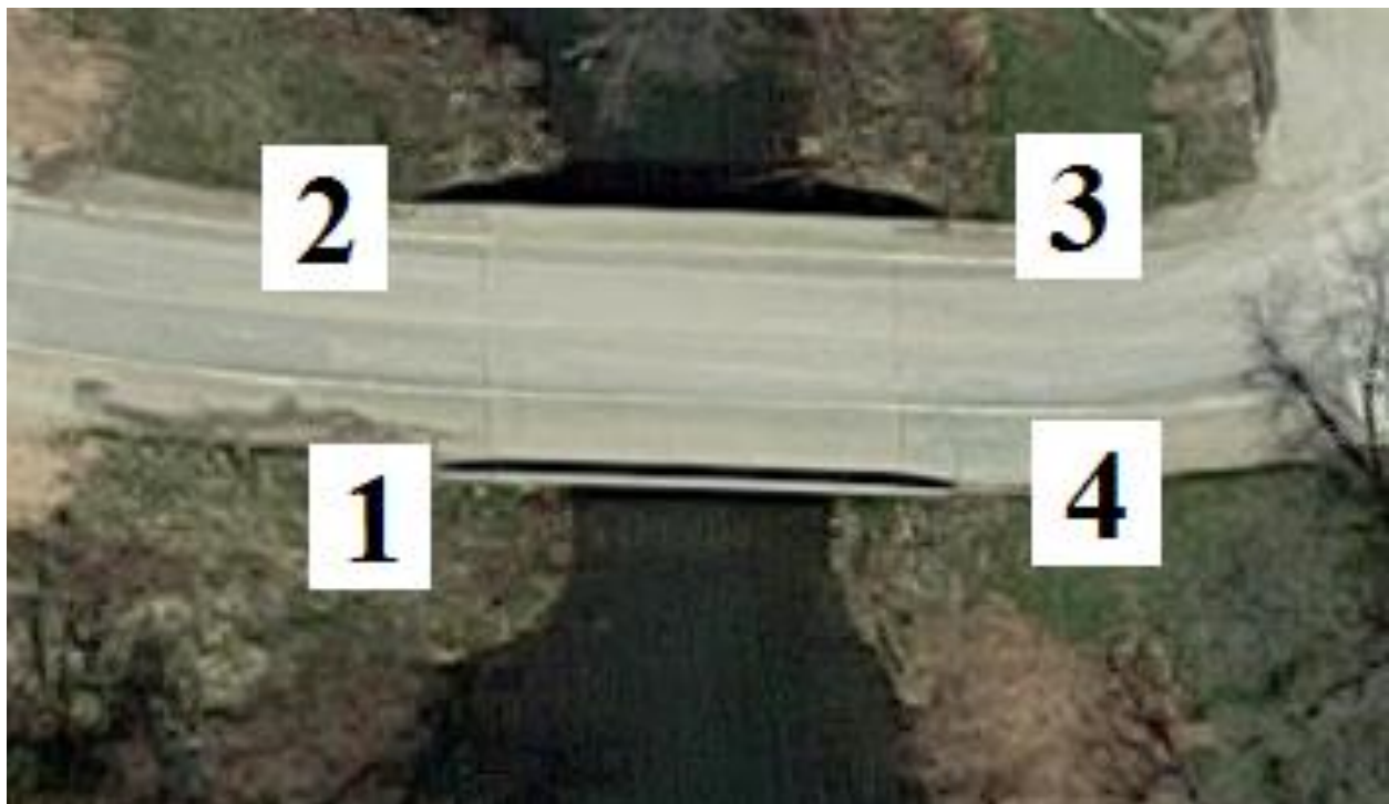
Figure B-104. Bridge No. 6200.9S622 [1]
