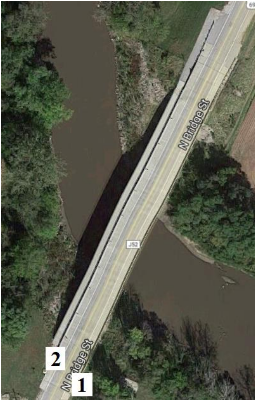
Figure B-34. Bridge No. 2711.3S069 [1]
