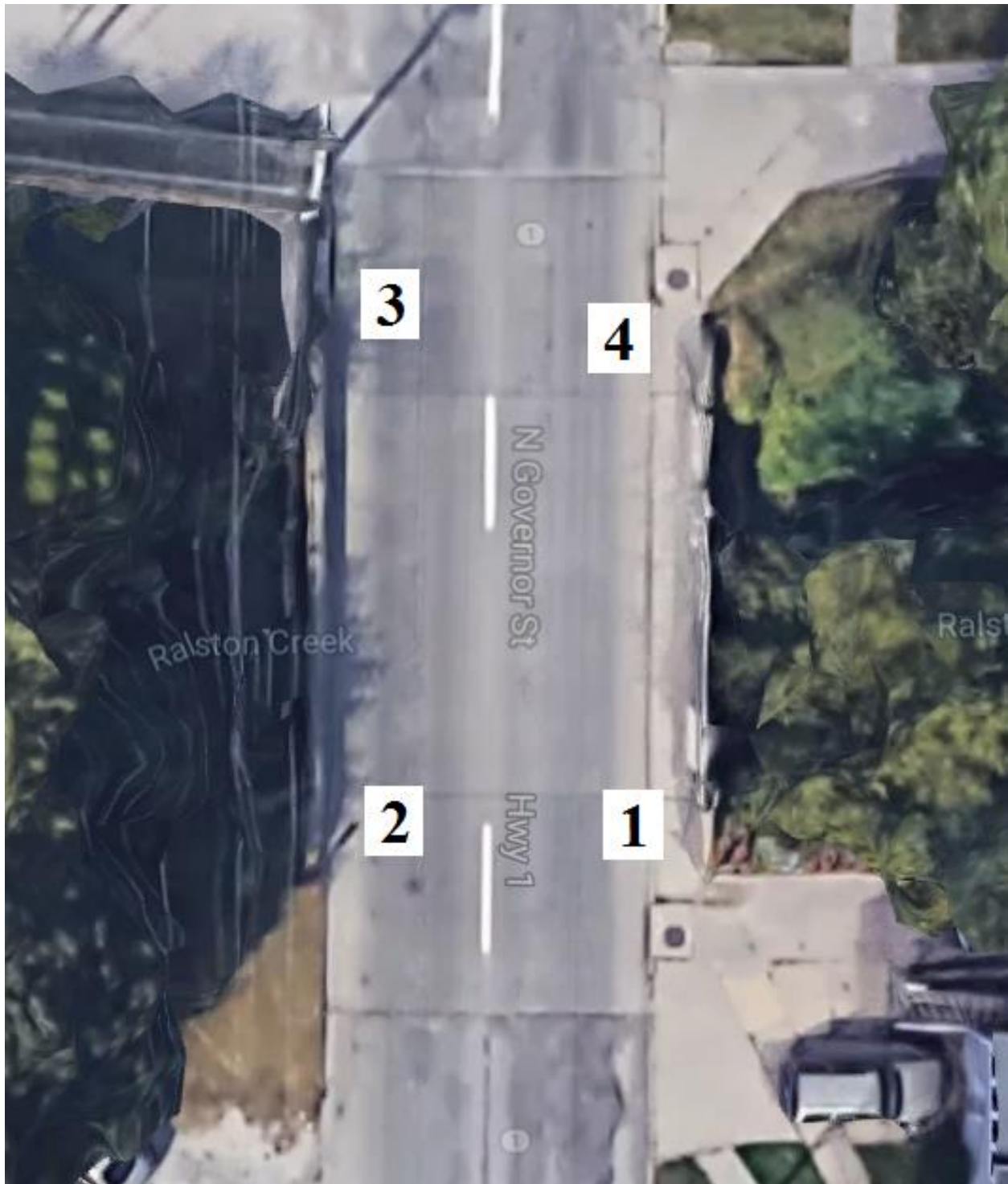
Figure B-84. Bridge No. 5287.2R001 [1]
