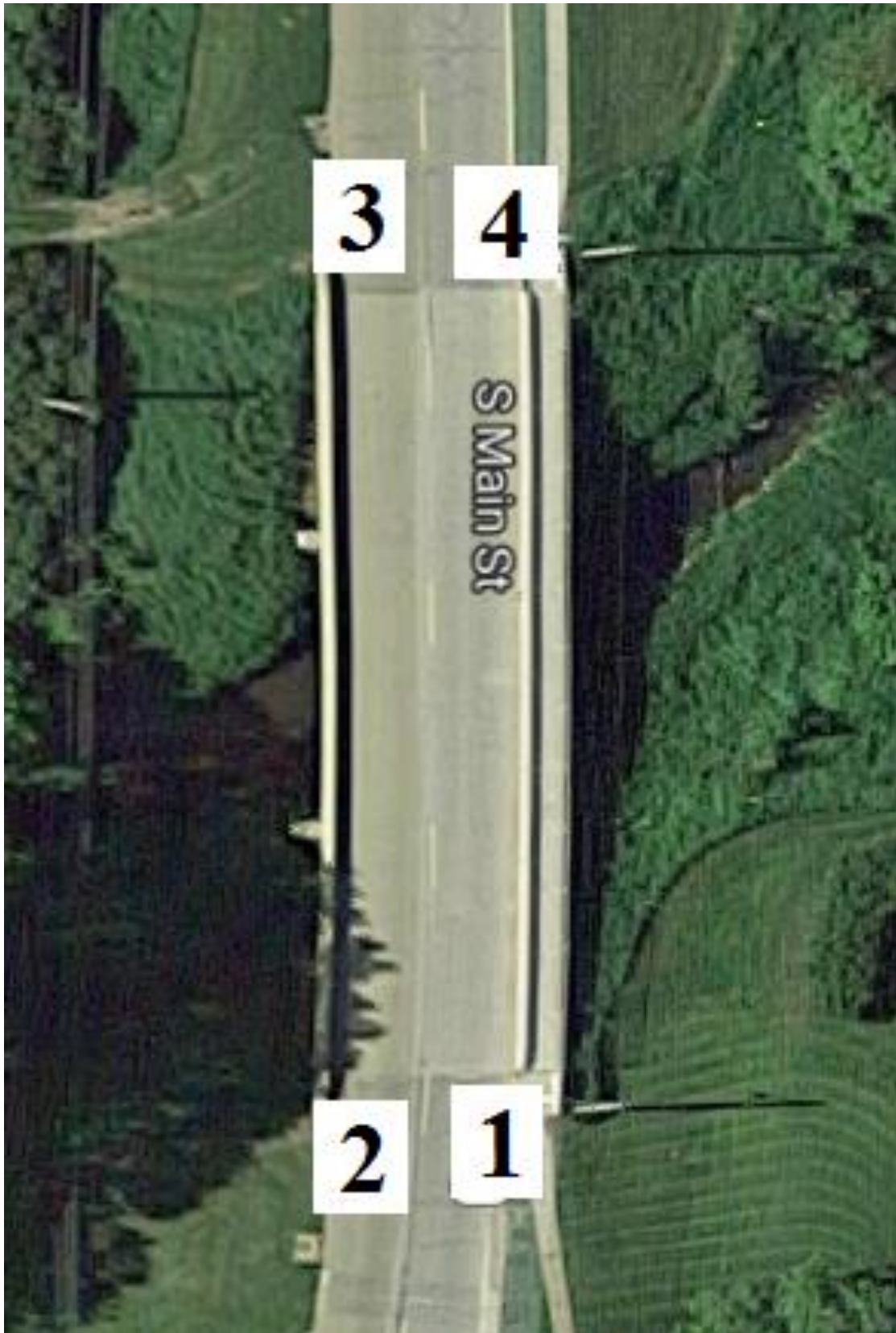
Figure B-111. Bridge No. 7509.3S140 [1]
