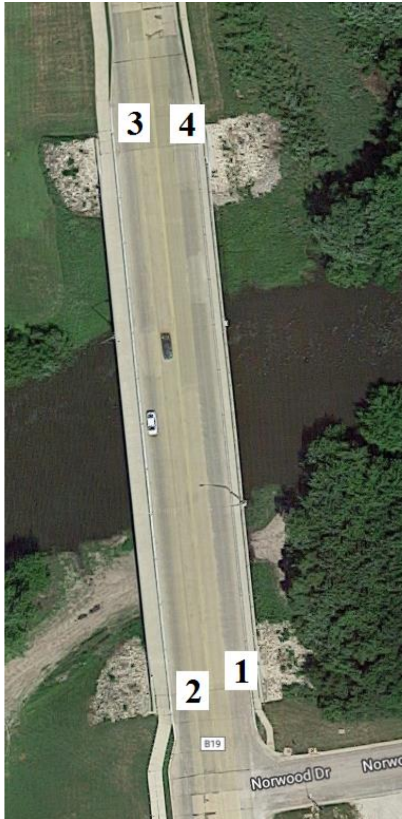
Figure B-88. Bridge No. 5598.7S169 [1]
