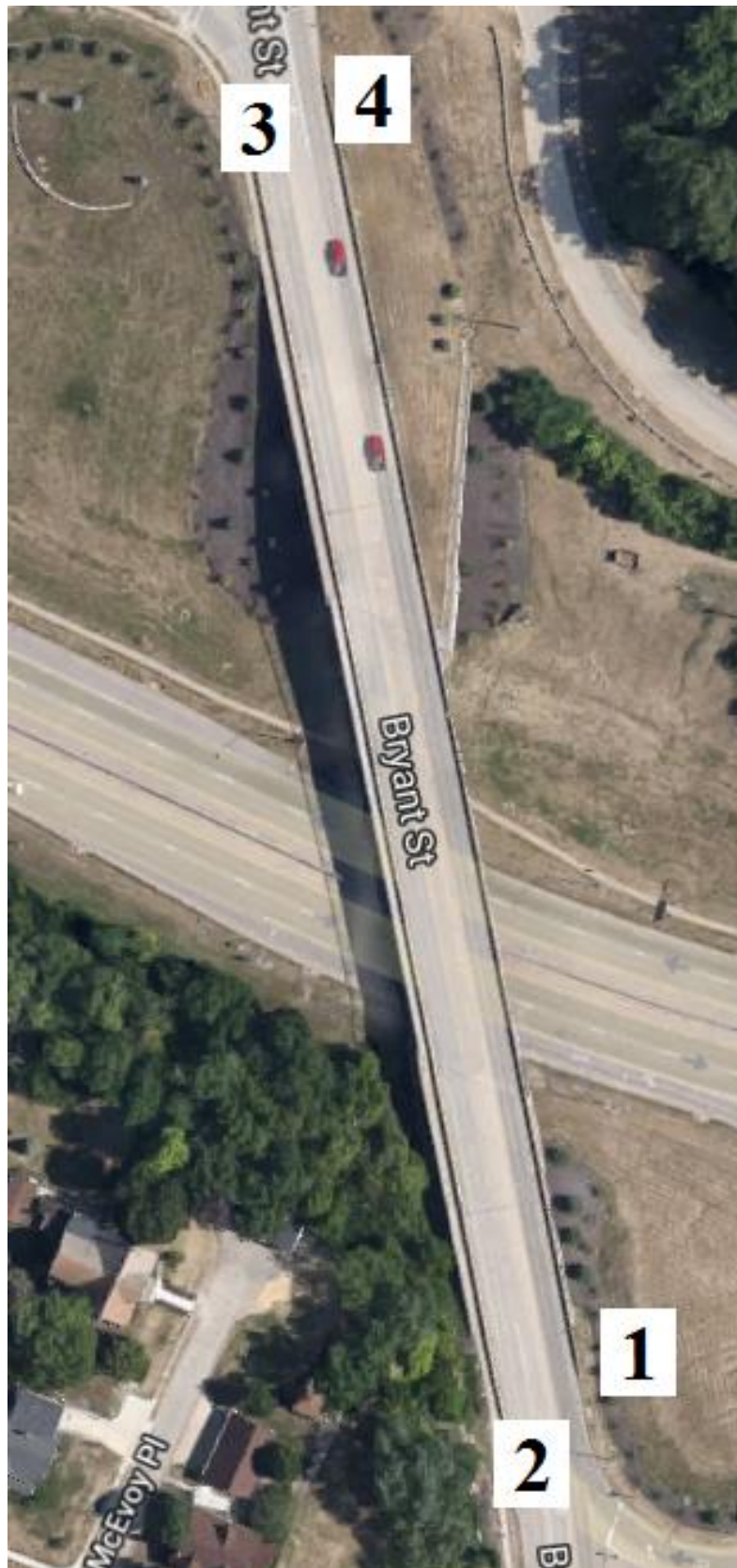
Figure B-51. Bridge No. 3119.00020 [1]
