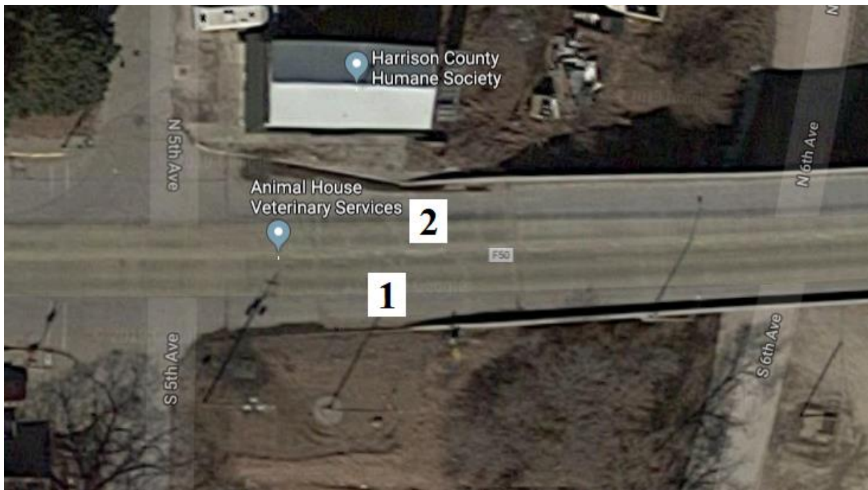
Figure B-69. Bridge No. 4319.5S030 [1]
