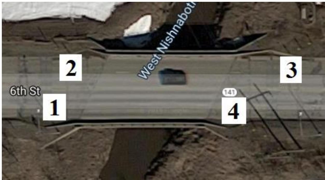
Figure B-19. Bridge No. 1477.0S141 [1]
