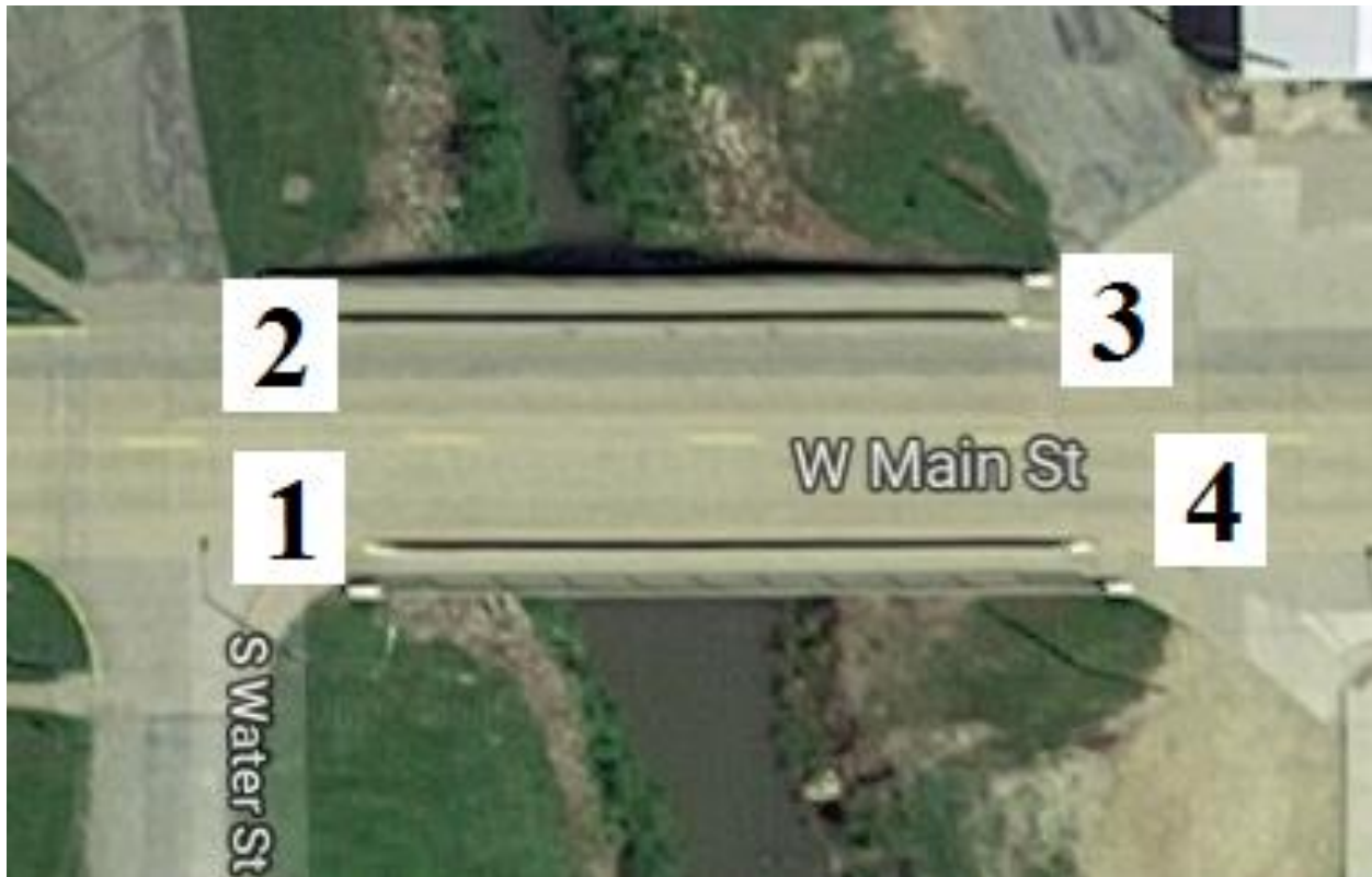
Figure B-85. Bridge No. 5314.8S064 [1]
