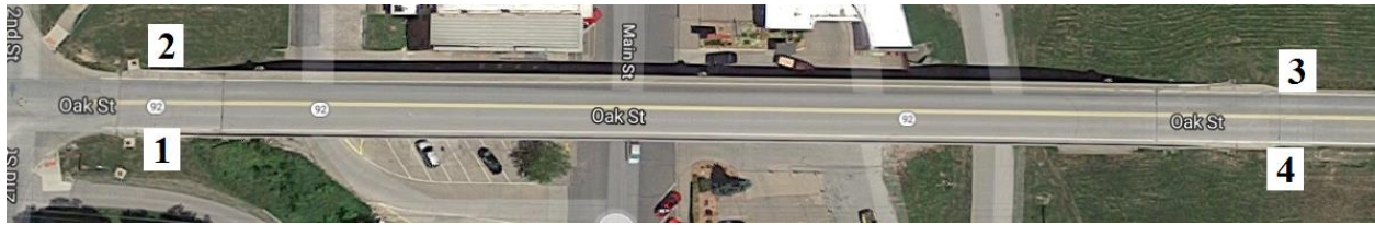
Figure B-101. Bridge No. 5851.3S092 [1]
