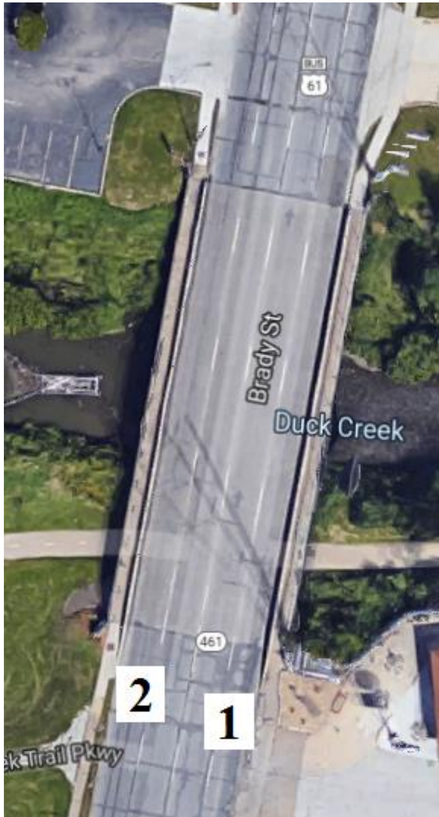
Figure B-156. Bridge No. 8220.1R061 [1]
