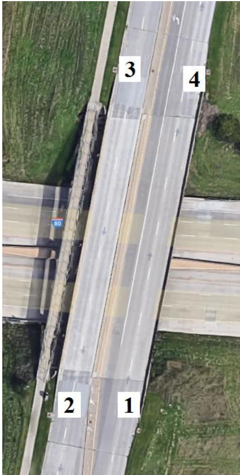
Figure B-77. Bridge No. 5243.00080 [1]
