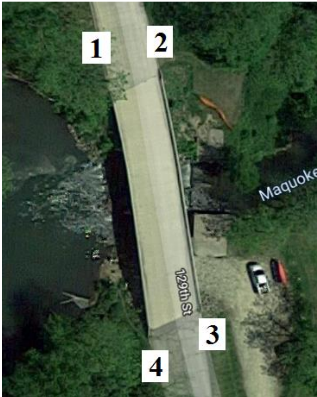
Figure B-37. Bridge No. 2803.8S603 [1]
