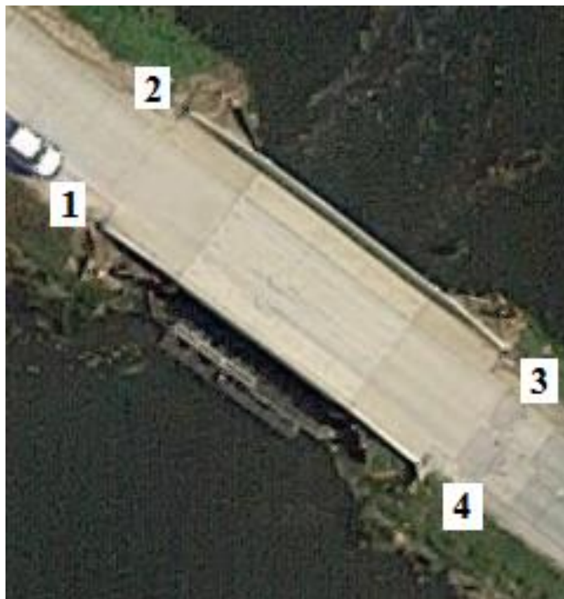
Figure B-150. Bridge No. 8100.3S607 [1]
