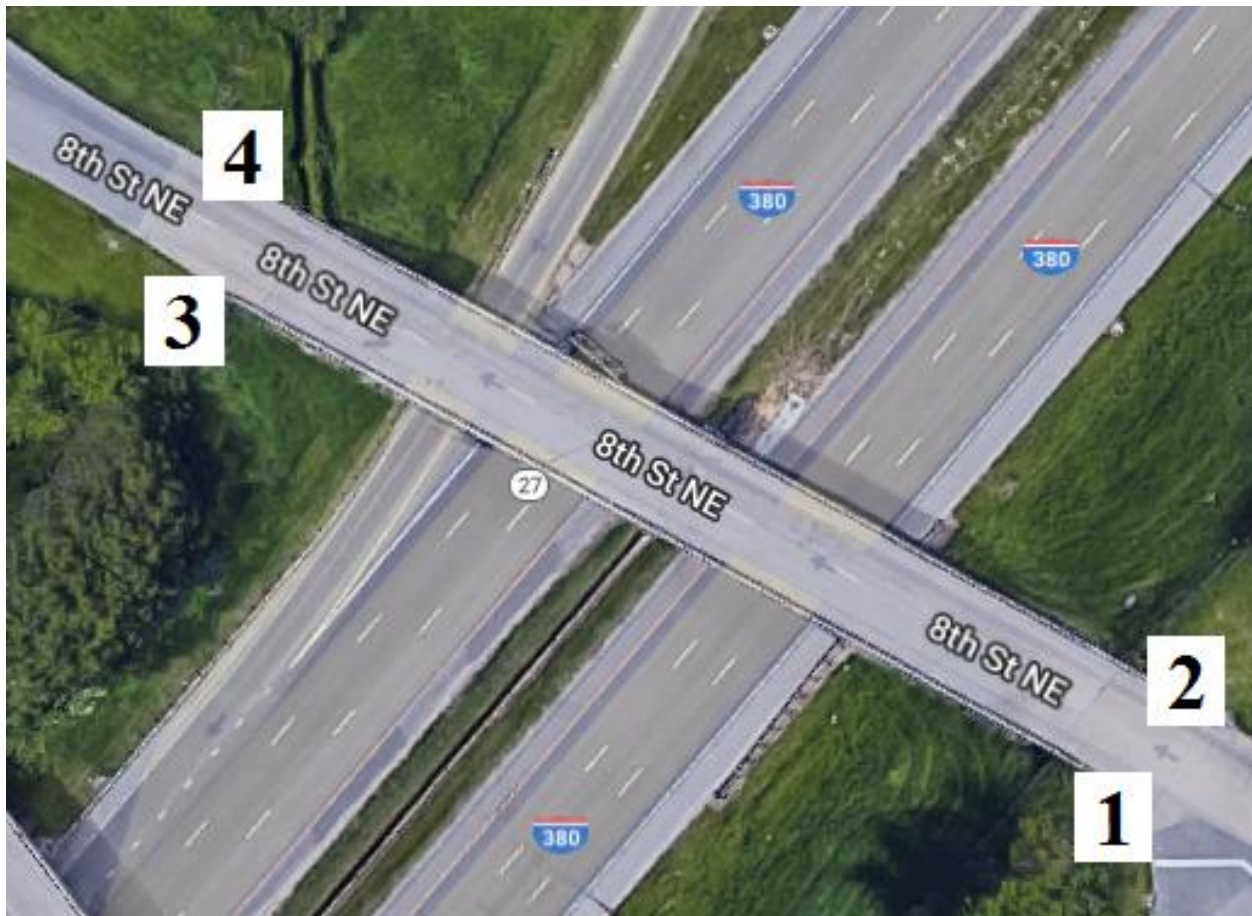
Figure B-93. Bridge No. 5720.8O380 [1]
