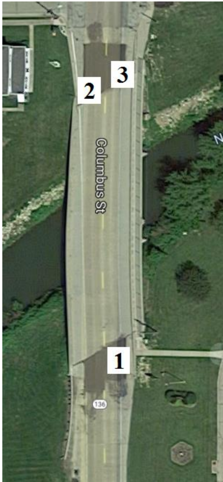
Figure B-56. Bridge No. 3192.7S136 [1]
