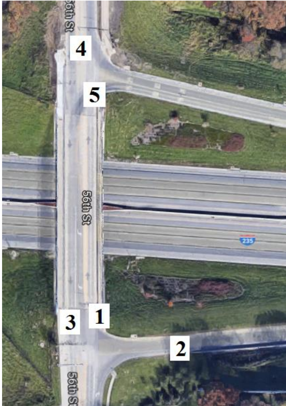
Figure 148. Bridge No. 7704.40235 with Sloped End Treatments Labeled [1]
