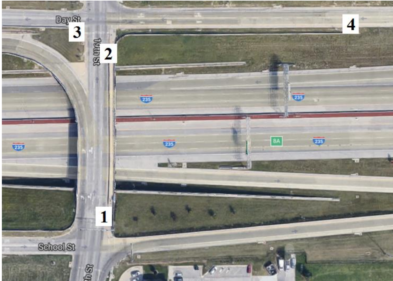
Figure B-125. Bridge No. 7707.20235 [1]
