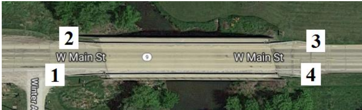
Figure B-107. Bridge No. 6616.8S009 [1]
