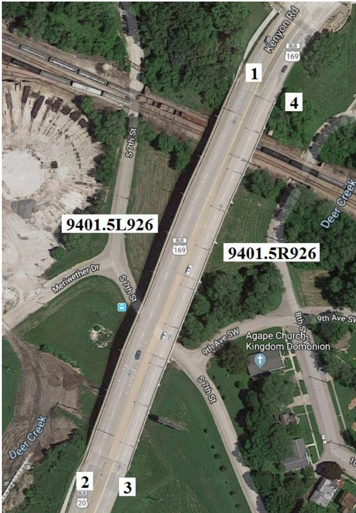
Figure B-174. Bridge Nos. 9401.5L926 and 9401.5R926 [1]
