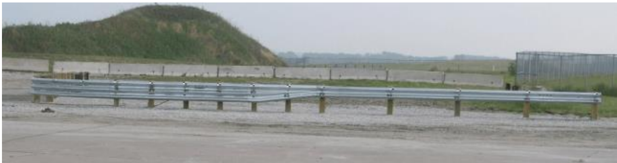
Figure 5. Short Radius Guardrail [26]
