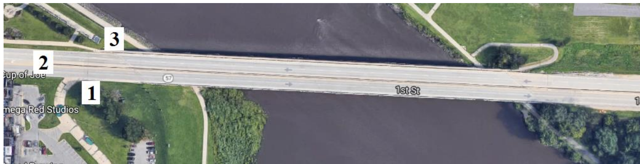
Figure B-10. Bridge No. 0743.1S057 [1]
