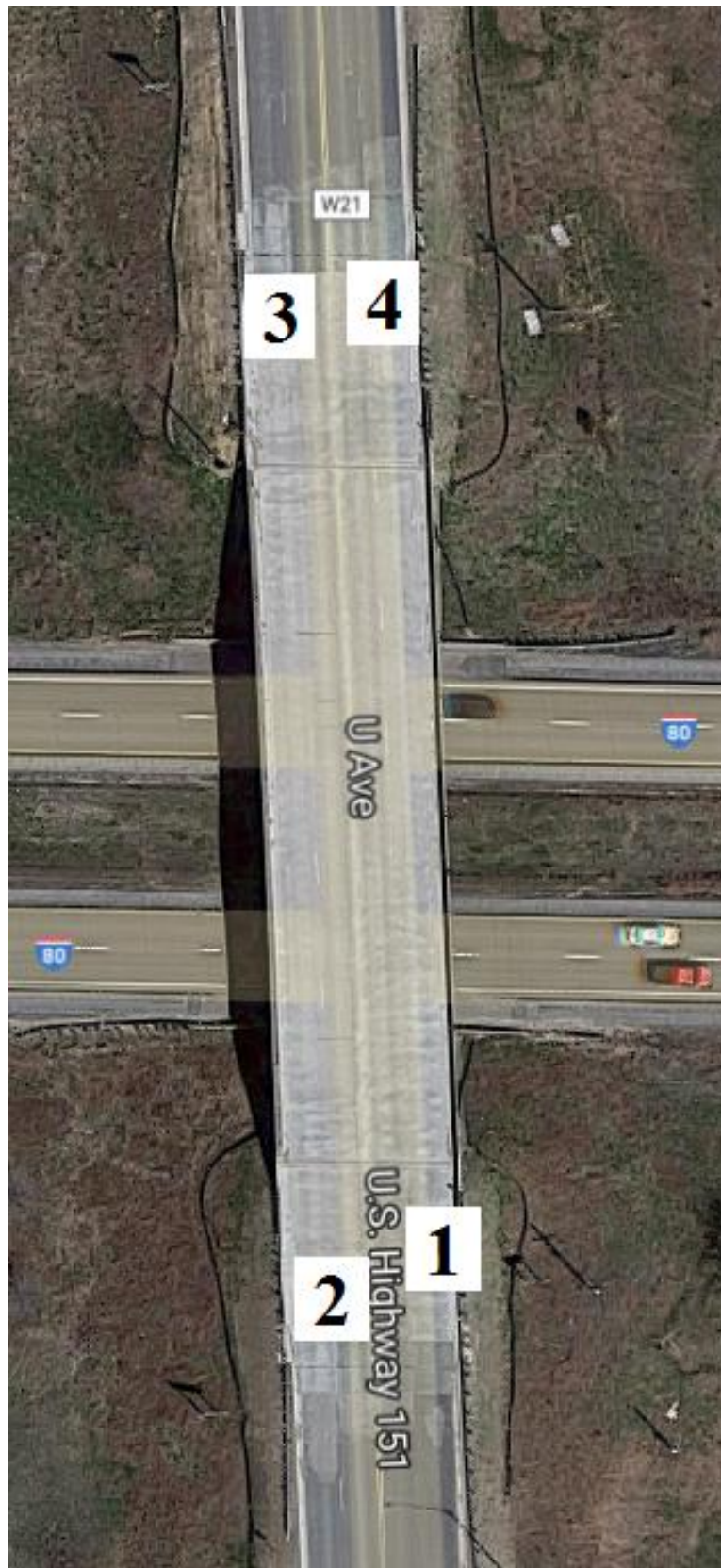
Figure B-70. Bridge No. 4800.2S151 [1]
