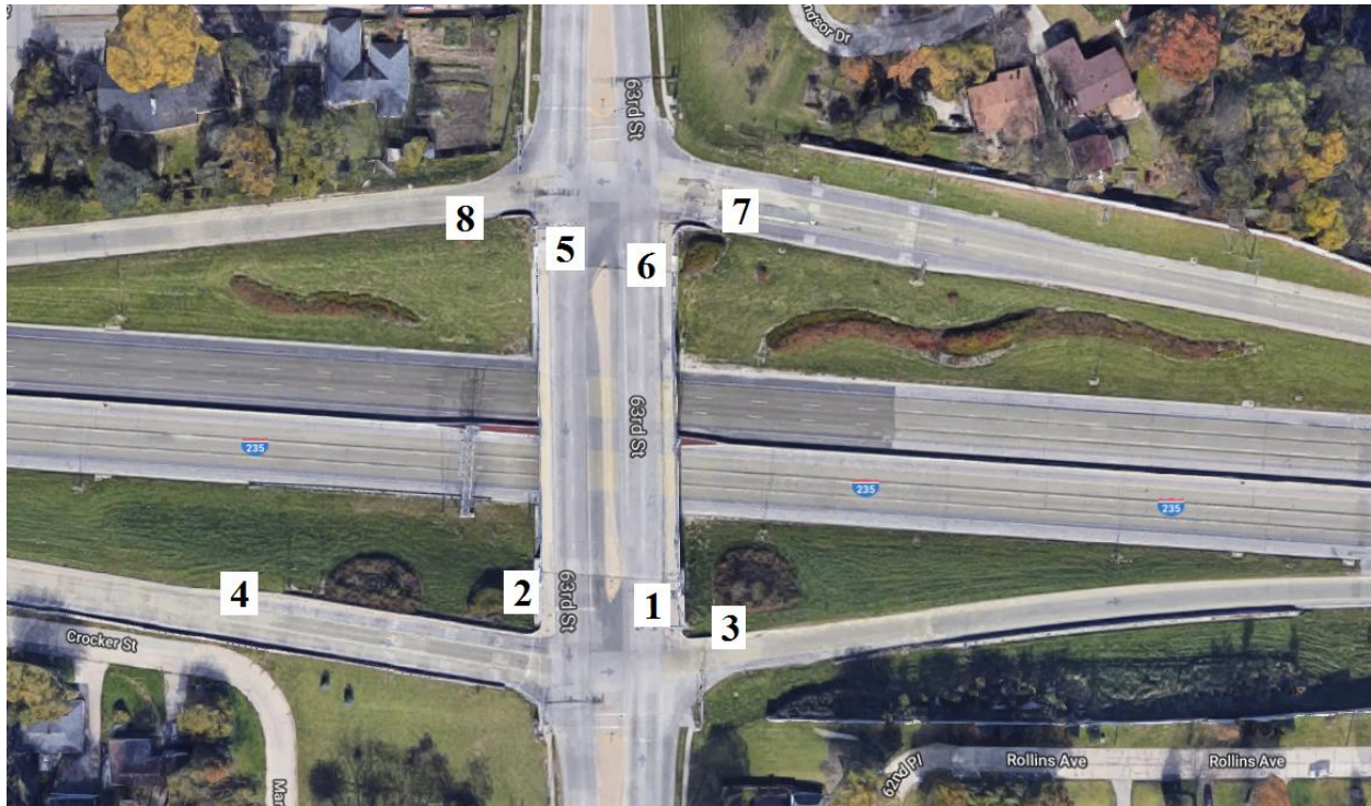
Figure 79. Bridge No. 7718.3S028 [1]
