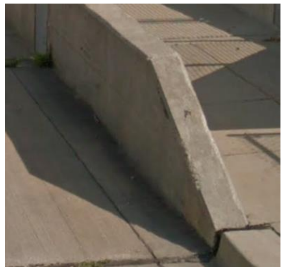
Figure 59. Sloped End Treatment Geometry – (a) Round Tapers and (b) Straight Tapers [1]
