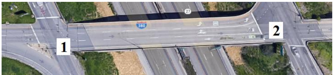
Figure B-95. Bridge No. 5723.8O380 [1]
