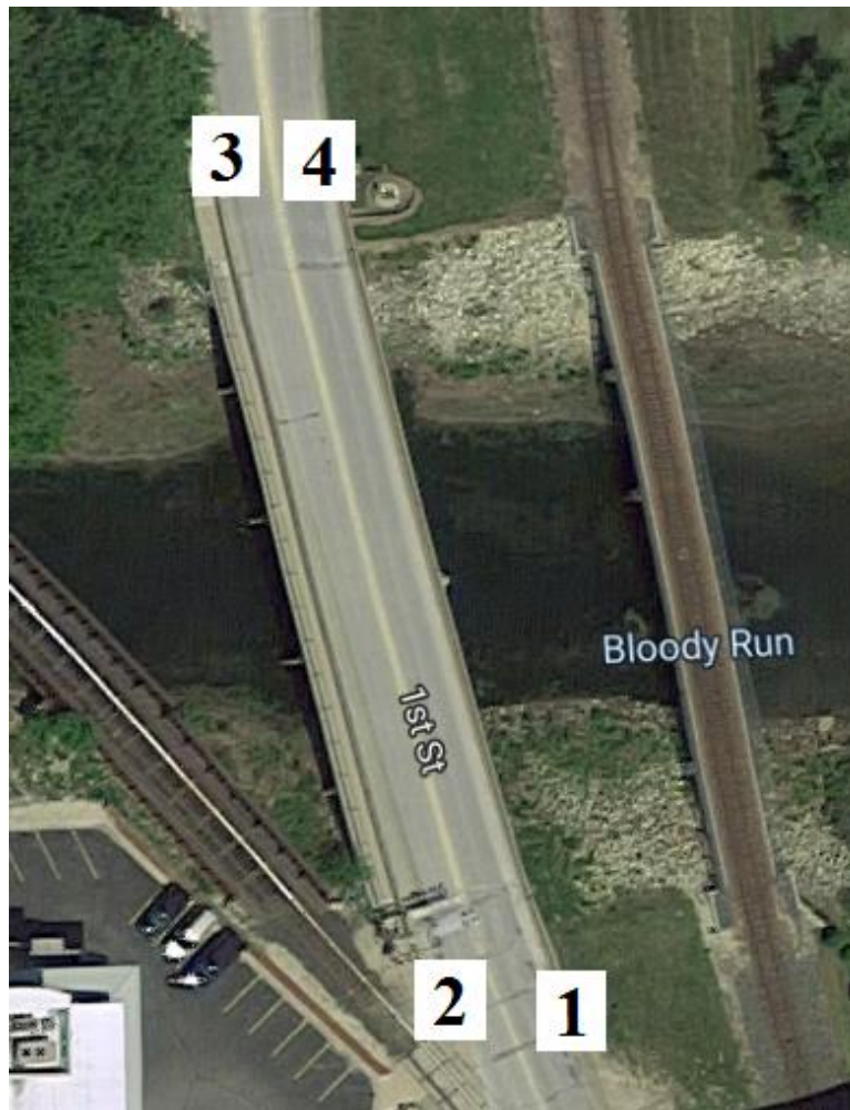
Figure B-29. Bridge No. 2204.5S076 [1]
