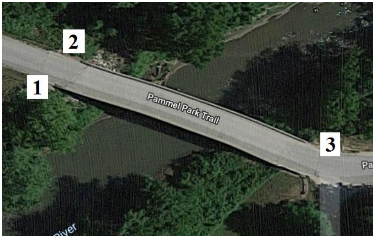
Figure B-103. Bridge No. 6100.1S637 [1]
