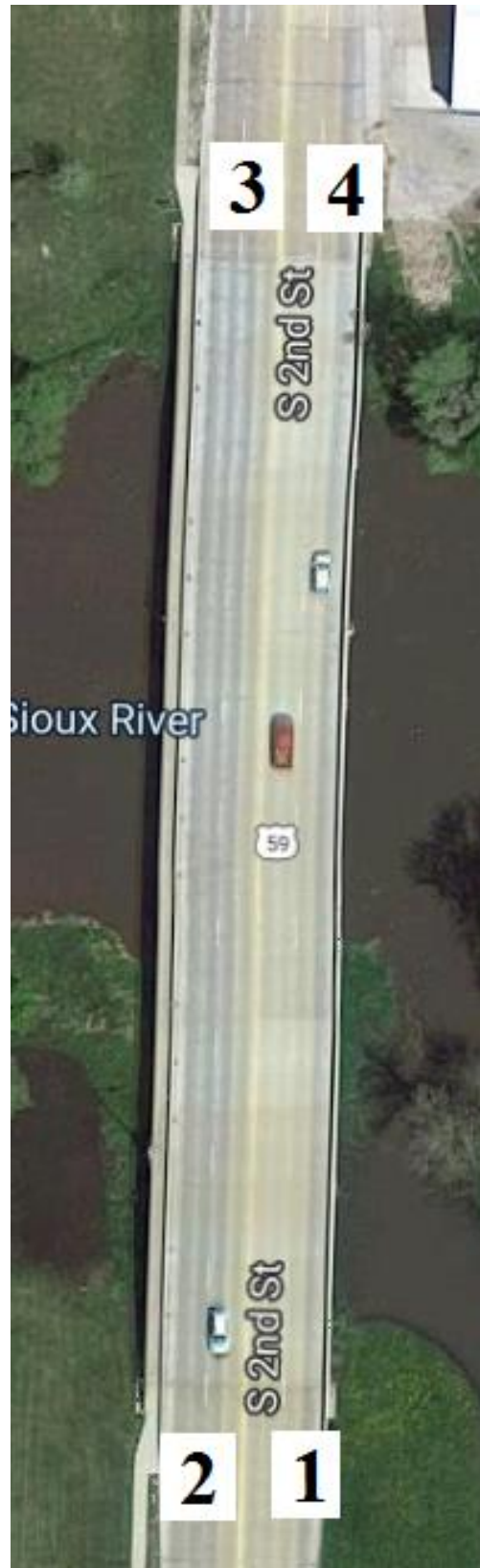
Figure B-26. Bridge No. 1859.0S059 [1]
