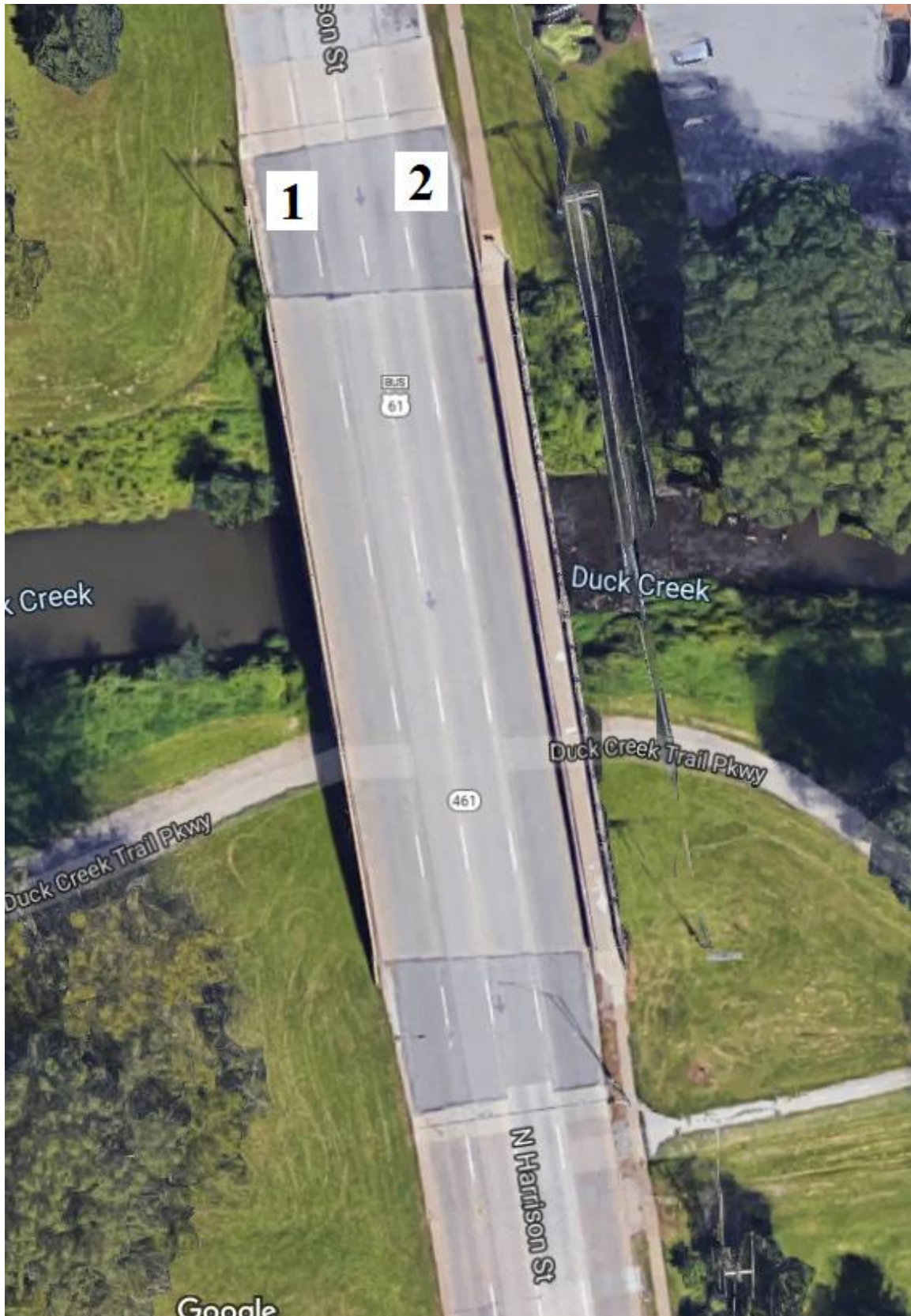
Figure B-155. Bridge No. 8220.1L061 [1]
