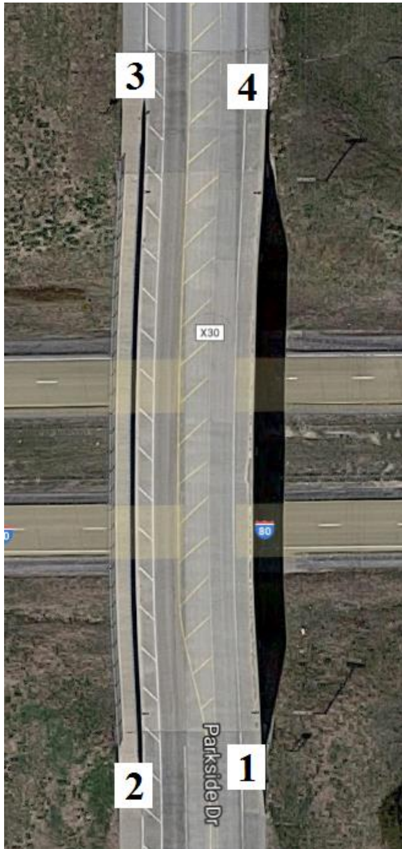
Figure B-22. Bridge No. 1654.6O080 [1]
