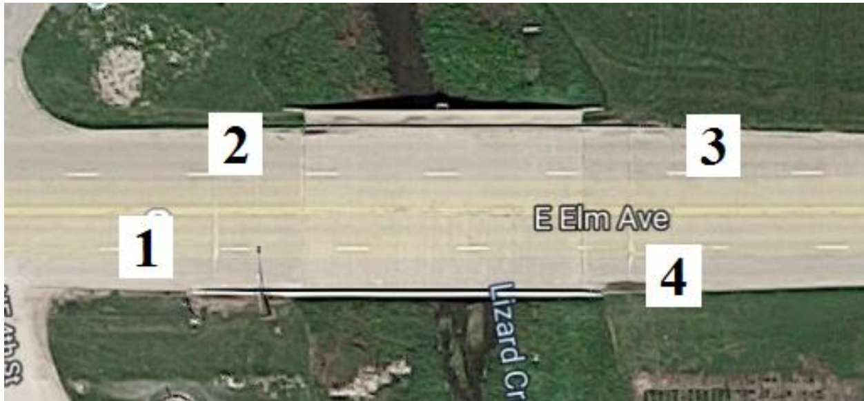
Figure B-113. Bridge No. 7607.2S003 [1]
