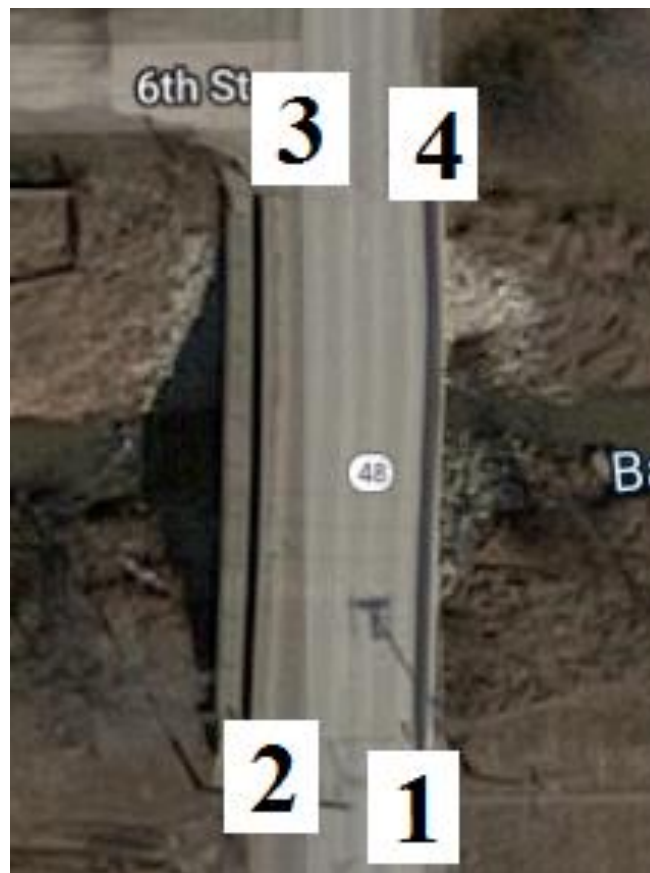
Figure B-20. Bridge No. 1542.6S048 [1]
