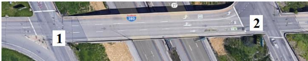
Figure 88. Bridge No. 5723.8O380 [1]
