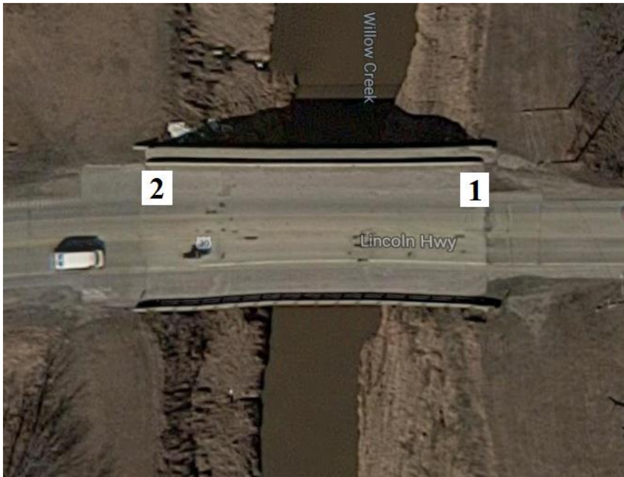
Figure B-66. Bridge No. 4309.8S030 [1]
