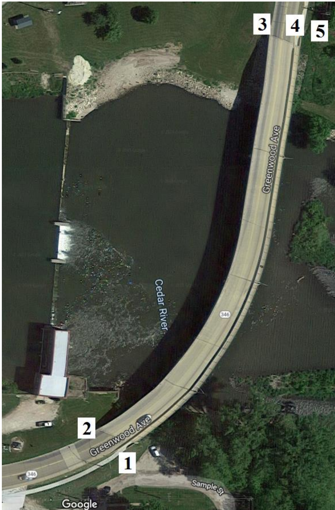
Figure B-27. Bridge No. 1900.5S346 [1]
