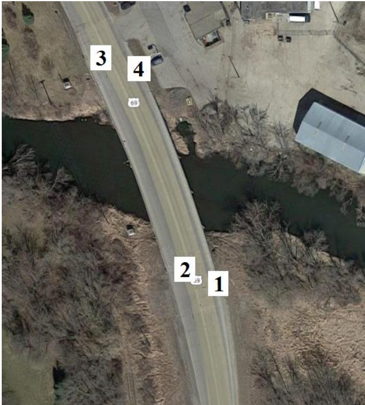
Figure B-175. Bridge No. 9505.0S069 [1]
