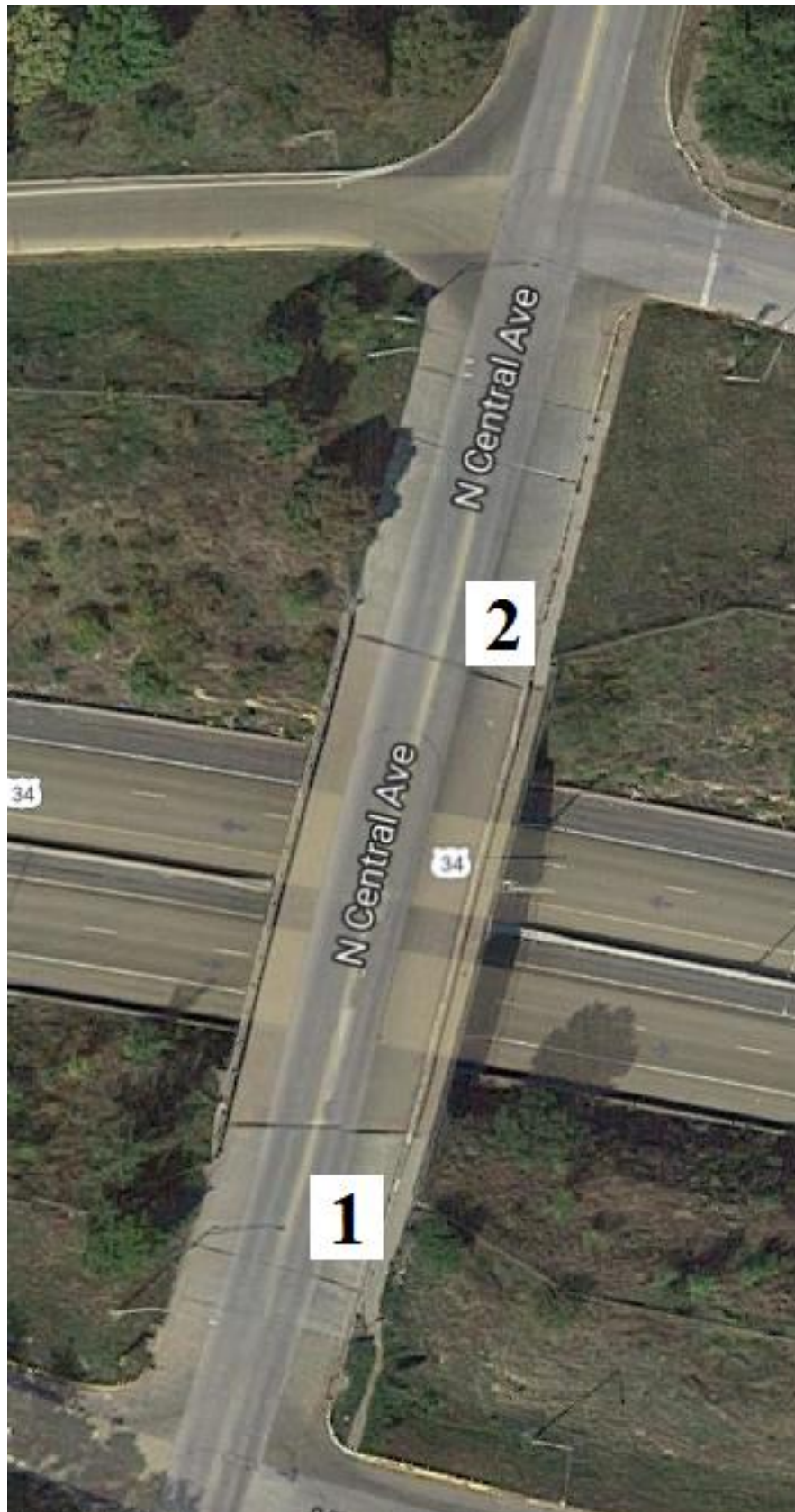
Figure B-42. Bridge No. 2962.9O034 [1]
