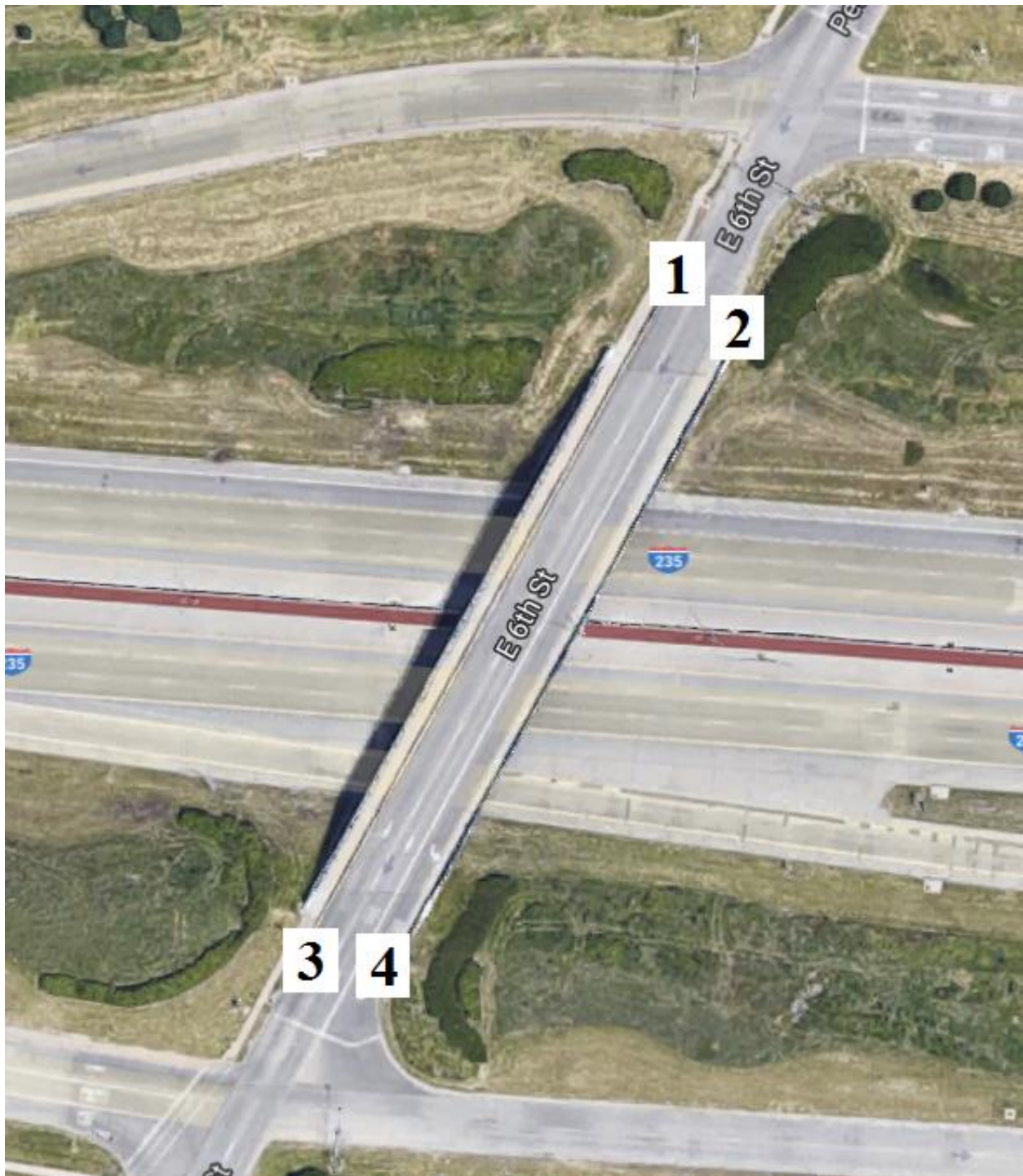
Figure B-131. Bridge No. 7708.8O235 [1]
