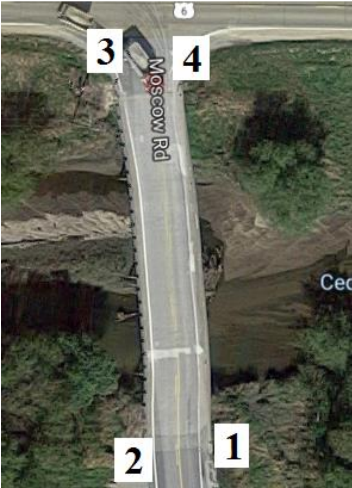
Figure B-109. Bridge No. 7078.0A006 [1]
