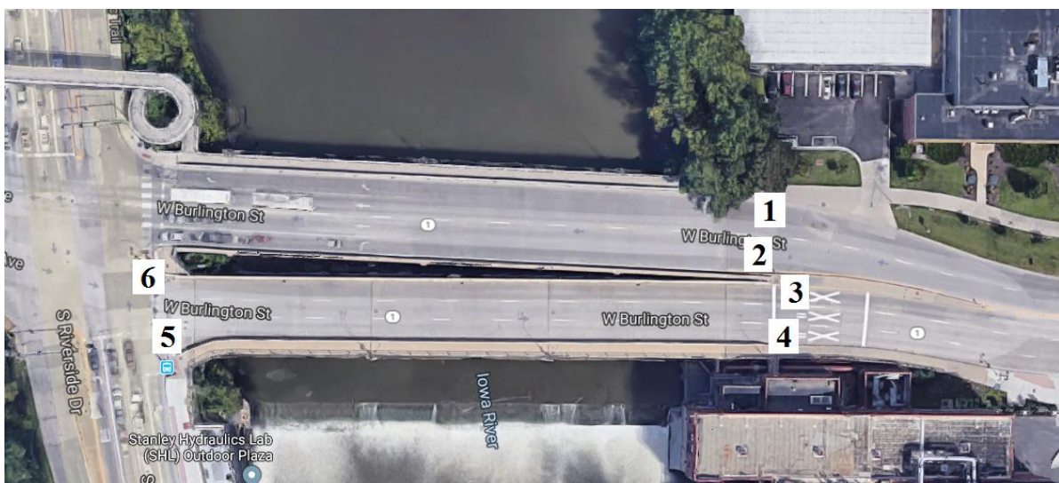
Figure B-81. Bridge No. 5285.9L001 [1]
