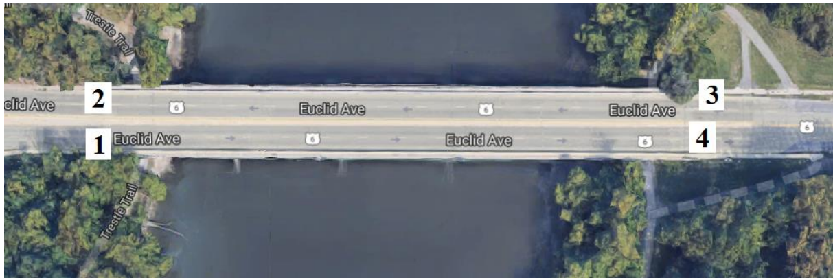
Figure B-143. Bridge No. 7735.4S006 [1]
