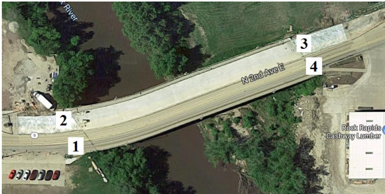
Figure B-102. Bridge No. 6020.4S009 [1]
