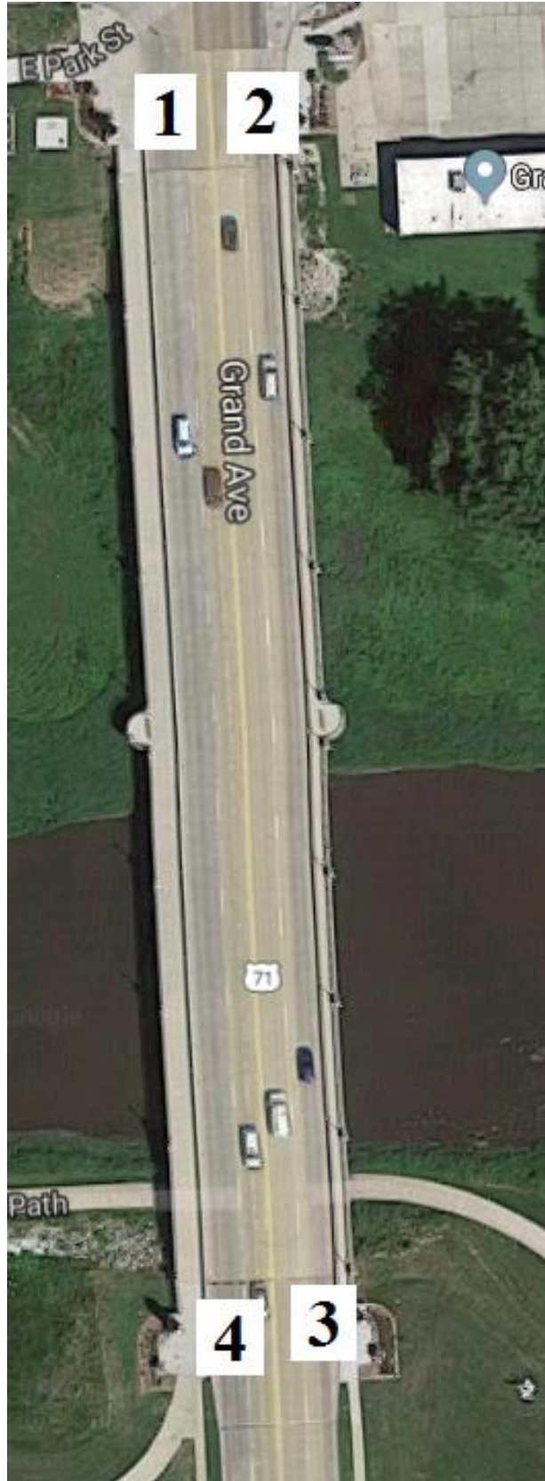
Figure B-28. Bridge No. 2181.0S018 [1]
