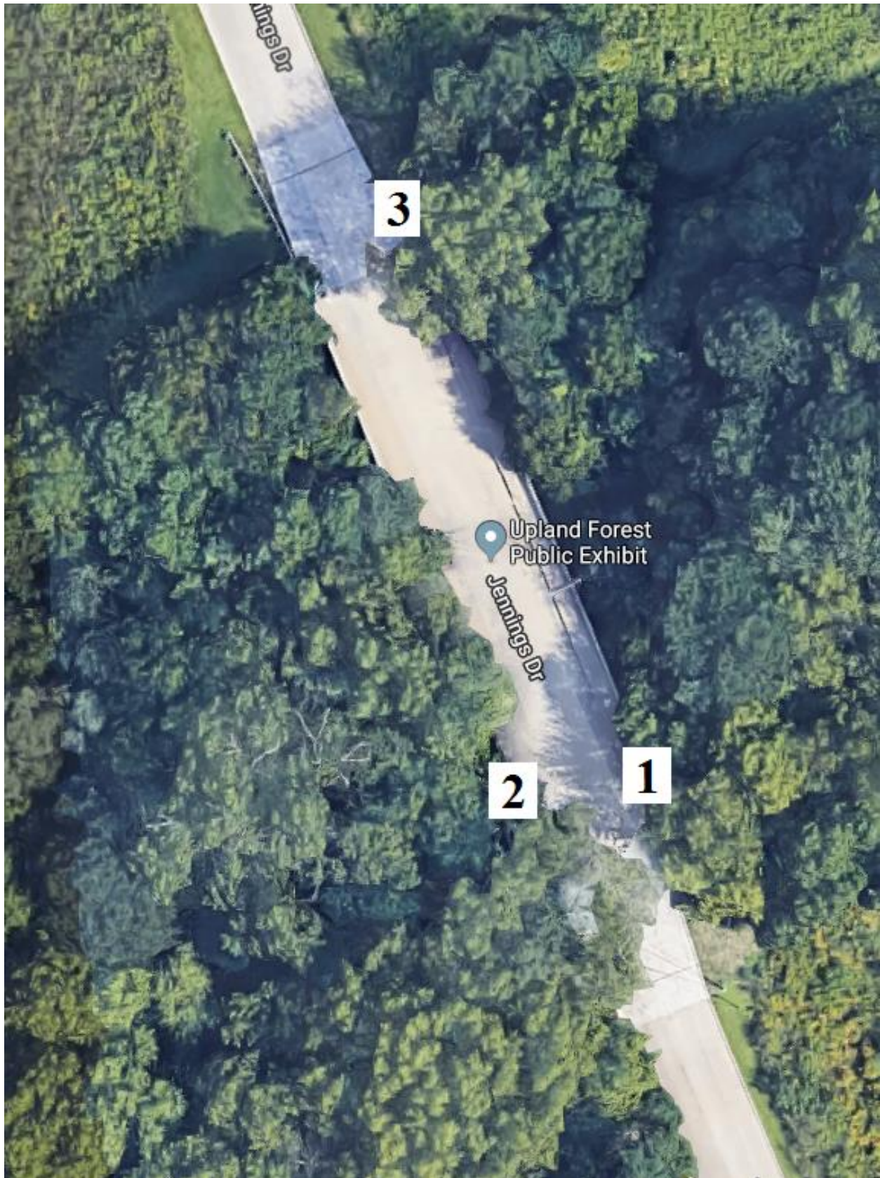
Figure B-4. Bridge No. 0700.4S820 [1]
