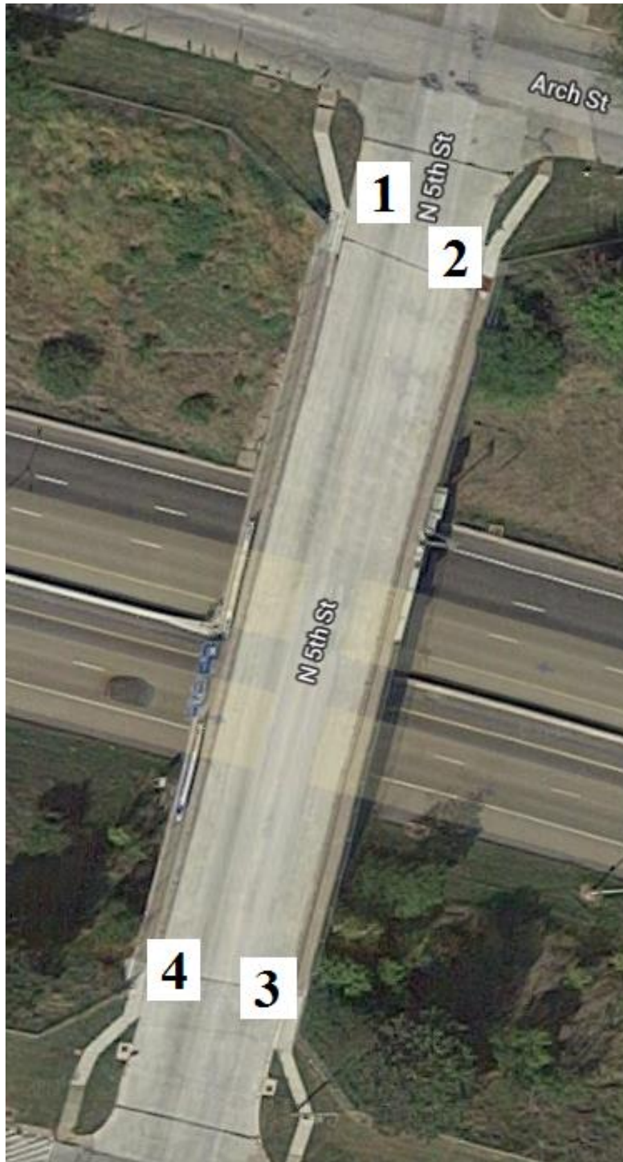
Figure B-44. Bridge No. 2963.2O034 [1]
