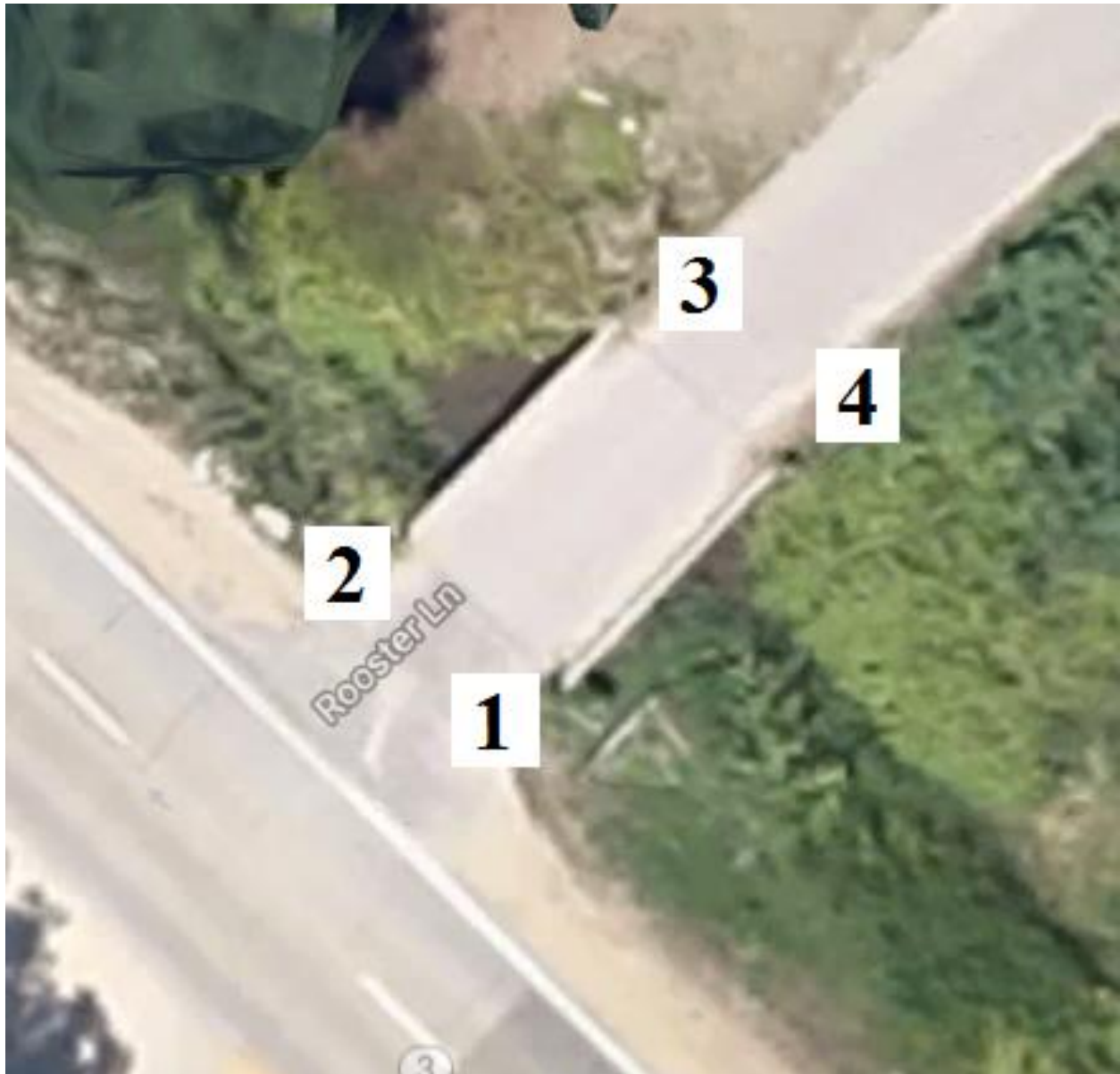
Figure B-54. Bridge No. 3150.7A052 [1]
