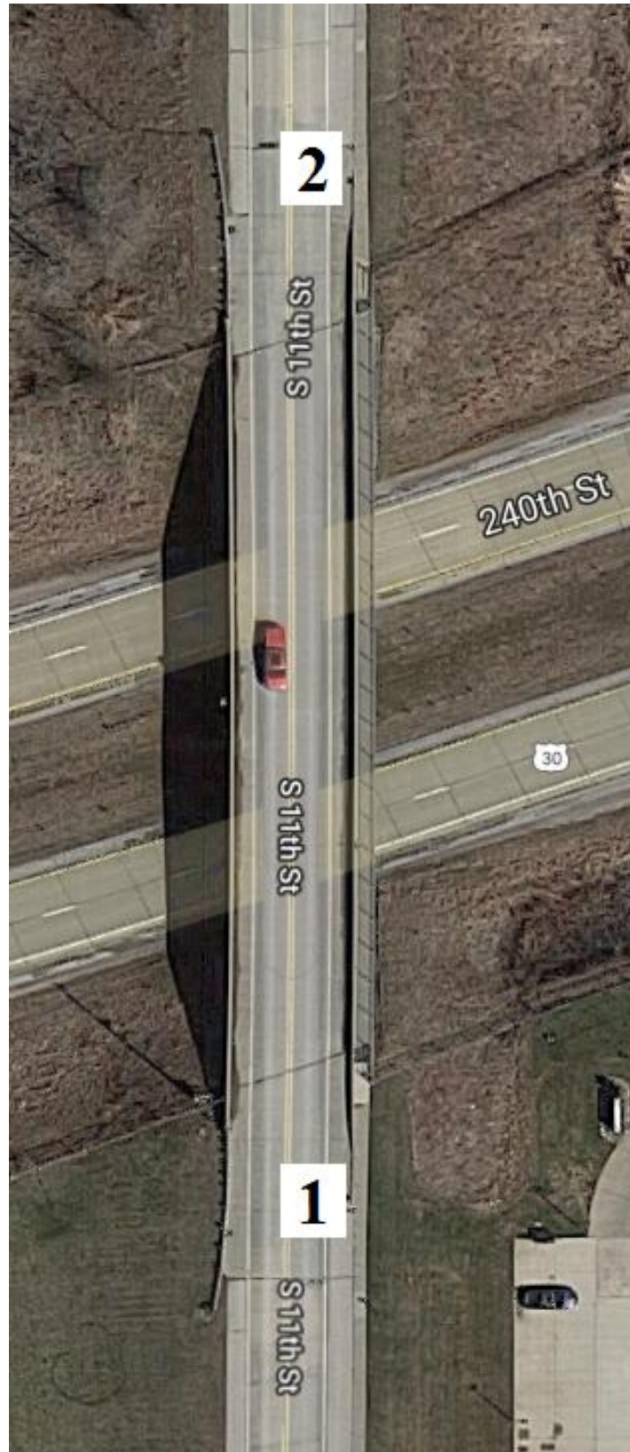
Figure B-162. Bridge No. 8557.9O030 [1]
