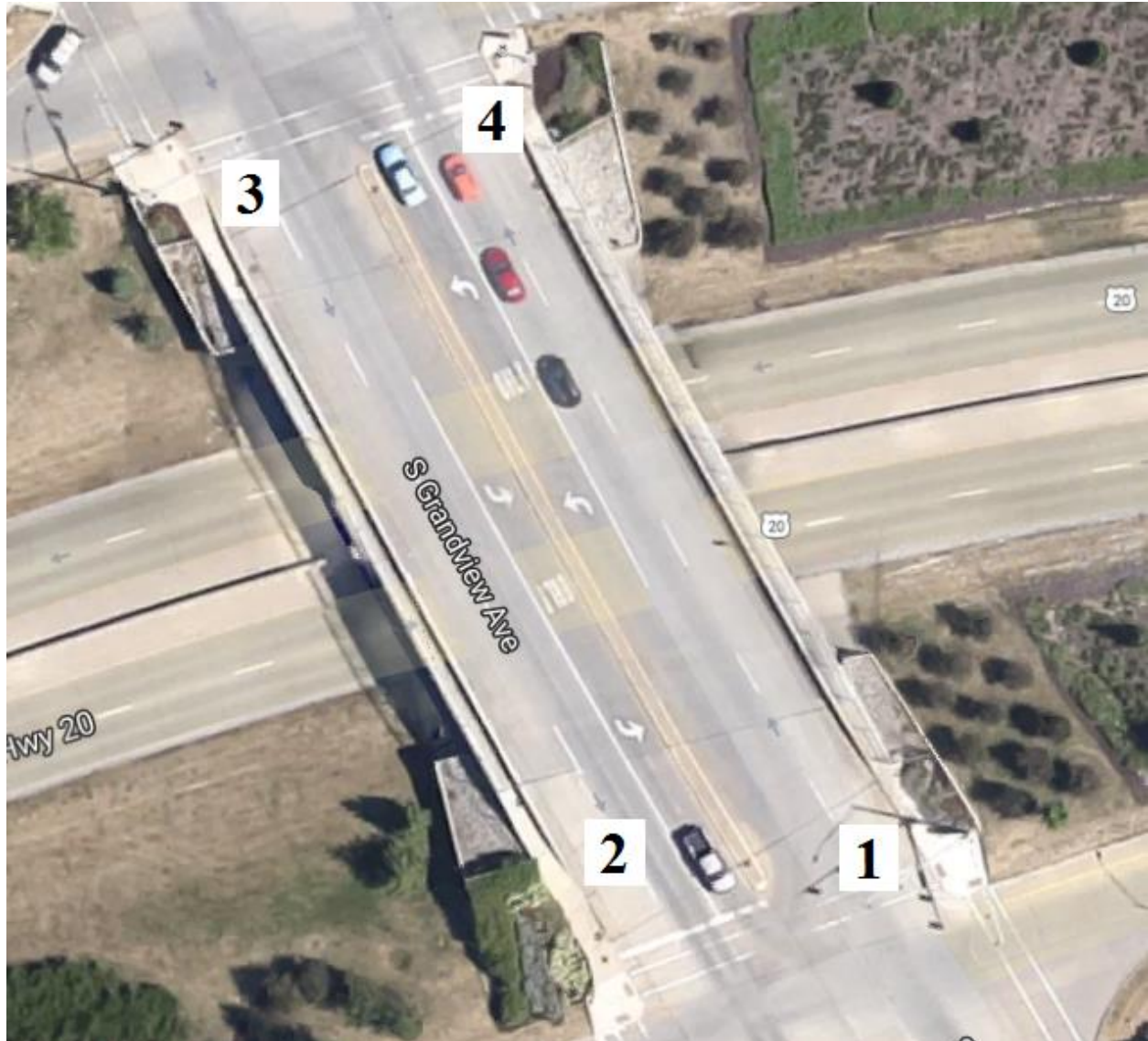
Figure B-50. Bridge No. 3118.5O020 [1]
