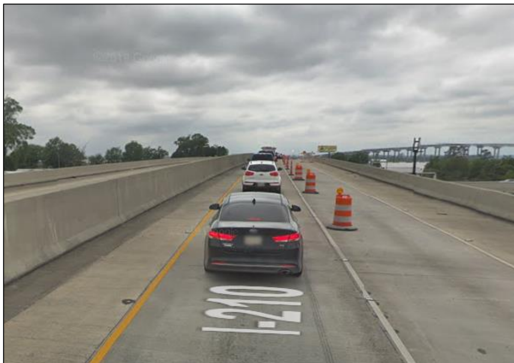
Figure 31. Right lane closure on I-210
