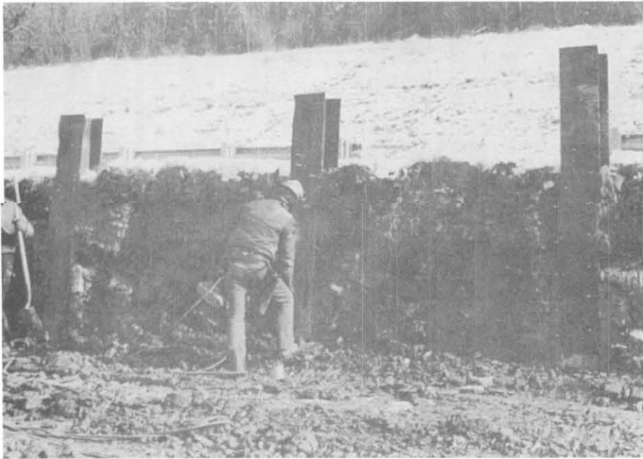
Figure 8. Piling in Place and Excavation of Embankment.
