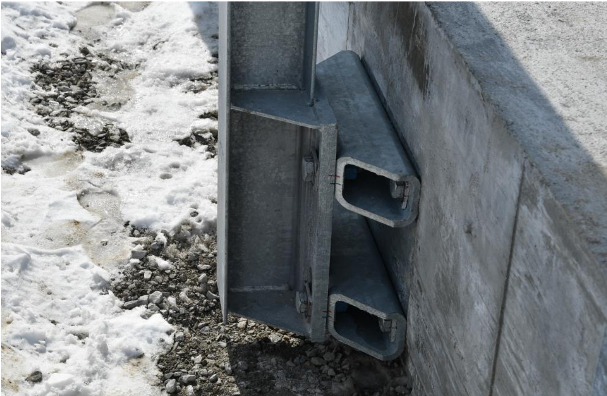
Figure 211. Side-Mounted Post-to-Deck Connections, Test No. STBR-2
