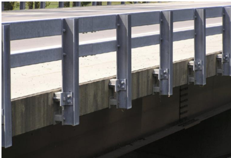
Figure 1. Steel, Side-Mounted, Beam-and-Post, Bridge Rail [1]
