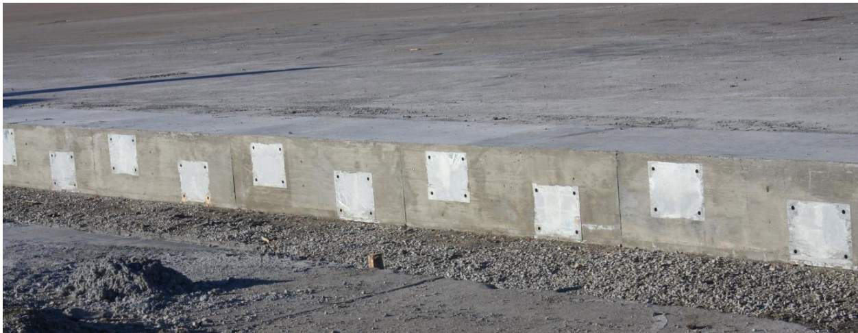
Figure 102. Surrogate Concrete Bridge Deck
