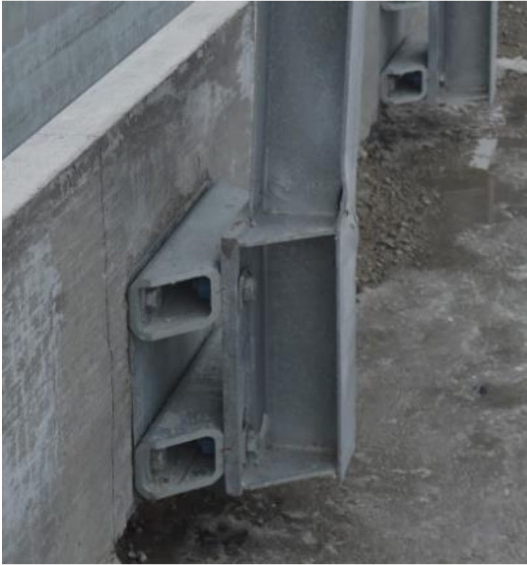
Figure 222. System Damage, Post No. 8, Test No. STBR-2
