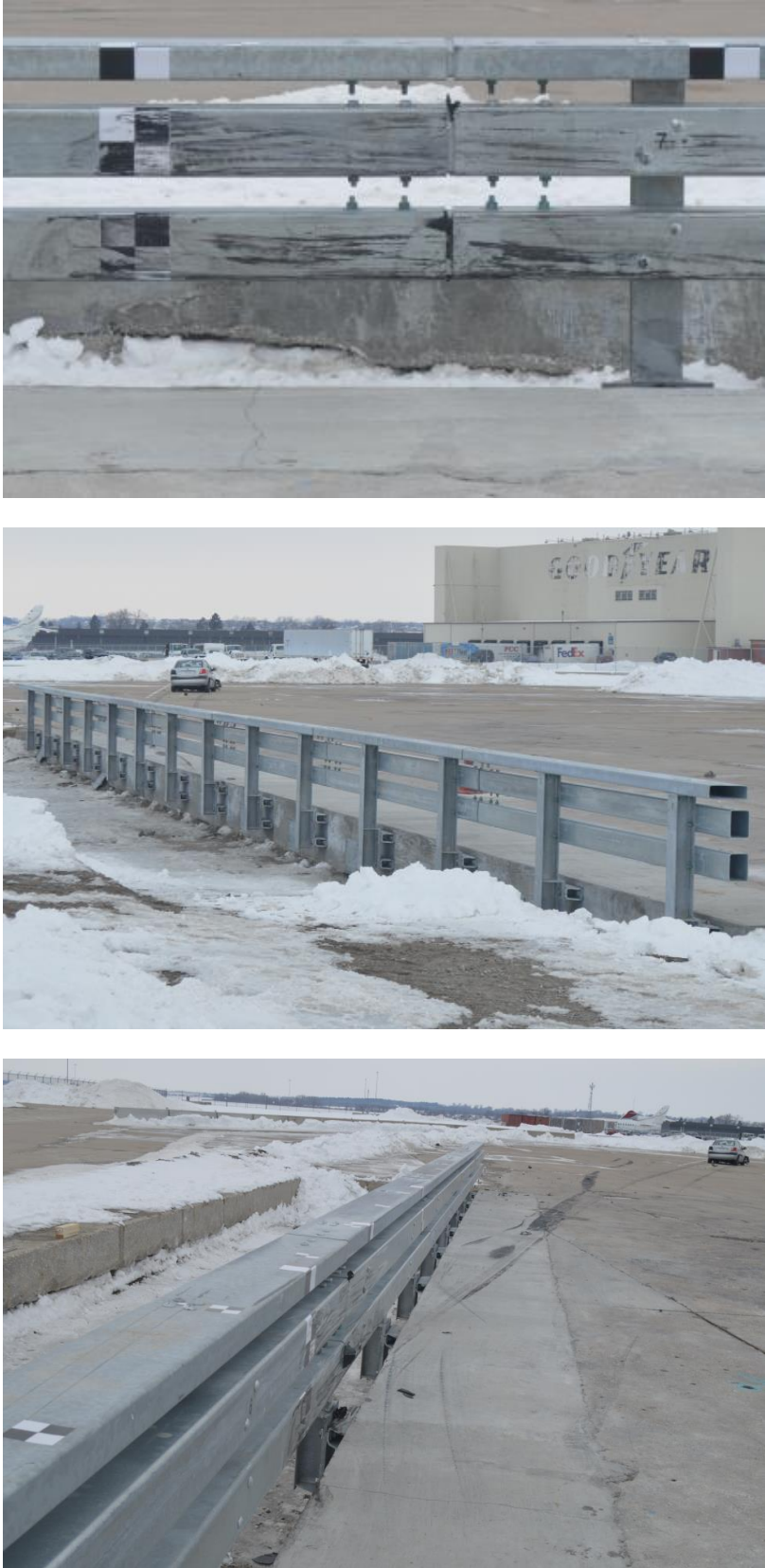
Figure 268. System Damage, Test No. STBR-3
