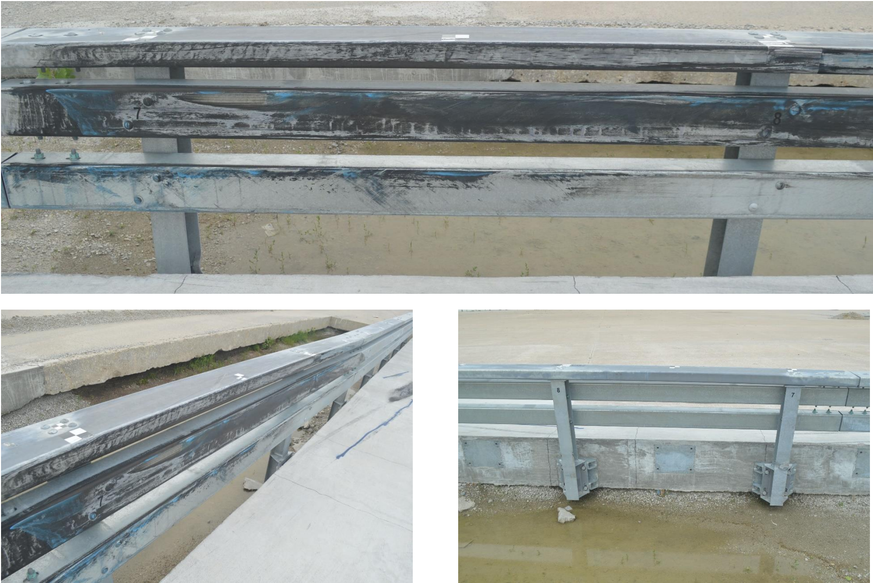
Figure 321. System Damage, Rail Span Between Posts Nos. 7 and 8, Test No. STBR-4
