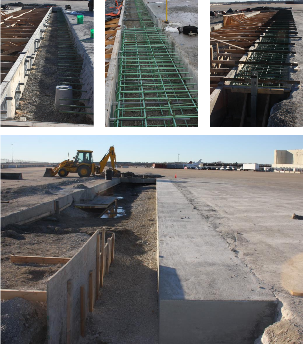
Figure 105. Construction of Surrogate Concrete Bridge Deck
