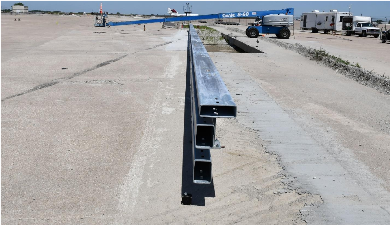
Figure 308. Test Installation Photographs, Bridge Railing End Views, Test No. STBR-4
