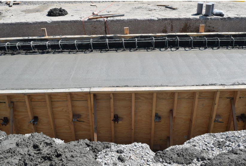
Figure 20. Concrete Top Slab and Headwall Construction, Test Nos. CMGS-1 and CMGS-2
