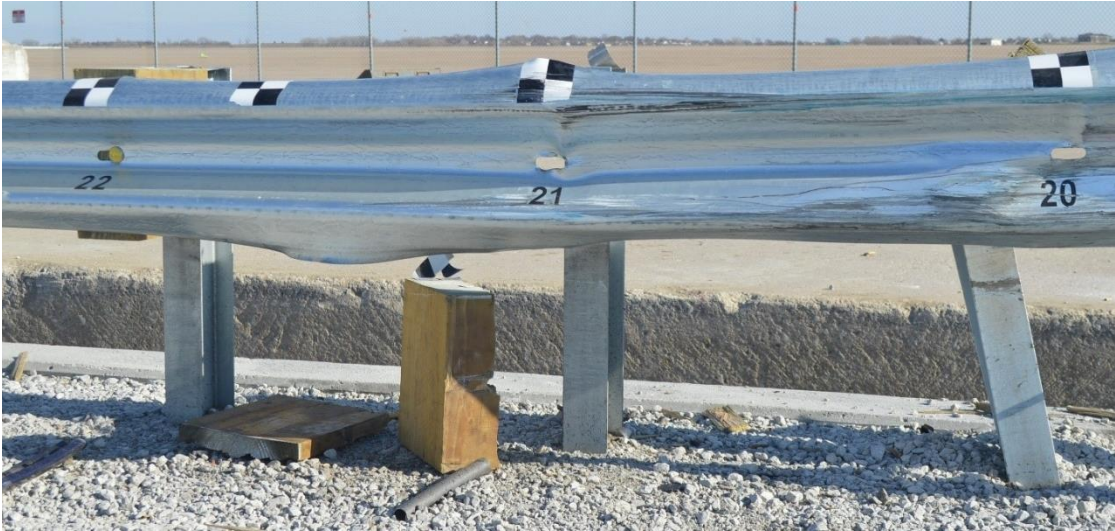
Figure 61. Damage to Post Nos. 15 through 22, Test No. CMGS-1
