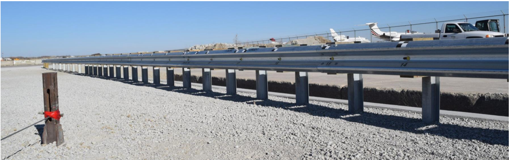
Figure 41. System Installation, Test Nos. CMGS-1 and CMGS-2
