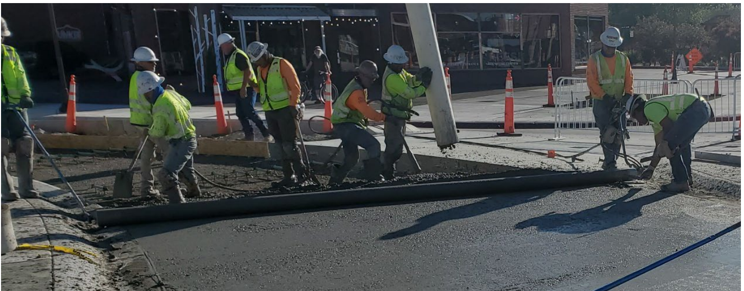
Figure 11. Single roller-tube vibratory screed used on a roundabout.
