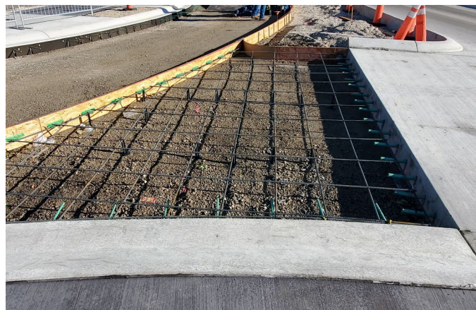
Figure 9. Example of steel reinforcement in an odd-shaped slab.
