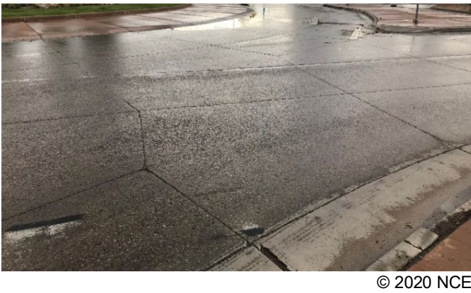
b. Odd-shaped panels in transition pavement.
