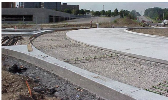
a. Dowel bar placement.
