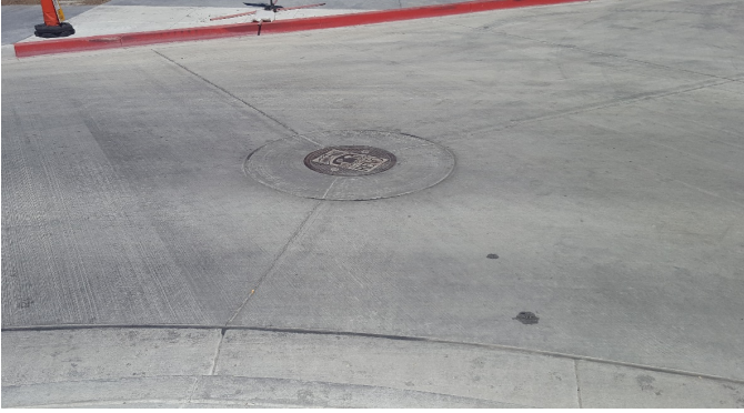
Figure 6. Example of a utility structure boxout and associated jointing.
