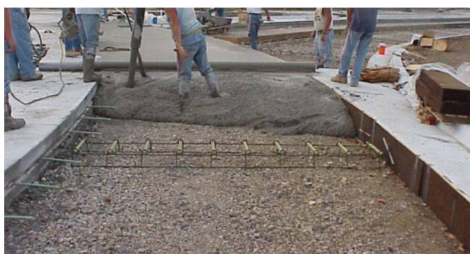
b. Tie bar and dowel bar placement.
