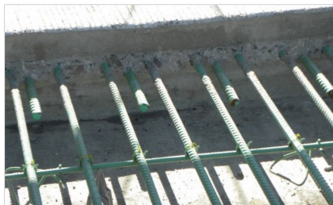
b) CRCP transverse construction joint.
