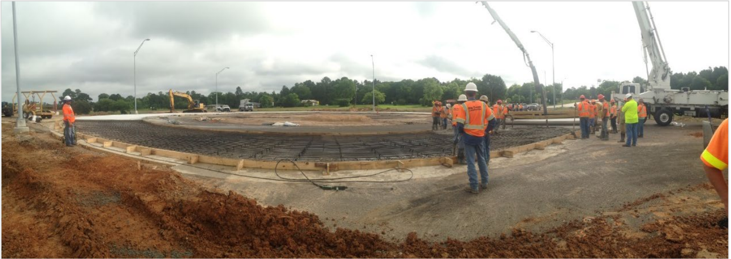
Figure 12. Formwork for the Walker County CRCP roundabout.
