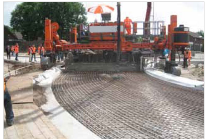
Figure 3. View of a European CRCP roundabout construction.
