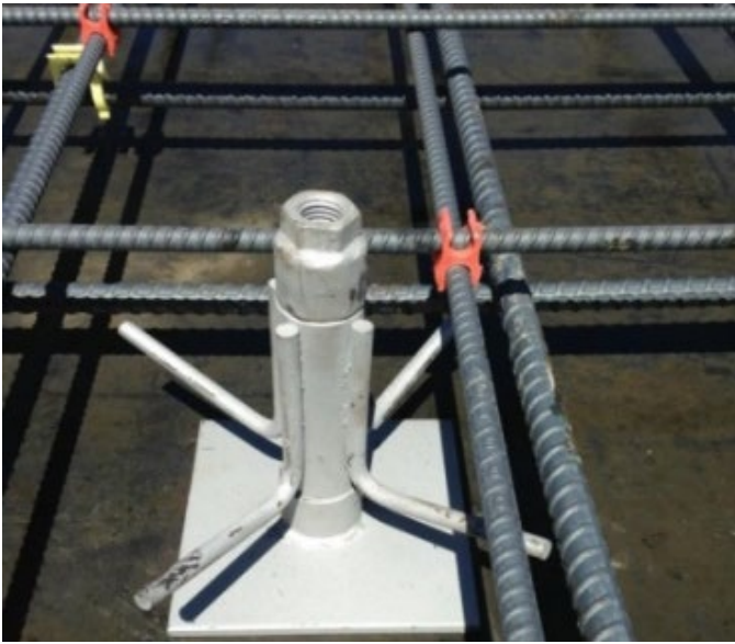
a. Panel leveling-lift.
