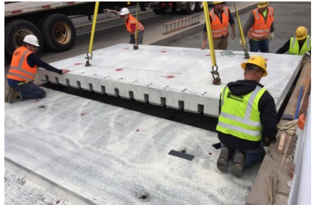
Figure 8. A PCP panel with dowel bar slots at the bottom.
