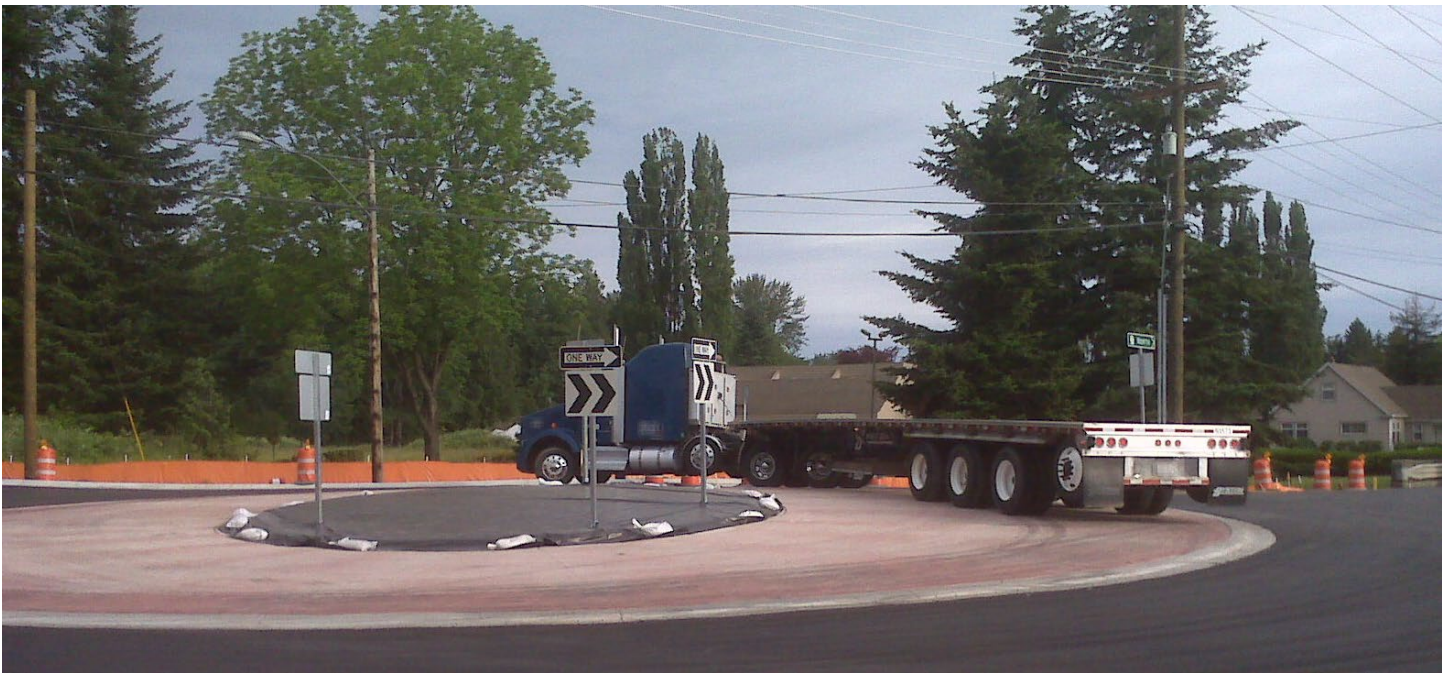
Figure 6. Truck traversing apron in HMAP roundabout.
