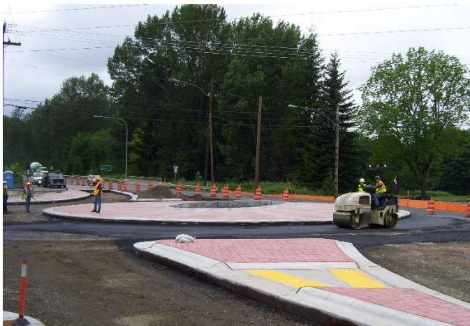
Figure 10. Vibratory steel-wheel roller compacting the first lift of a new roundabout.
