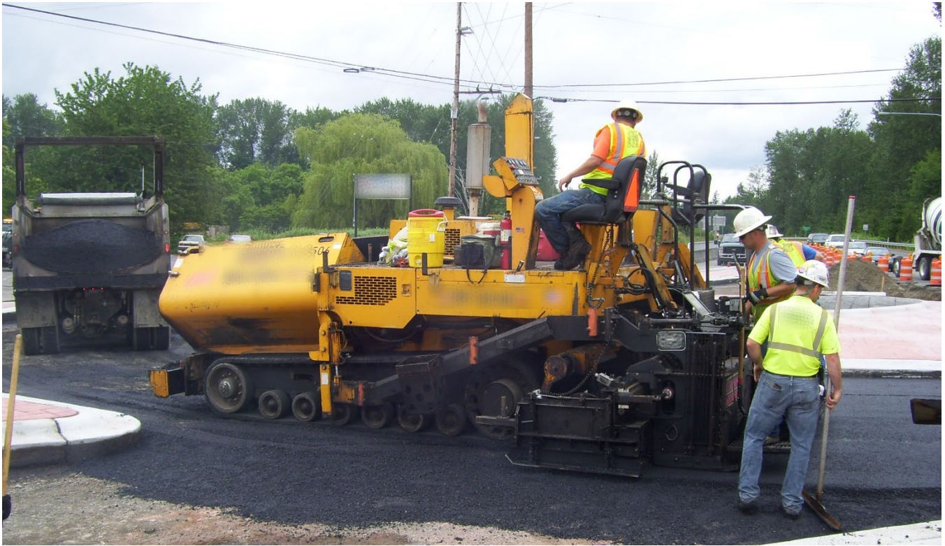
Figure 8. Close-up of paver placing HMA along the outer perimeter of a roundabout.
