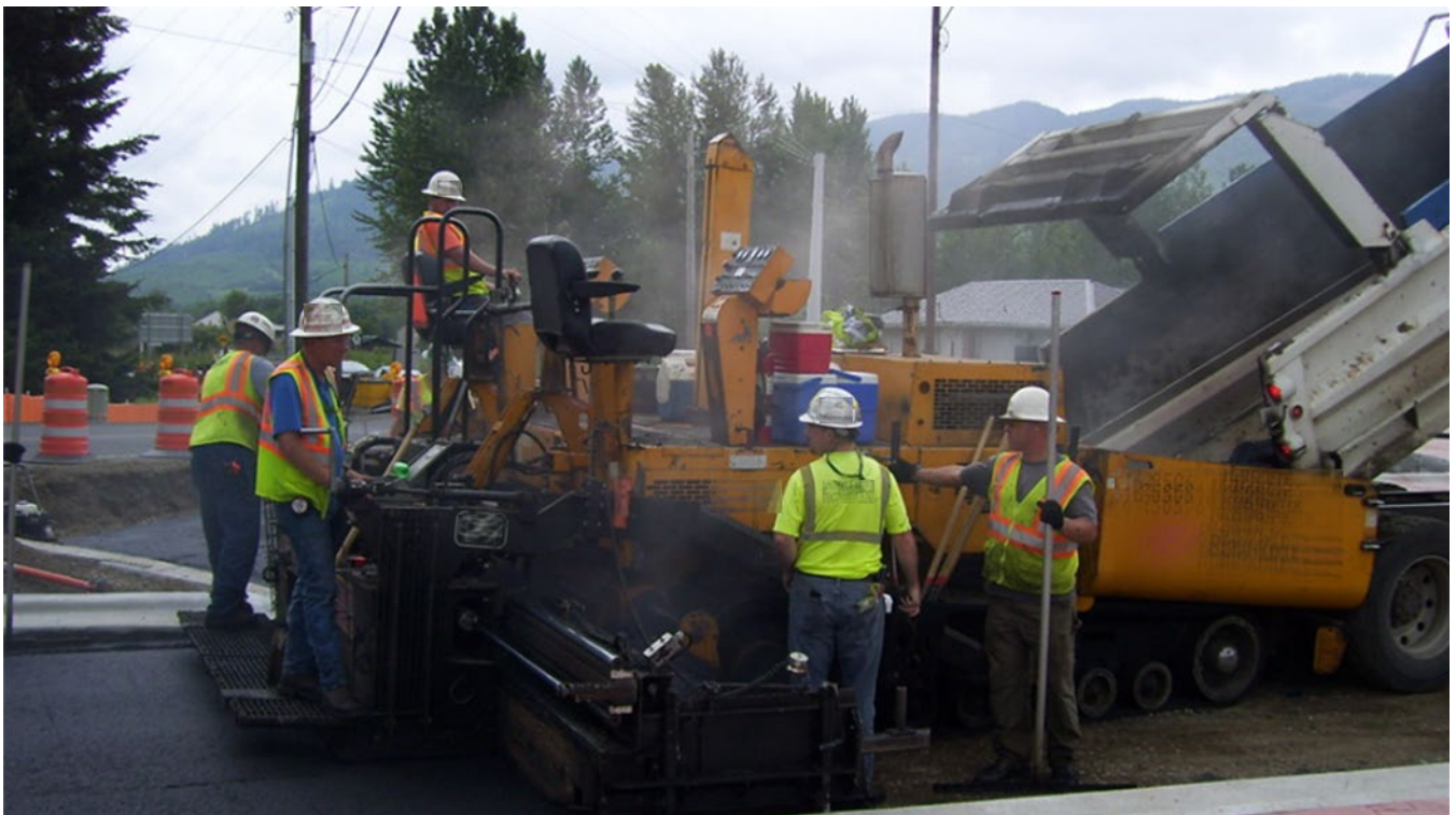
Figure 9. Paver with screed extended to pave the entire 16-ft width of an entry lane.
