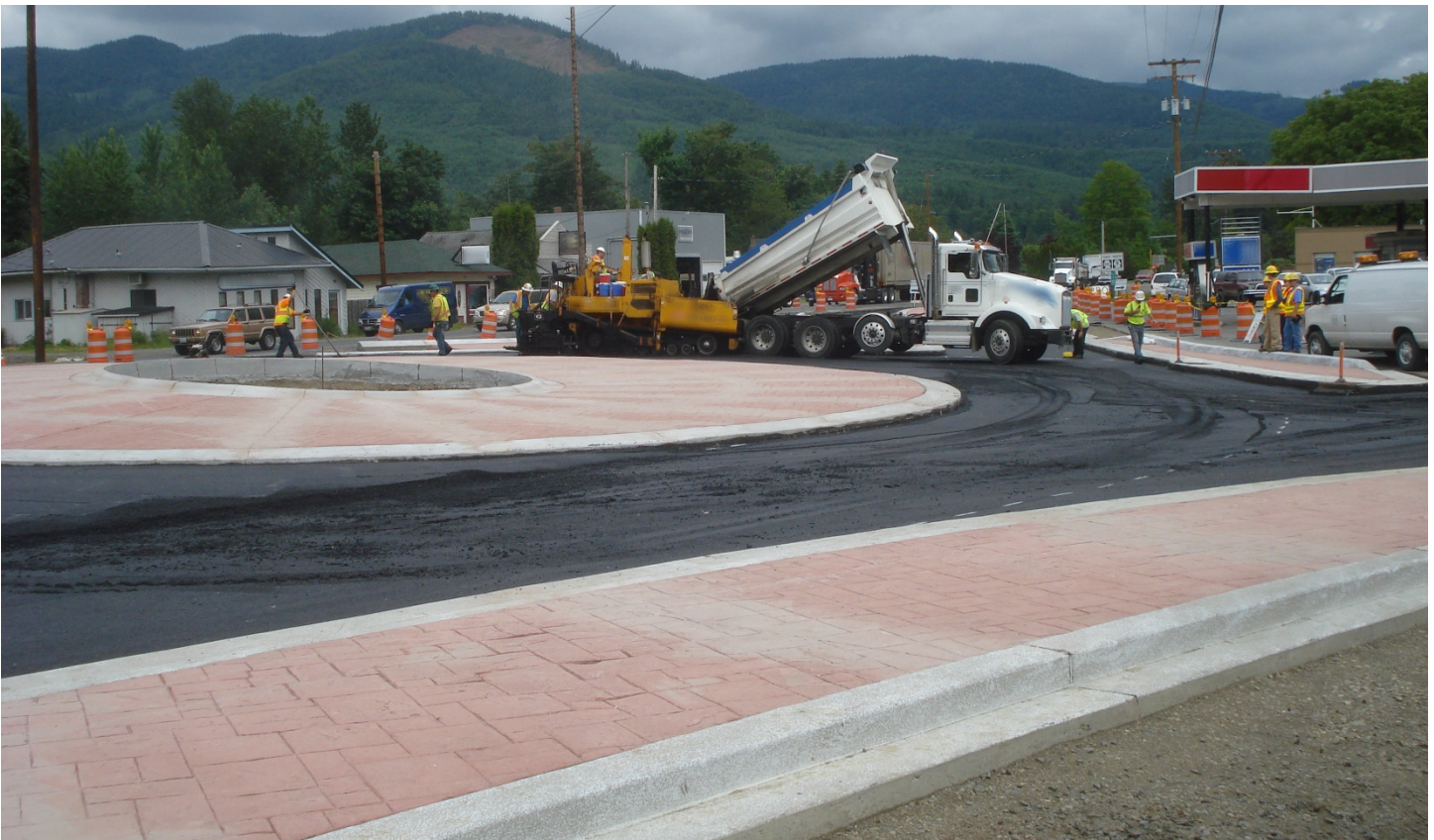
Figure 7. Loading asphalt mixture into the paver hopper using a short end-dump truck.
