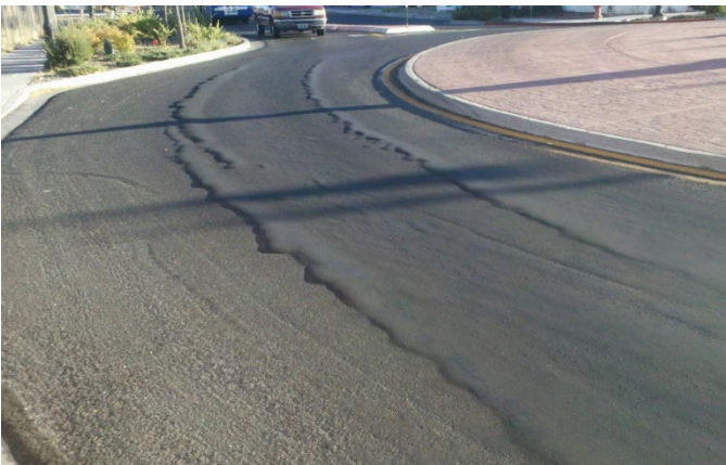
Figure 5. HMA roundabout exhibiting rutting and shoving in wheelpaths.
