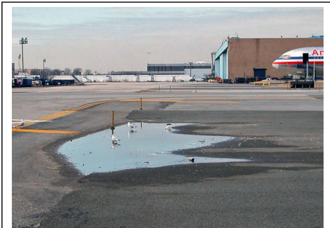
Standing water at airports is a strong attractant for gulls and other birds and should be eliminated. Photo, R. Dolbeer, USDA.
