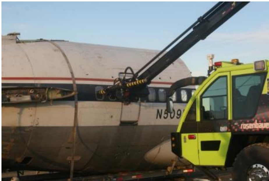
Figure 132. Window Removal Using an HRET (Photograph courtesy of FAA (2010))
