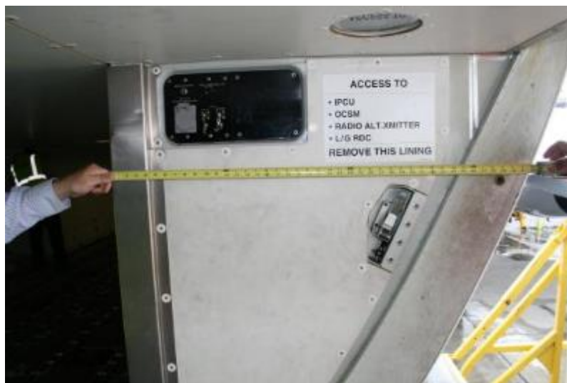
Figure 141. Cheek Area Inside Rear Cargo Compartment (42 in.) (Photograph courtesy of FAA)
