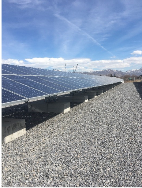
Salt Lake City-owned solar array (Image source: Volpe Center).
