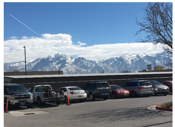
Solar parking lot canopy at UDOT headquarters (Image source: Volpe Center).
