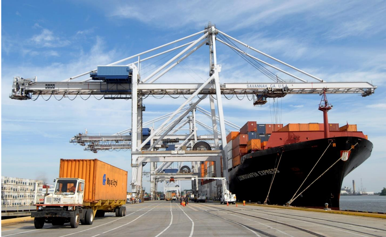
Figure 2.2: Ship-to-Shore Gantry Cranes (Source: Google Image)
