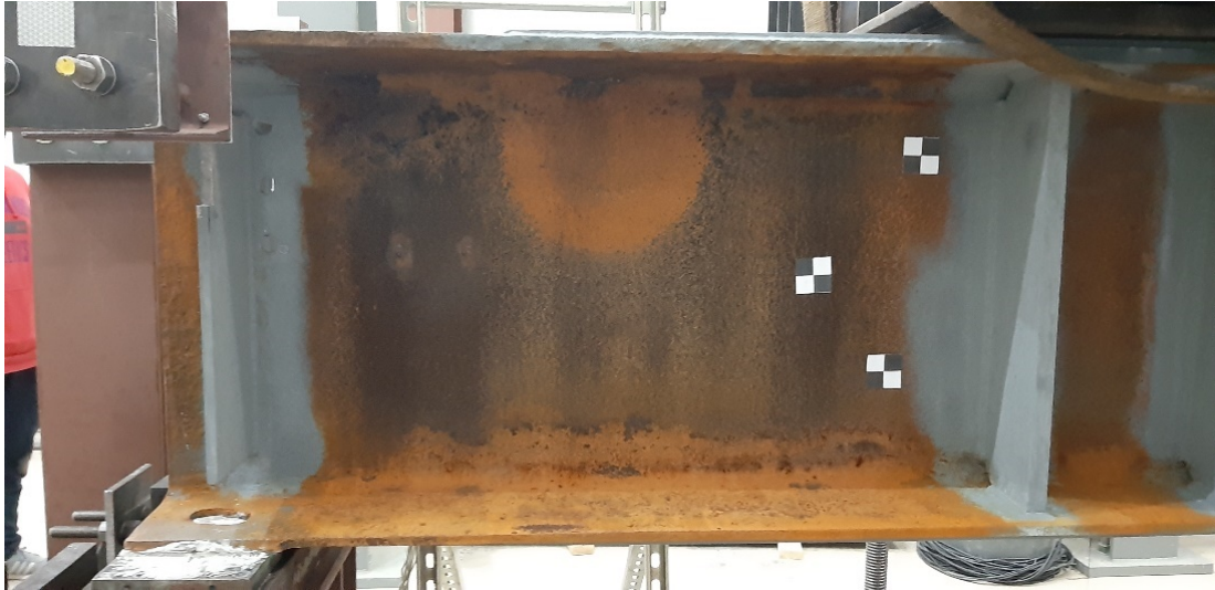
Figure 3.12: Corroded end of Specimen B
