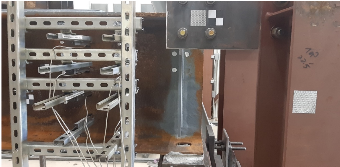
Figure 3.15: Instrumentation configuration at tested end of Specimen B
