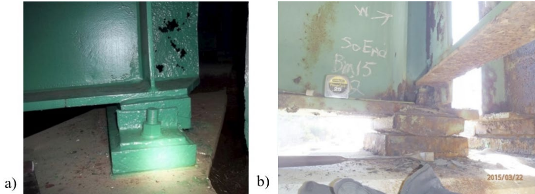
Figure 4.9: a) Expansion and b) fixed bearing types commonly found supporting corroded plate girders in Massachusetts
