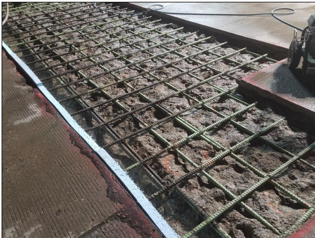
Figure 2.4.4.1 Localized Partial-Depth Hydrodemolition (UDOT 2017)
