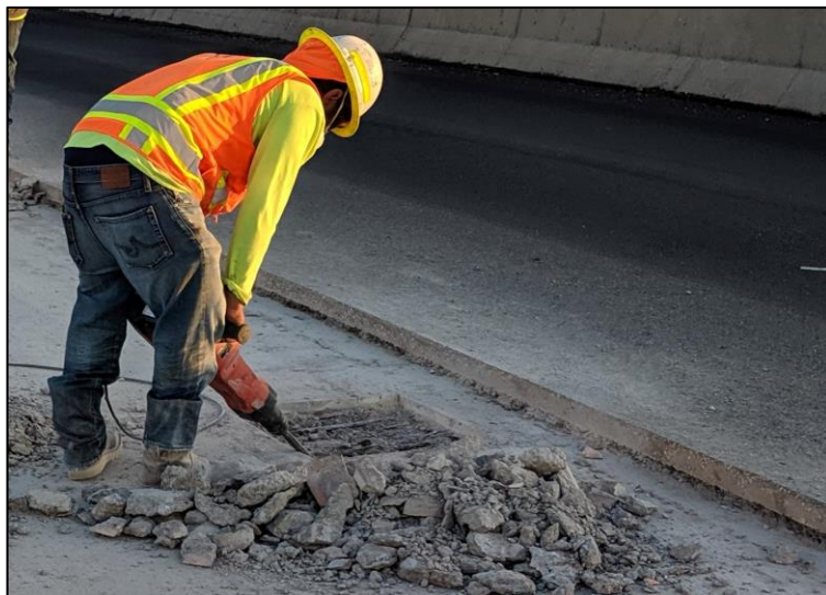
Figure 2.4.1.1 Chipping a Structural Pothole Patch (UDOT 2017)
