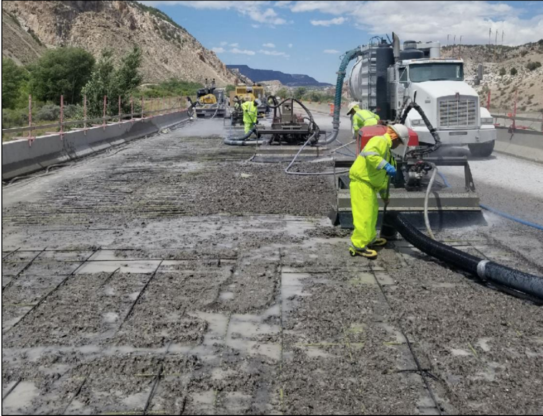
Figure 2.1.2 Partial Depth Hydrodemolition Deck Rehabilitation (REDI Services 2019)
