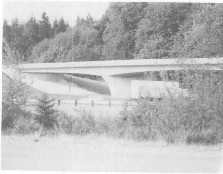
Figure 10. Continuous concrete box girder bridge- left abutment settled approximately 1.5 inches (38.1 mm) relative to the pier.
