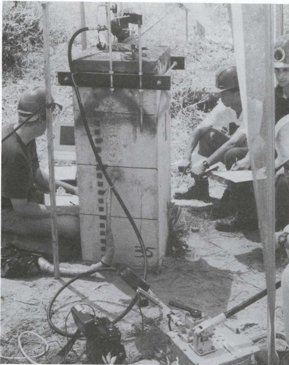
Figure 20.4 Osterberg Test in Progress on a 457 mm Concrete Pile (courtesy of Loadtest, Inc.)
