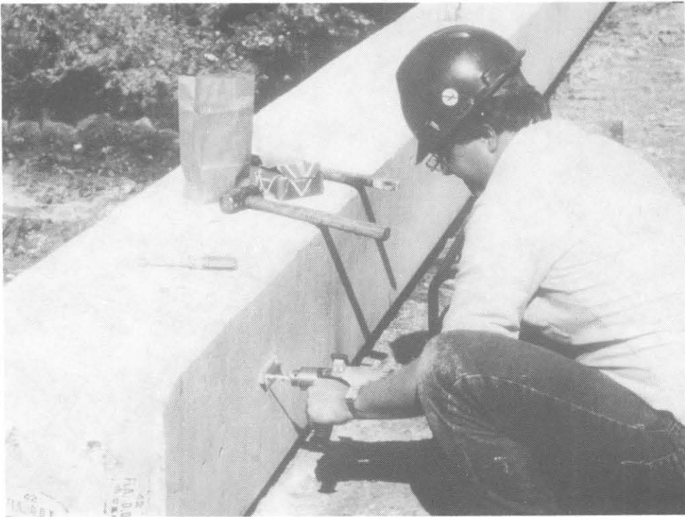
Figure 18.1 Pile Preparation for Dynamic Testing
