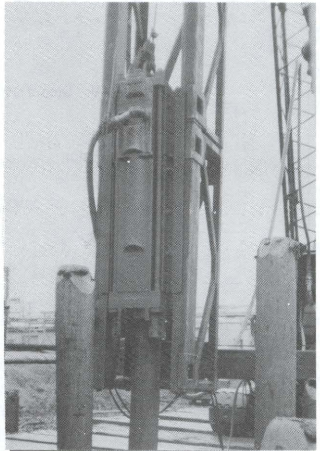
Figure 22.15 Double Acting Air Hammer
