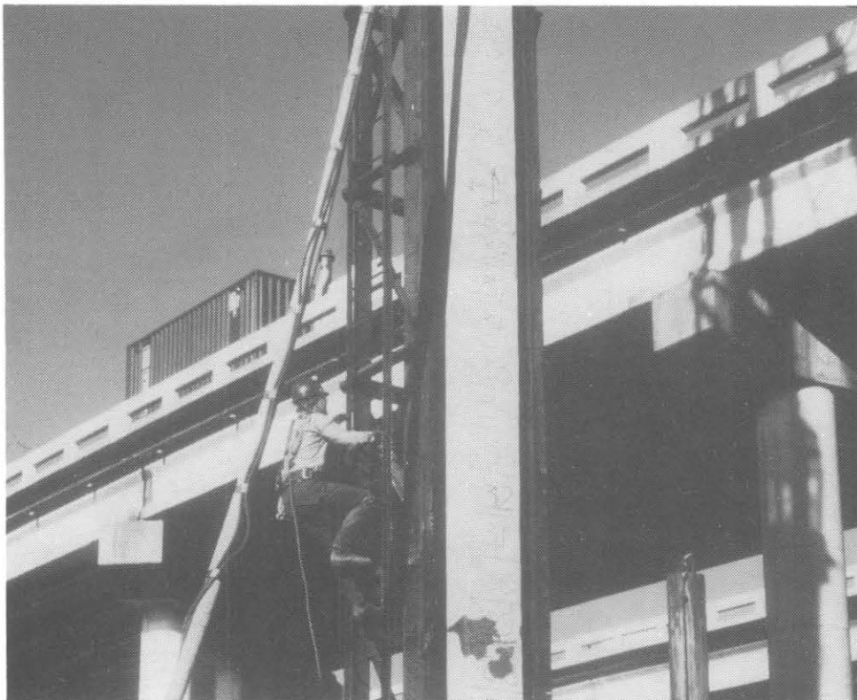
Figure 18.2 Pile Positioned for Driving and Gage Attachment
