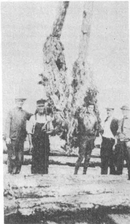
Figure 5 - Timber Pile Damage
