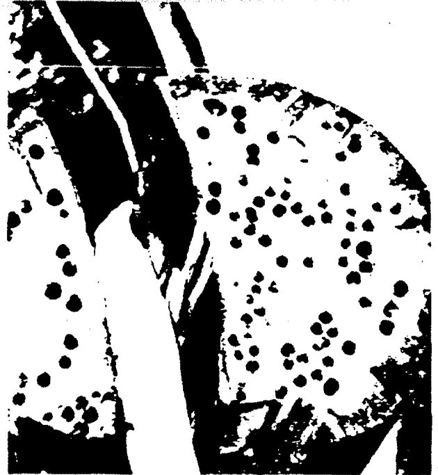
Figure 3-21 Section cut from a pile damaged by the teredo.
