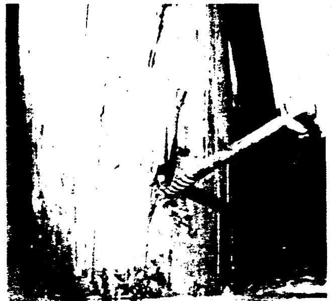
Figure 3-18 Marine borer damage to end of cross brace.
