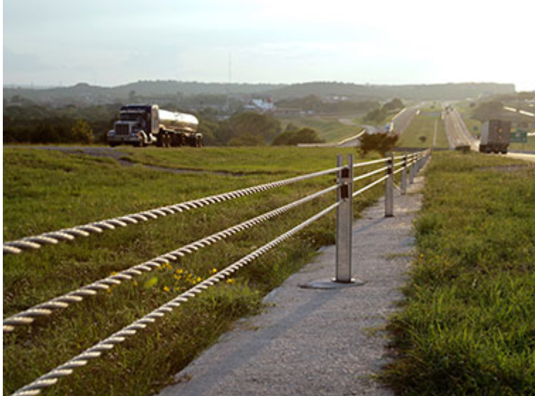
Figure 35. Example of a cable median barrier
