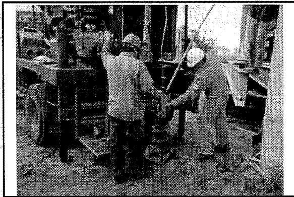
3.65 Inserting float out transmitter
