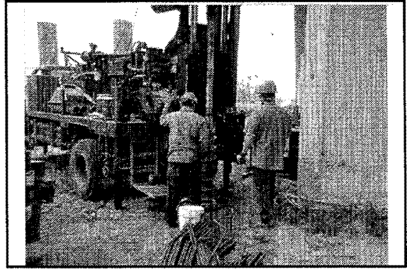
3.64 Hollow stem auger
