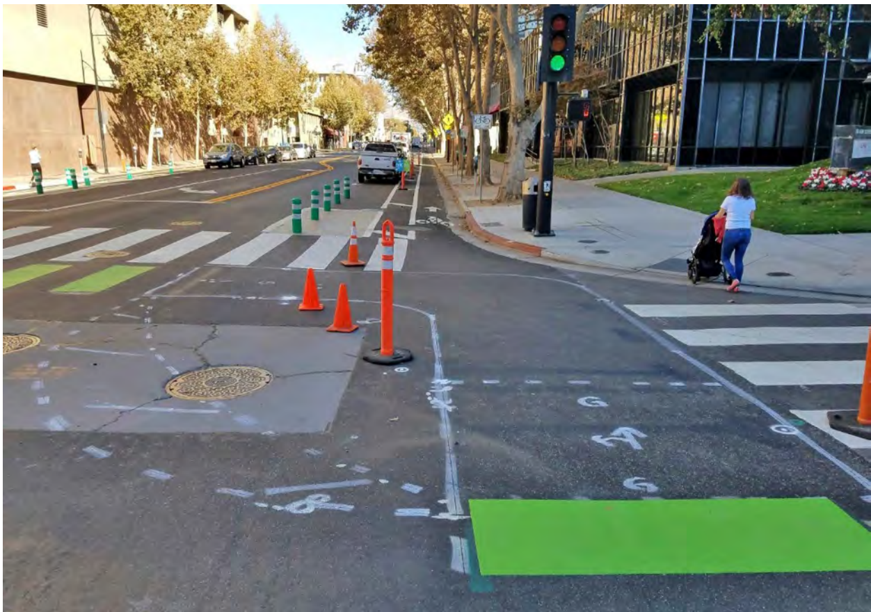
Figure 7. Photo. Field adjustments to enhance turn radii were identified during implementation of a quick-build buffer-separated bicycle lane project in San José, CA, USA. Source: Fehr & Peers.
