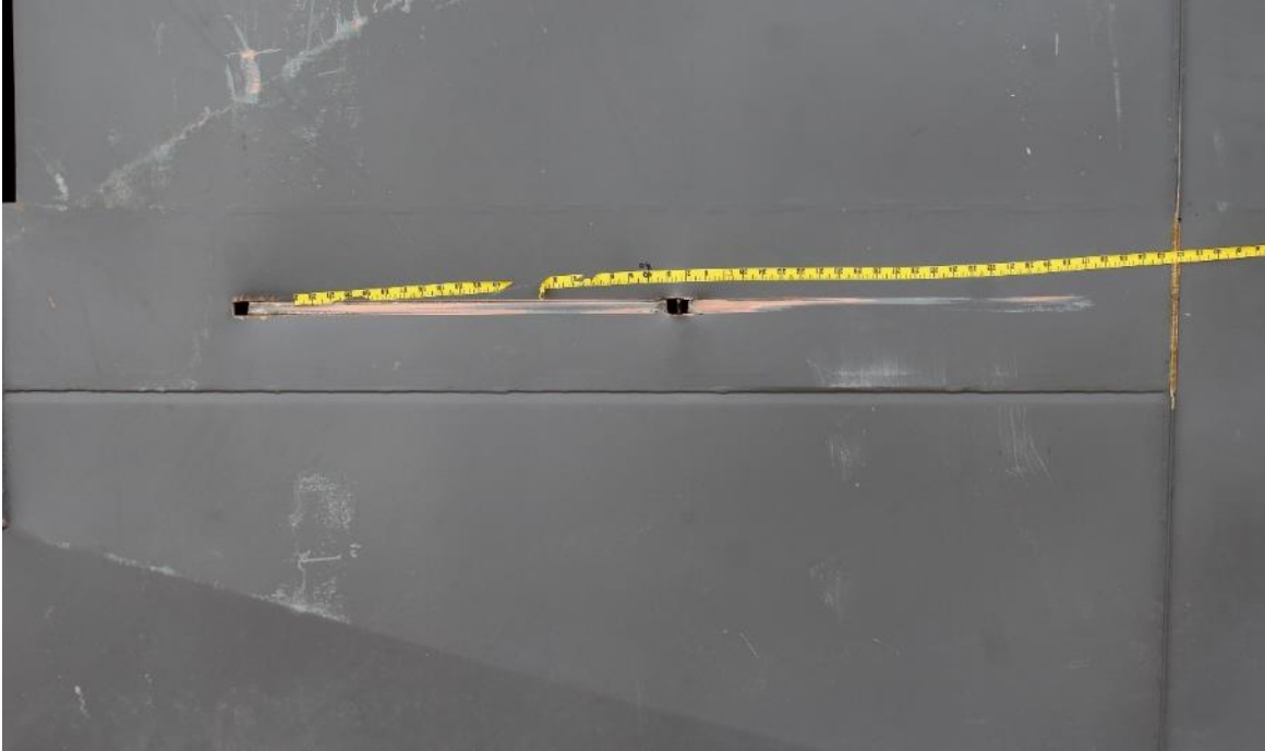
Figure 44. Tears in Test 2 Fuel Tank
