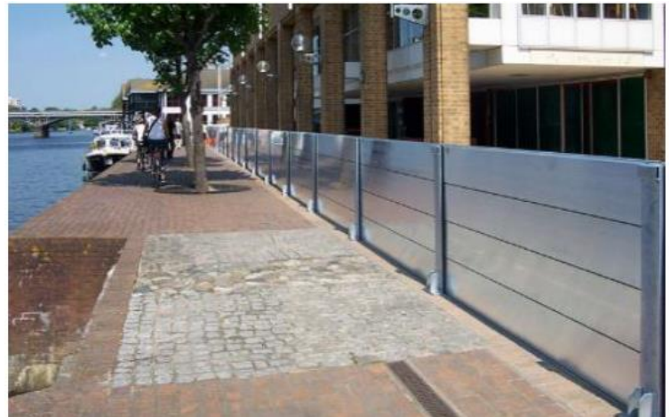
Figure 2. Example of drop-in flood barrier system. Source: MassDOT.
