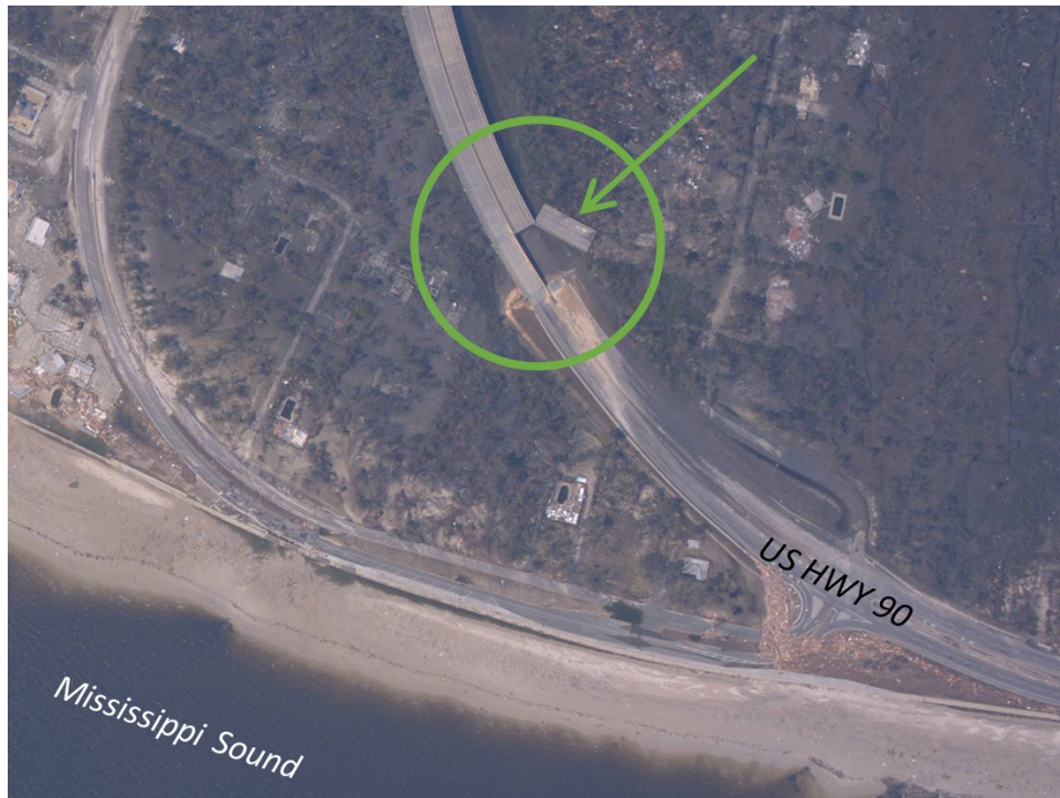
Figure 3. Image showing damage to Henderson Point bridges during Hurricane Katrina (Photo credit: NOAA).
