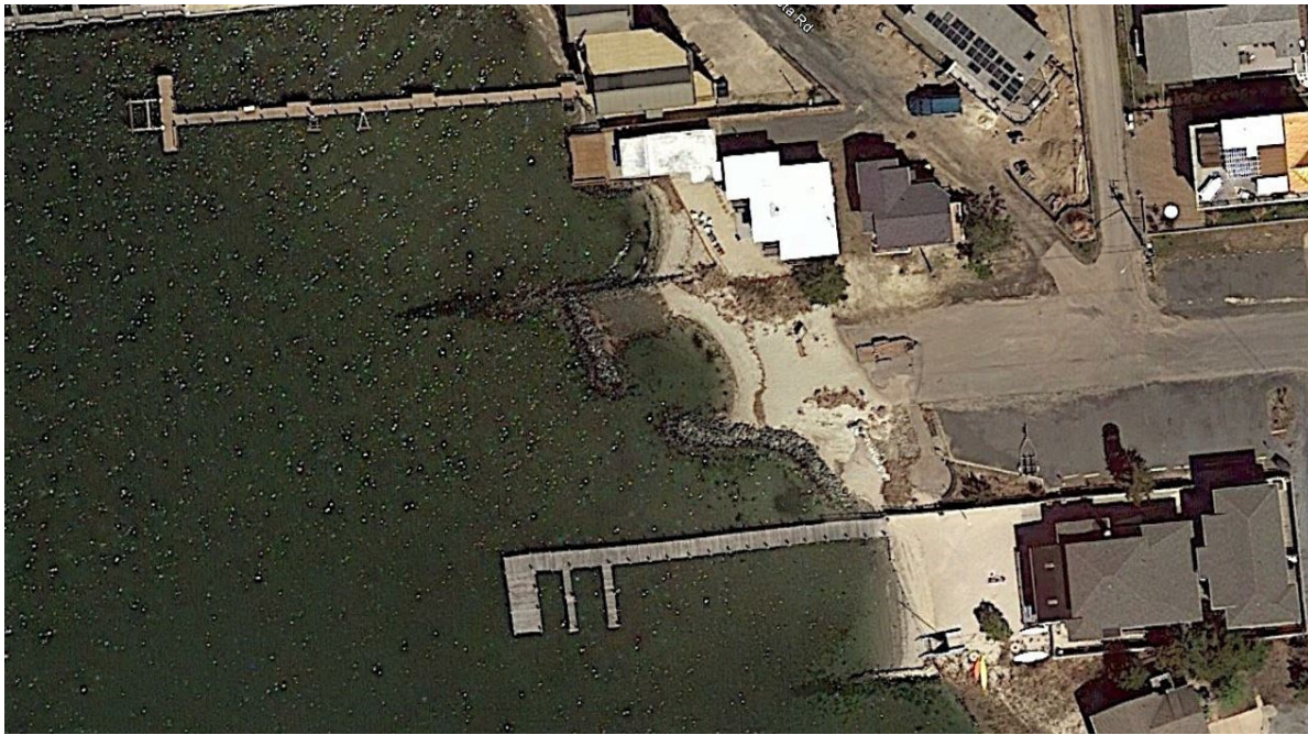
Figure 189 - Read Avenue Existing Conditions (Plan View - Not to Scale). Map Credit: Google Earth, Map©2018Google.
