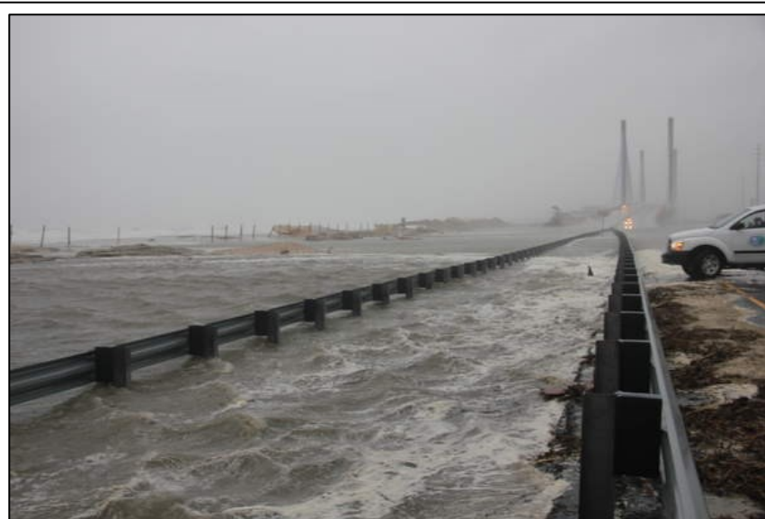
Figure 2 - Storm surge affecting the oceanside lane of Route 1 just north of Indian River Inlet Bridge. Source: capegazette.villagesoup.com (Image by: Dennis Forney)
