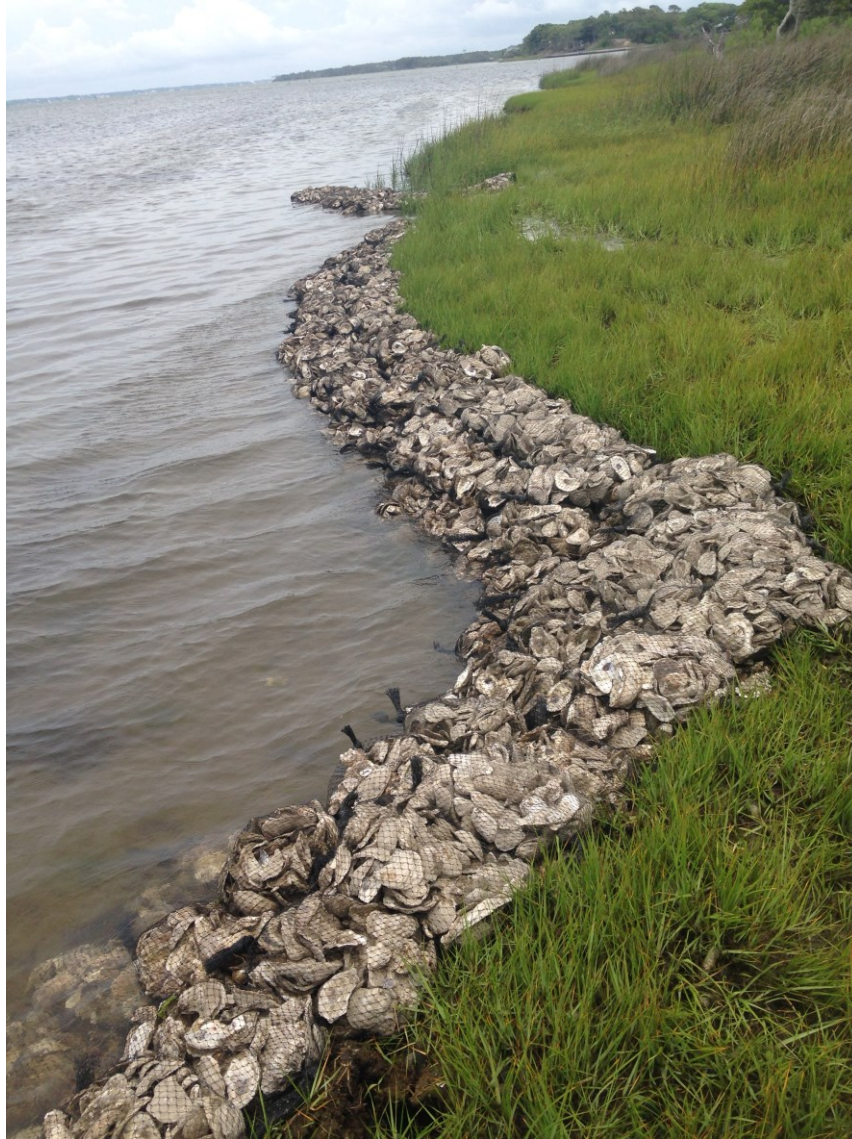
Figure 24 – Oyster Bags Applied in Practice. Source: DelDOT
