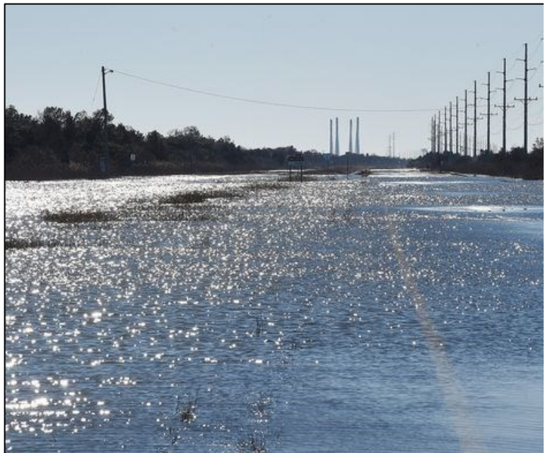
Figure 4 - Coastal Highway flooding between Dewey Beach and Indian River Inlet. Source: delawareonline.com
