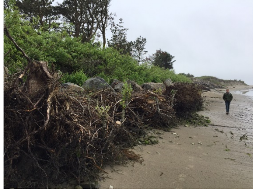
Root wad seawall (Photo credit: BioEngineering Associates)
