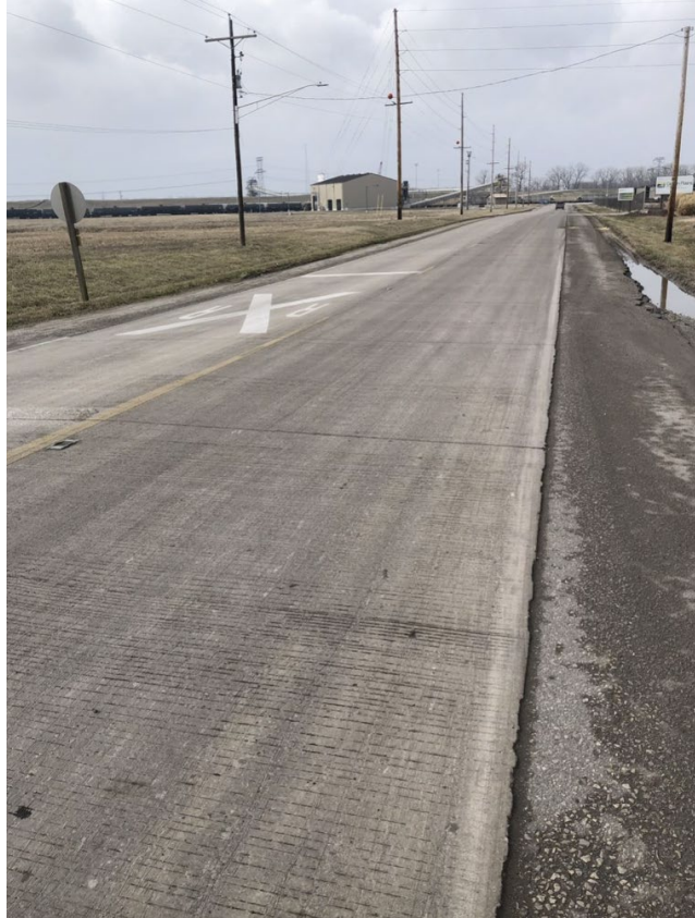
Figure 121. Photos. Bissel Road.
