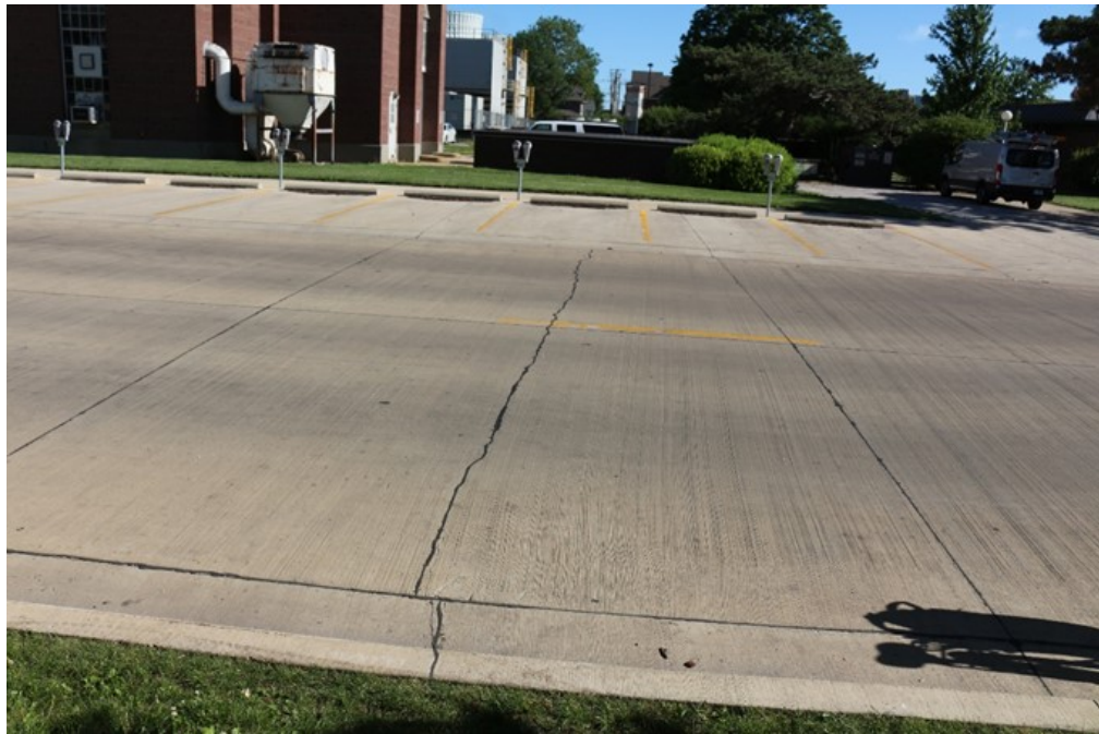
Figure 72. Photo. Gregory Drive from Oak Street to First Street.
