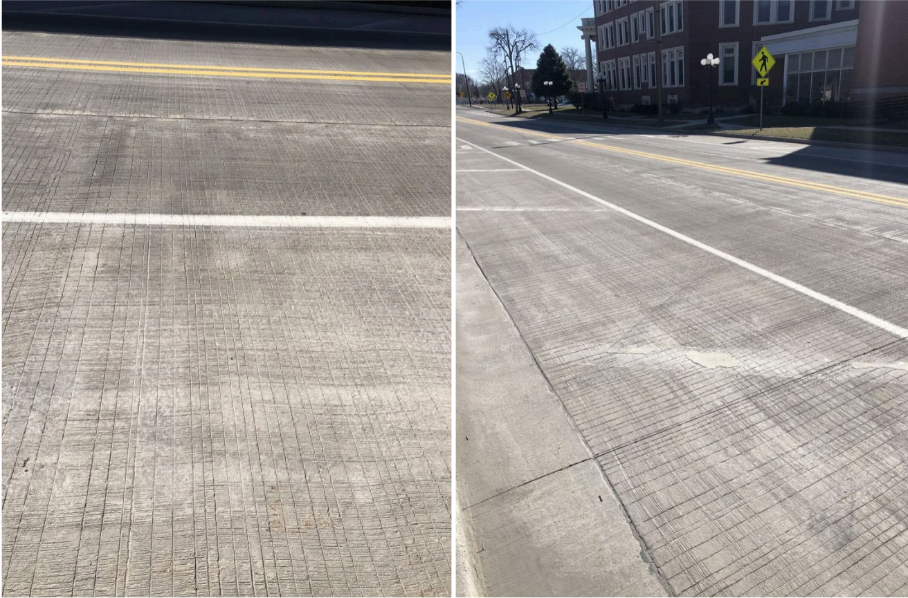
Figure 49. Photos. Marmont Street with Dwight Street.
