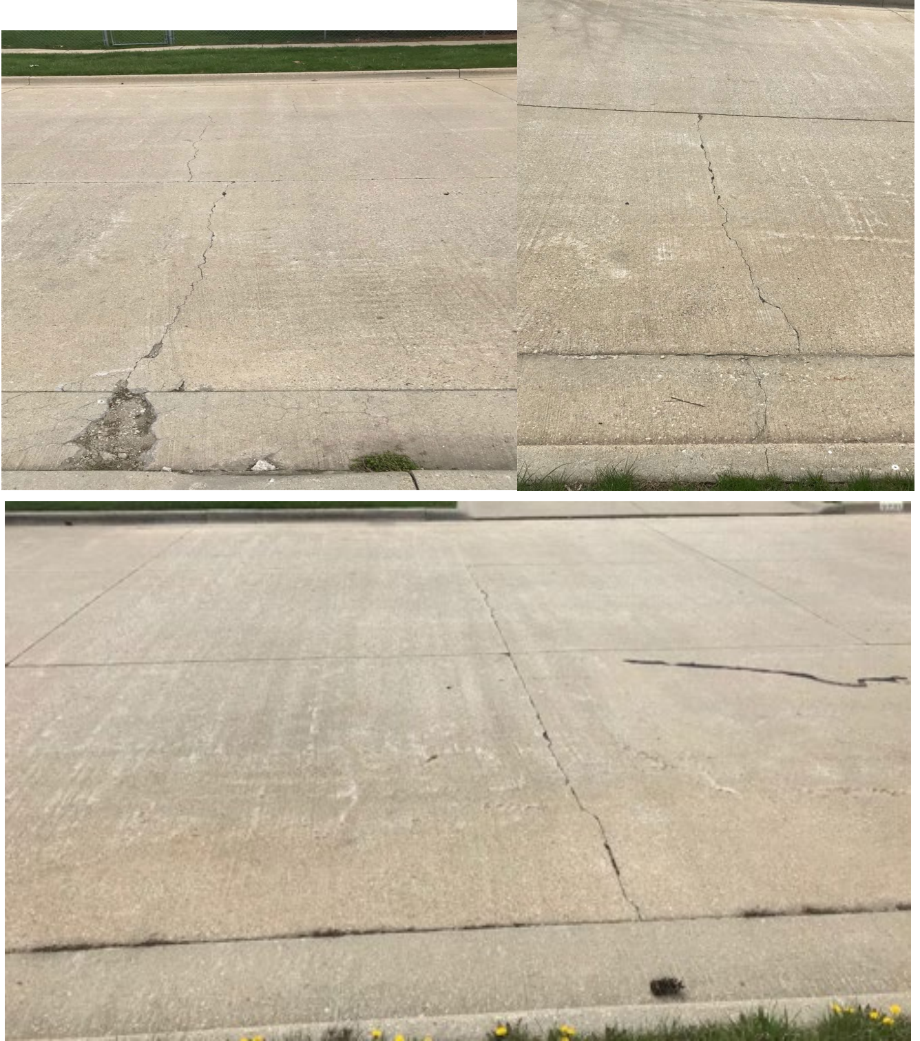
Figure 102. Photos. Slaydon Drive.
