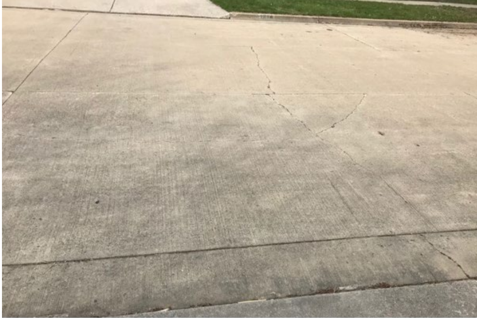
Figure 103. Photos. Challis Drive.
