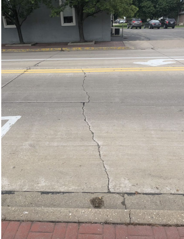
Figure 60. Photos. Jefferson Street with Jackson Street.
