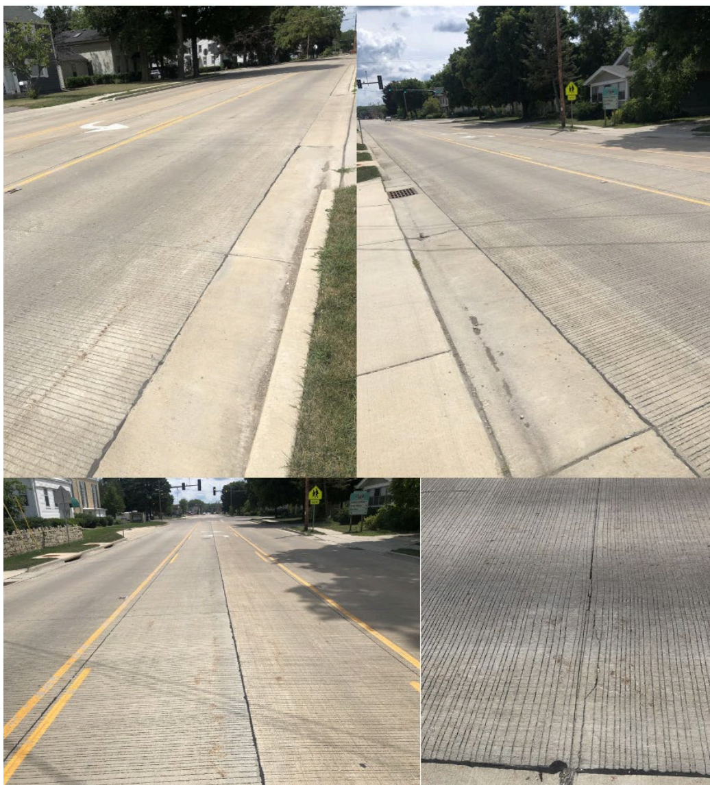
Figure 46. Photos. Union Street with Blackhawk Boulevard.
