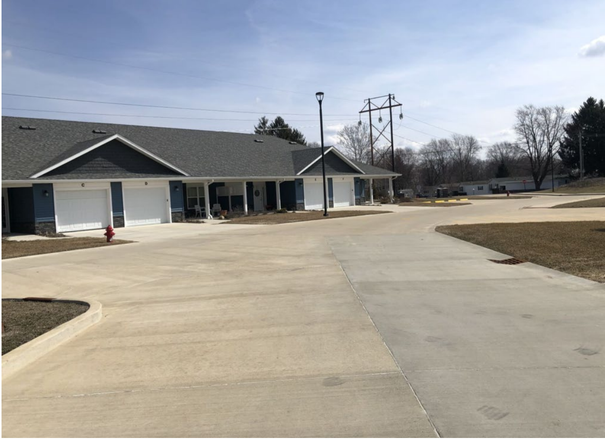
Figure 91. Photos. Forest View Drive.
