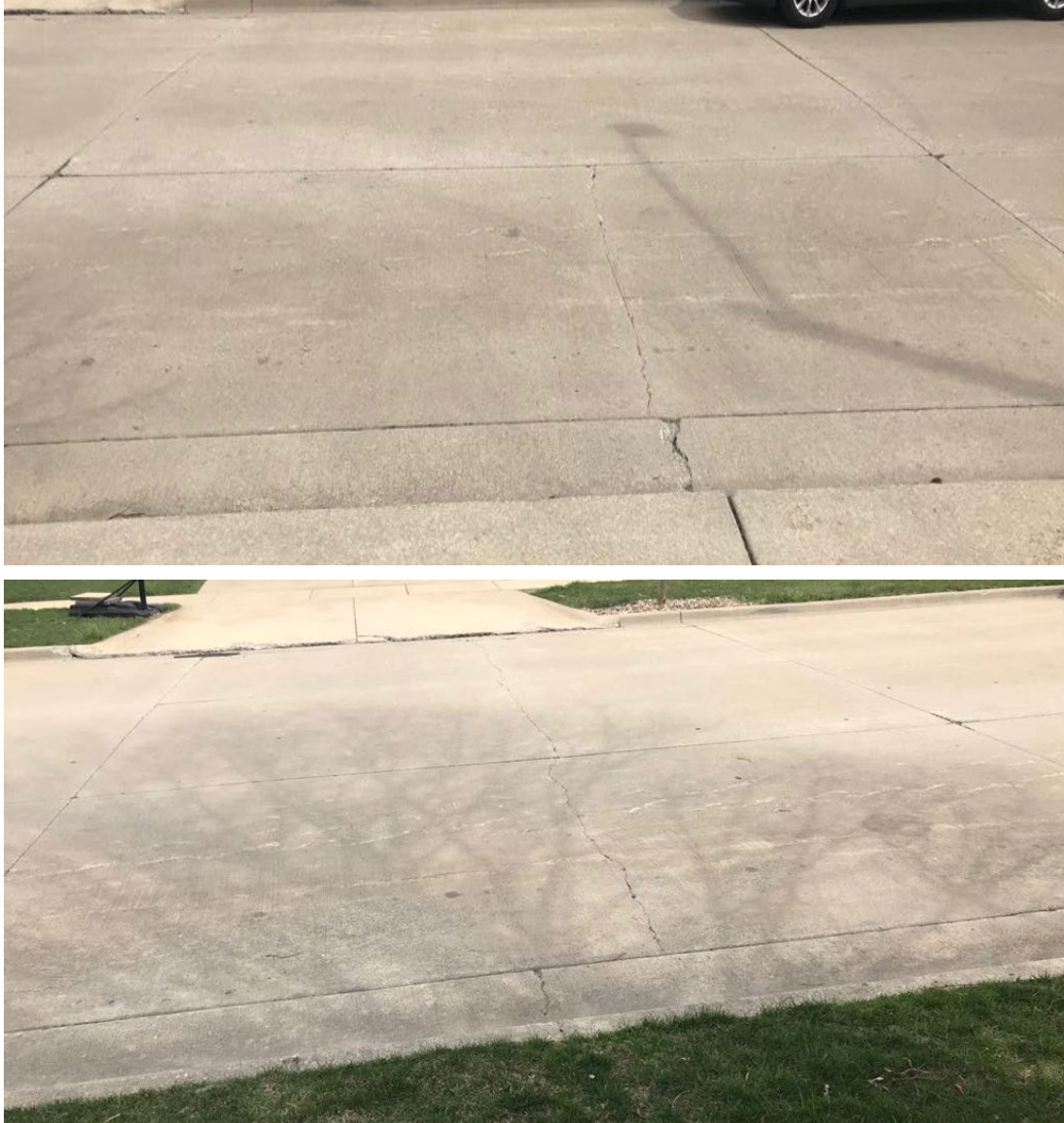
Figure 106. Photos. Newcastle Drive.
