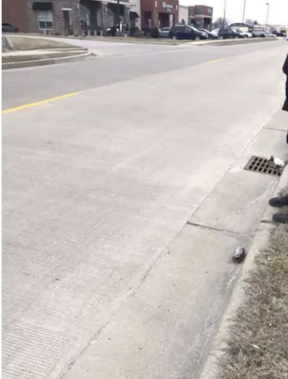
Figure 115. Photo. Merchant Street.
