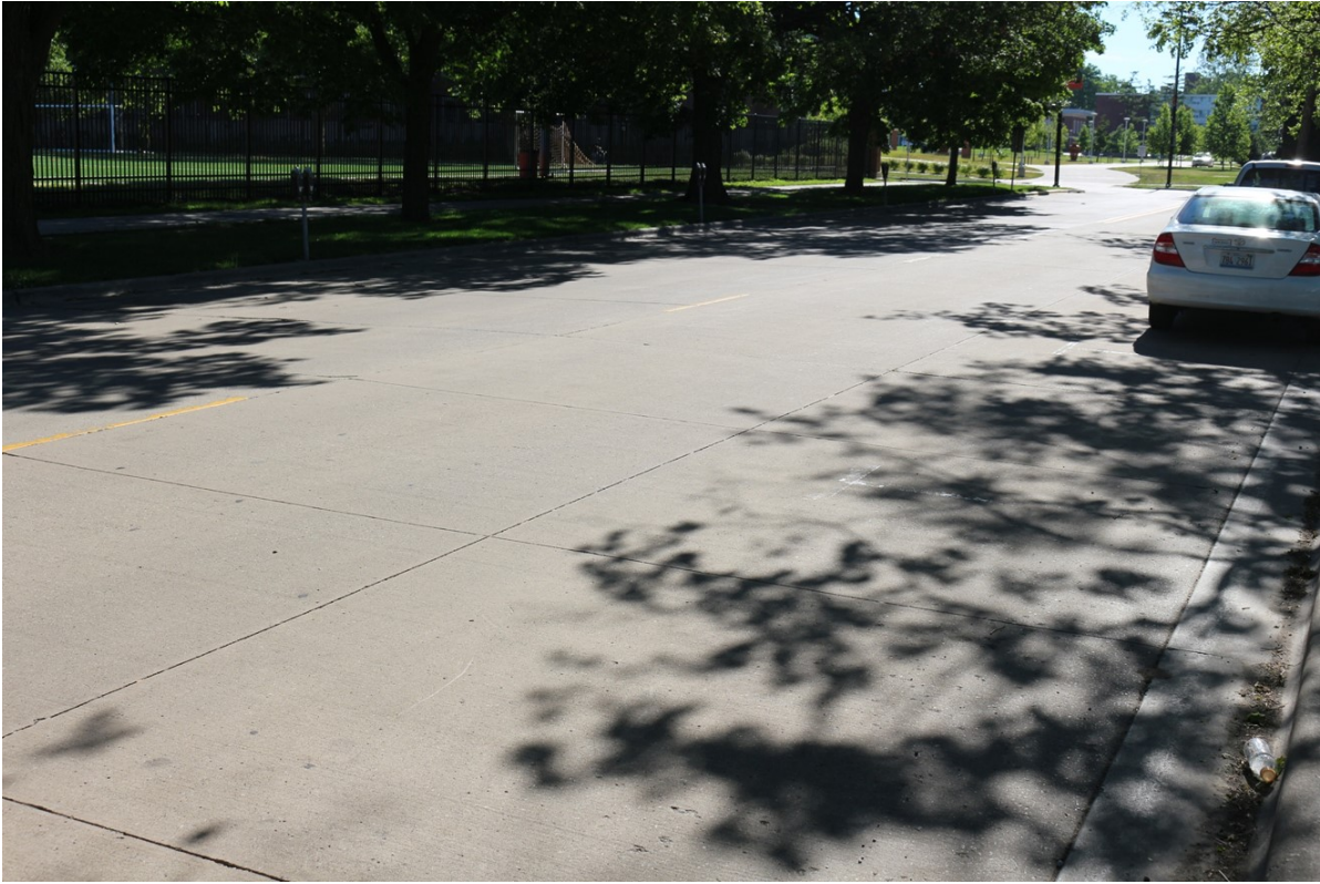
Figure 80. Photos. Stadium Drive.
