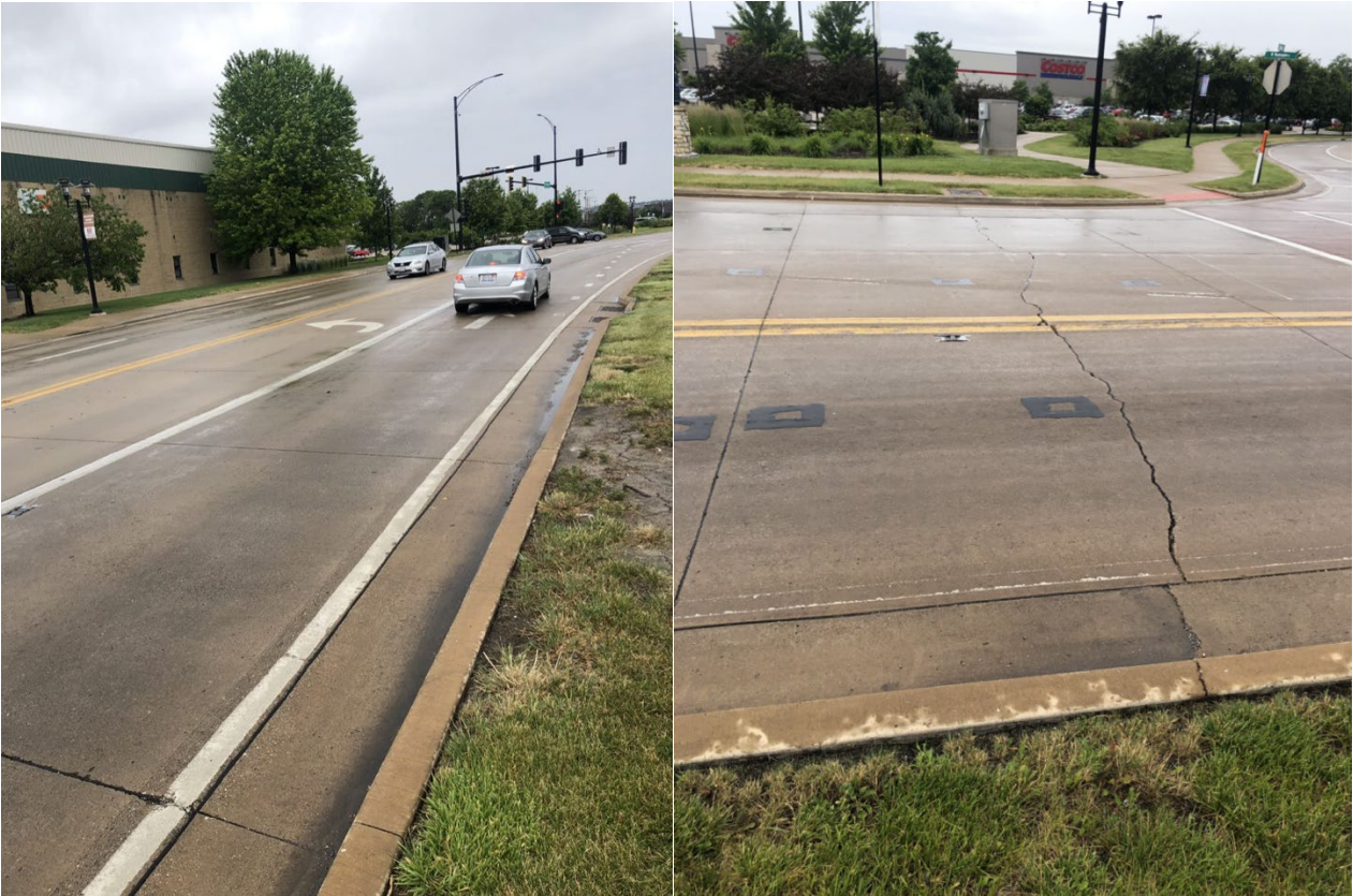
Figure 57. Photos. MacArthur Highway with Richland Street.
