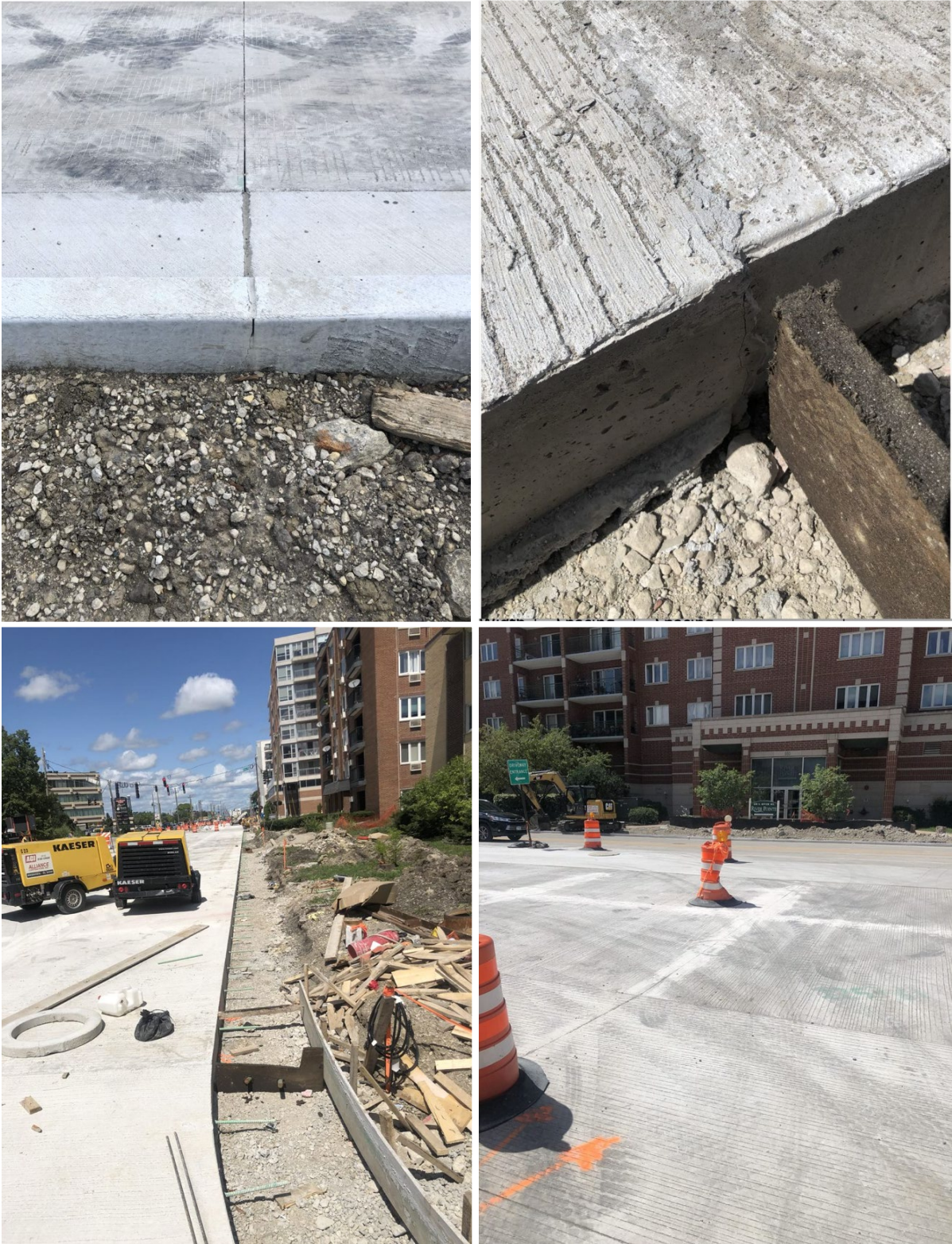
Figure 44. Photos. River Road (under construction).
