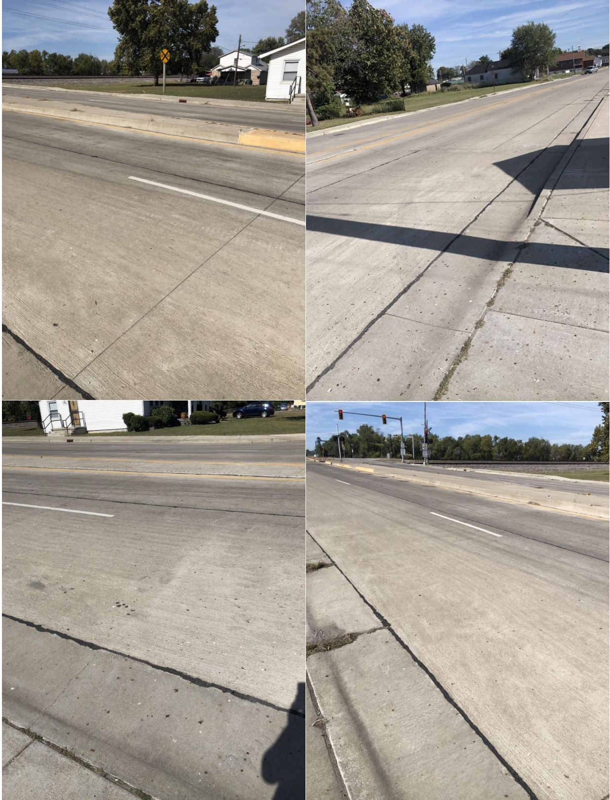
Figure 123. Photos. Bissel Road section 2.
