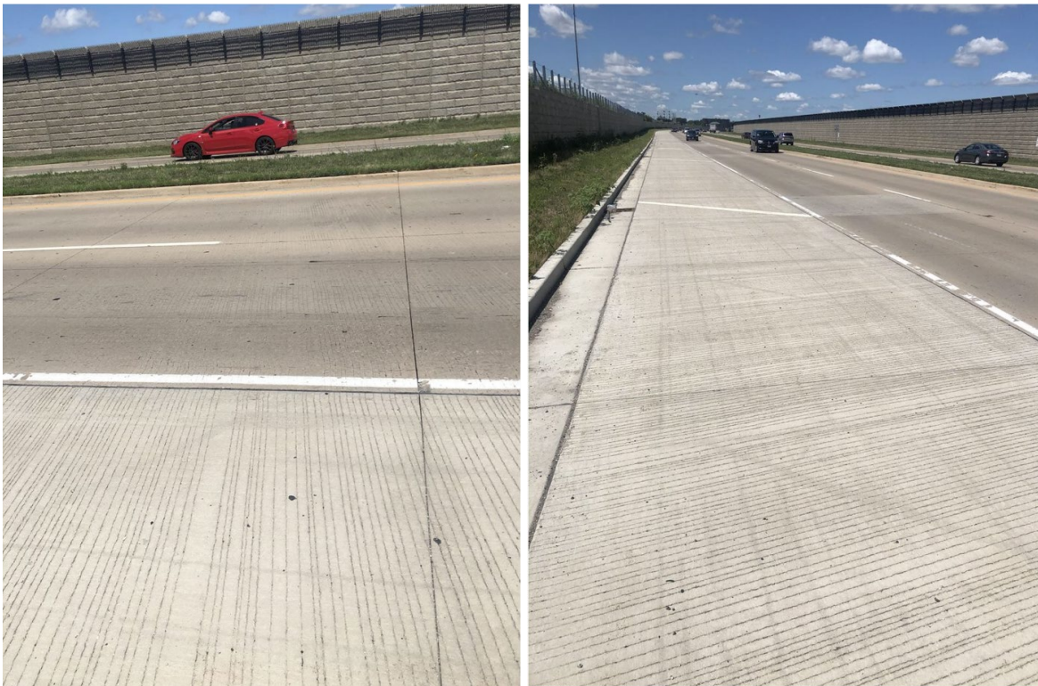
Figure 43. Photos. IL 19 and York Way.
