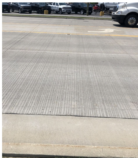
Figure 11. Photo. IL 59 section constructed approximately in 2010 (no distress).
