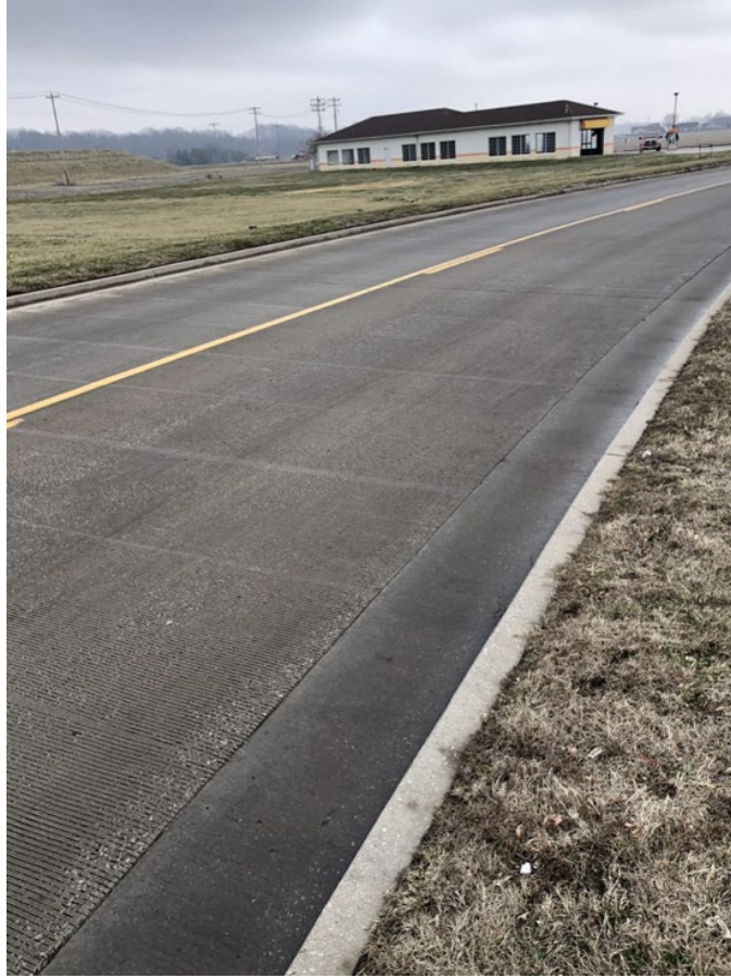
Figure 116. Photos. Harrison Street with Wesley Drive.
