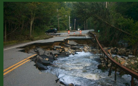
Roadway washout in the Lake Champlain Basin during Tropical Storm Irene. Photo credit: Tom Woodman
