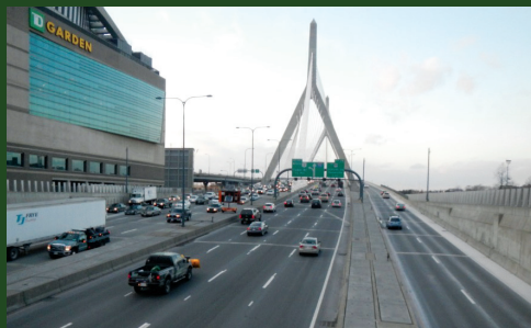
Tip O'Neill Tunnel northernmost portal. Photo credit: MassDOT
