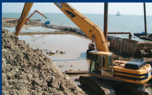
Levee construction. Photo courtesy of MTC.
