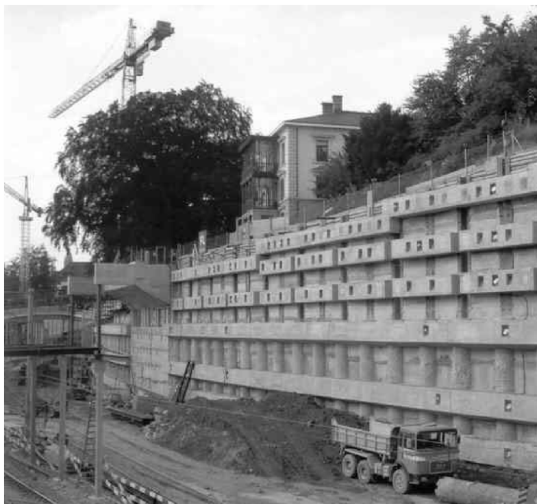
Figure 3. Photo. Encapsulated anchorages in retaining wall adjacent to Stadelhofen Railway Station, Zurich.
