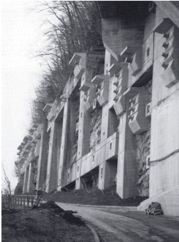
Figure 4. Photo. Electrically isolated anchors in stabilized rock cuts at the Seelisburg Tunnel.
