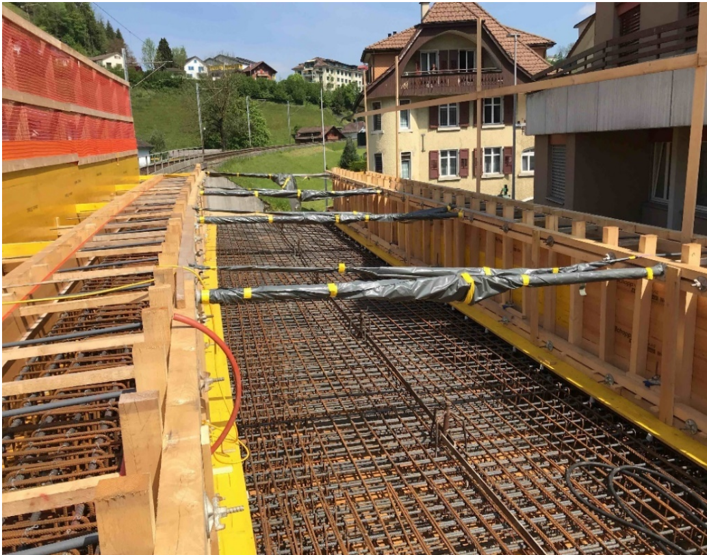
Figure 19. Photo. Formed through-through-girder with reinforcement and PT ducts in place, awaiting concrete.
