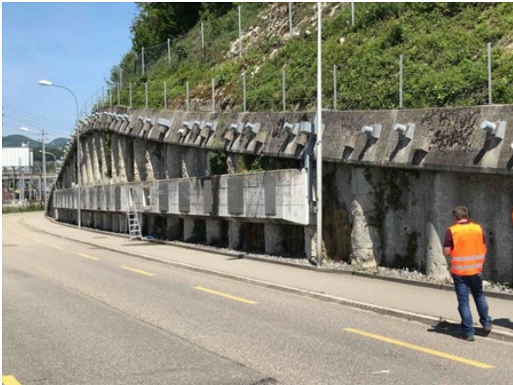
Figure 5. Photo. Overview of in-service ground anchor wall containing EIT ground anchors in Olten, Switzerland.
