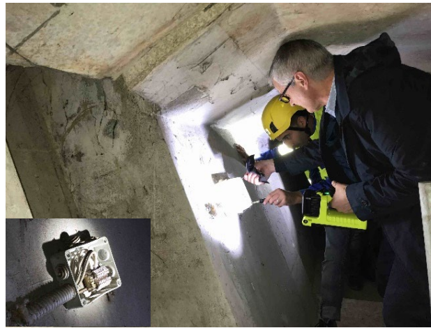
Figure 27. Photo. Engineers inspecting an EIT junction box; inset is close-up of the junction box.
