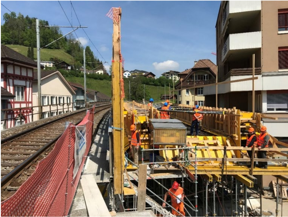
Figure 18. Photo. New post-tensioned concrete superstructure being formed adjacent to an in-service rail service rail bridge.
