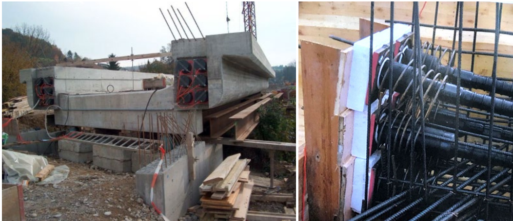
Figure 24. Photo. Construction of the Mittelmuhlen Bridge showing end of span with EIT wires extending from anchorage caps (left) and PT anchorage assemblies prior to concrete placement (right).
