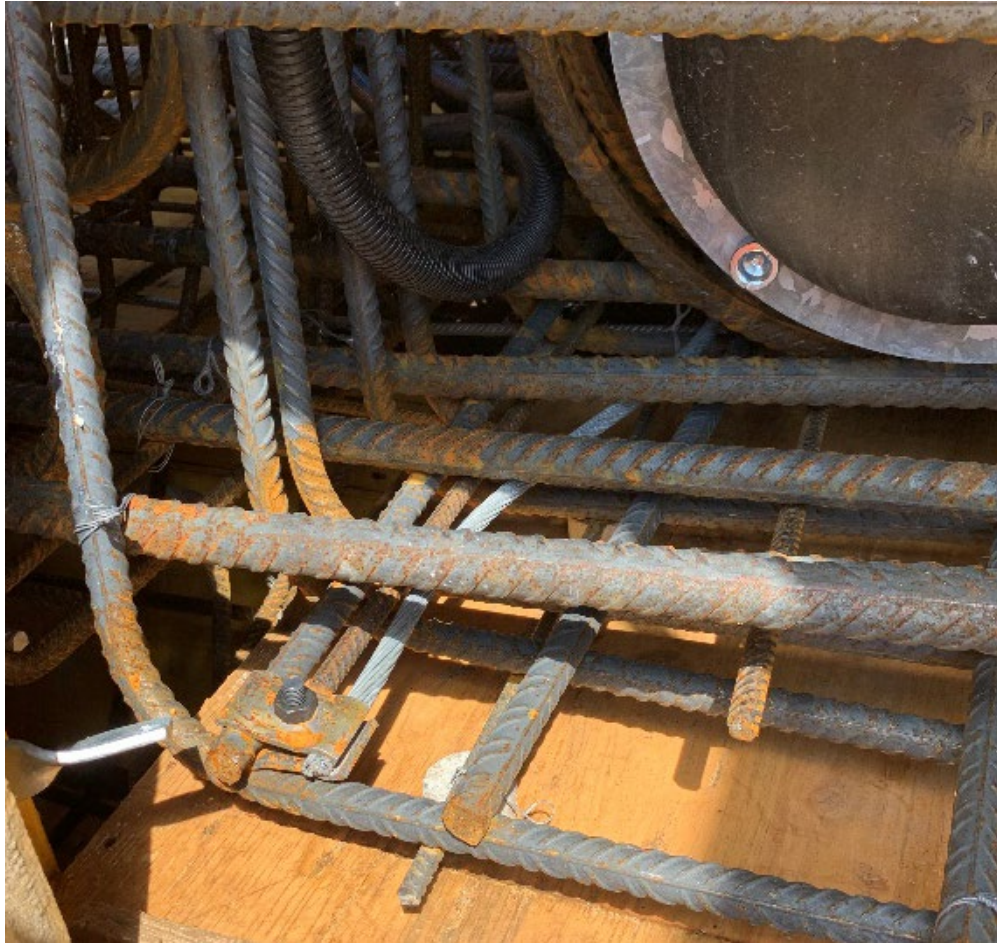
Figure 21. Photo. Grounding wire attached to steel reinforcement cage.
