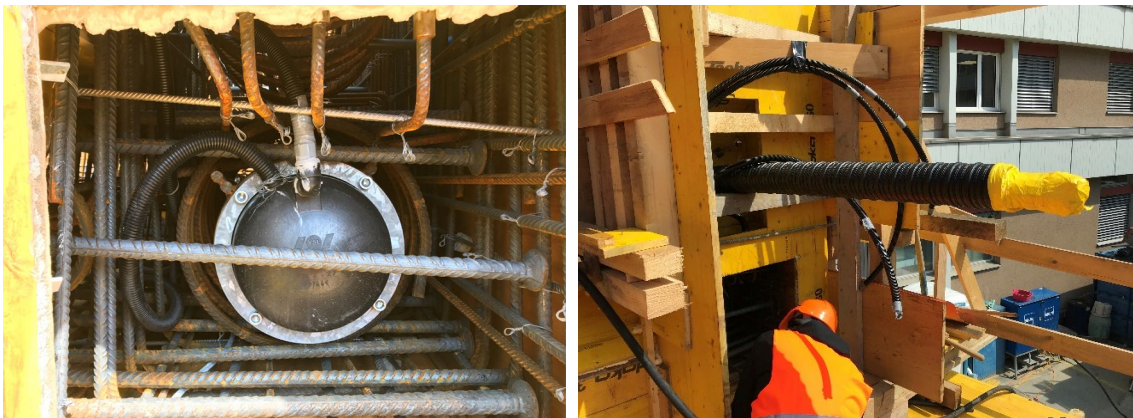
Figure 20. Photo. Post-tension assembly awaiting concrete; dead end (left) and live end (right).
