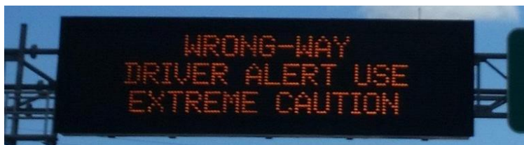
Figure 6-4: Wrong-way Driver Alerts on Dynamic Message Signs in Florida (Source: DHSMV, 2016)
