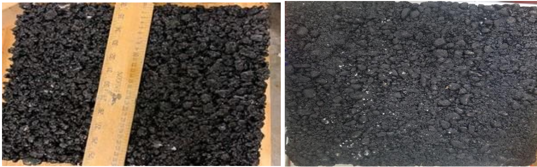
Figure 14. Photos. OGFC-12.5 (left) and Superpave-12.5 (right) pavement slabs.
