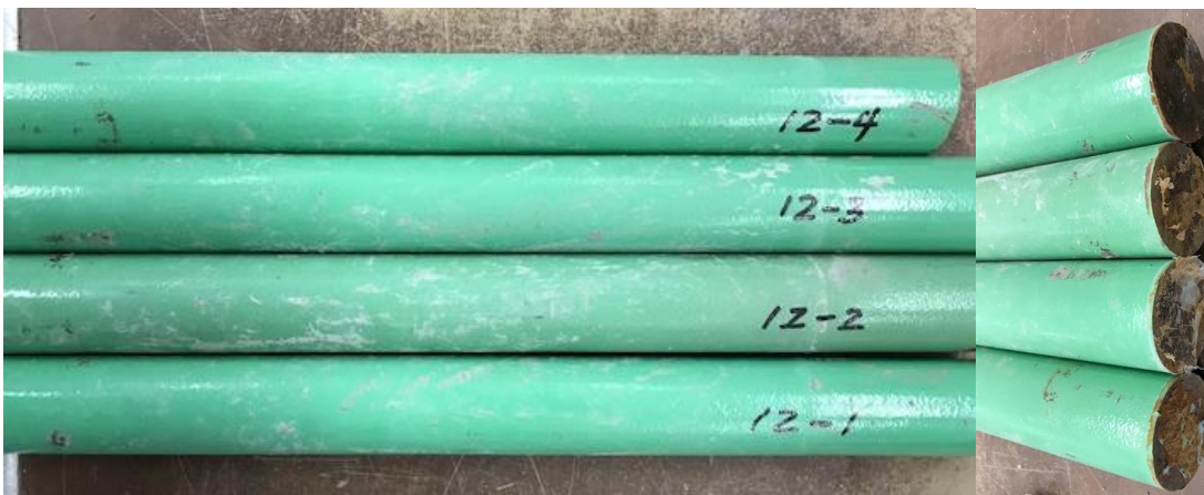
Figure 50. Photo. Dowel bars after corrosion test.
