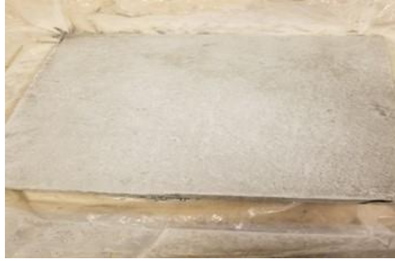
Figure 15. Photo. Portland cement concrete slabs.
