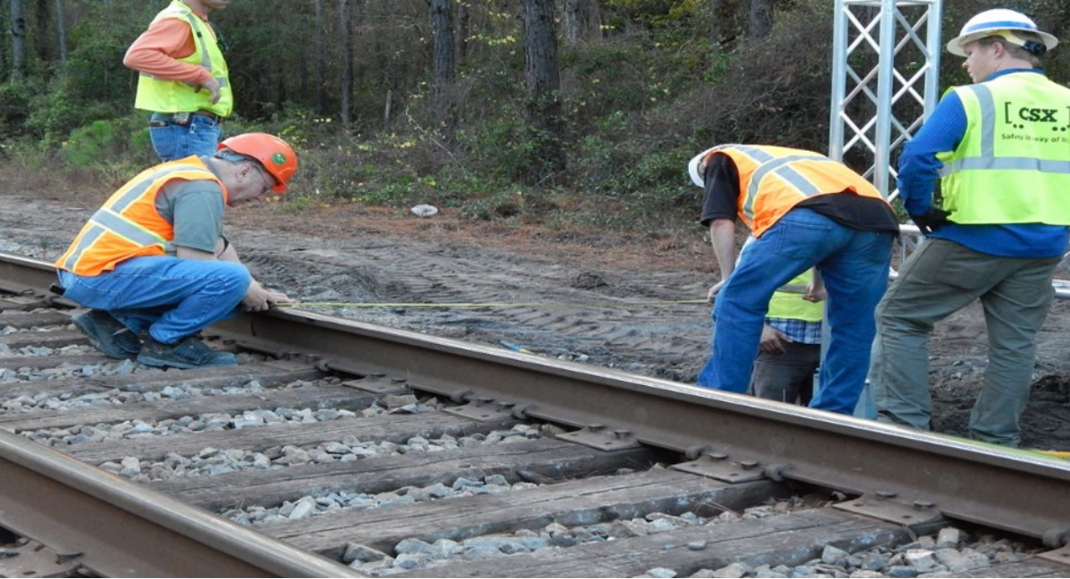
Figure 2. Installation Team Positioning Stanchions
