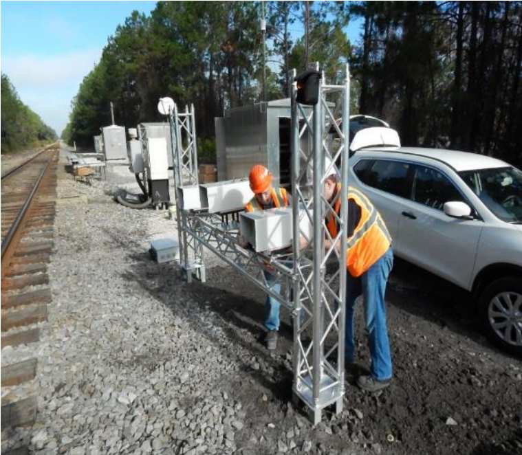
Figure 6. Installation of Axle-level Cameras at Hague Site
