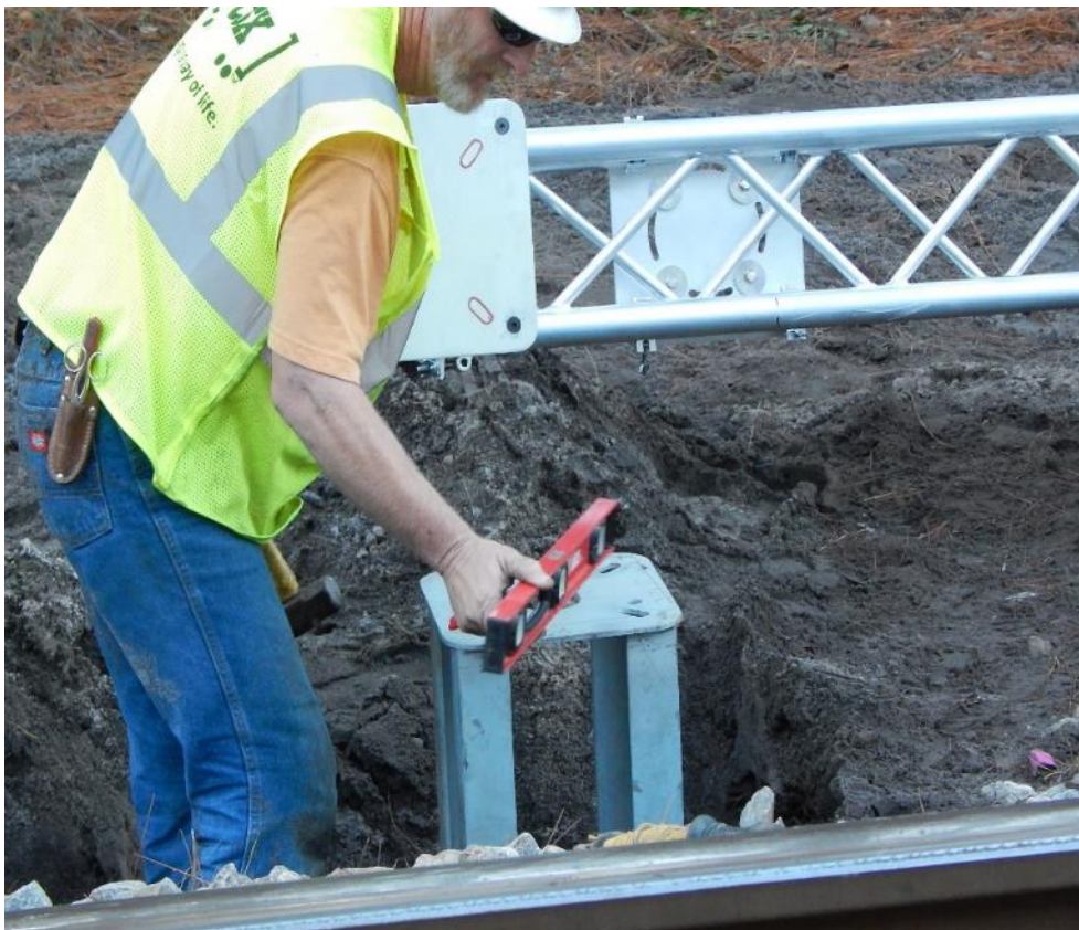
Figure 1. Installation and Leveling of the Foundation Pylons for the Camera Stanchions
