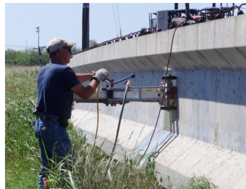
Figure 4. TxDOT worker extracting cores for further testing.
