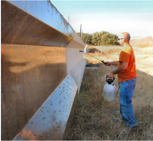
Figure 3. Topical application of silane using a handheld garden sprayer (left); view of girder after treatment (right). Only half of each girder was treated with silane.
