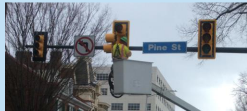
Upgrading 8" to 12" signal heads
