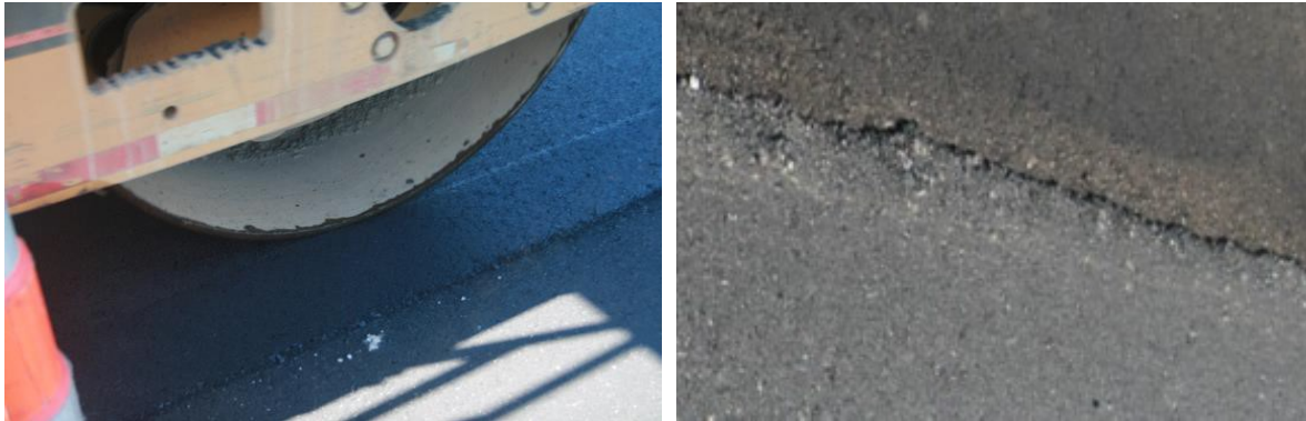
Figure 3. Butt joint construction with hot pinch on US 61
