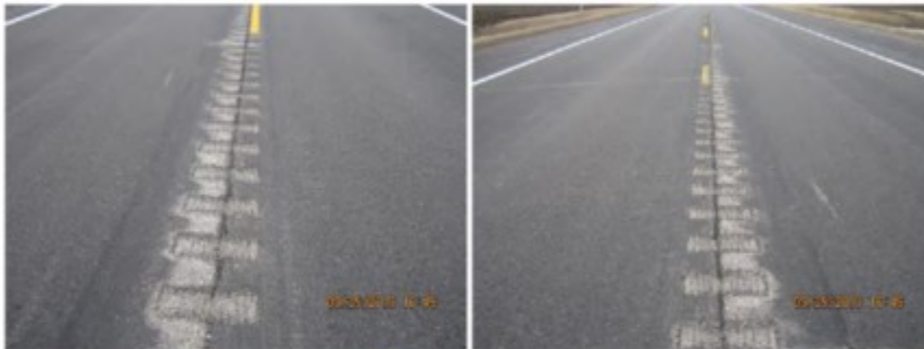
Figure 3 Longitudinal Joint Adhesive US 169. Good condition.
