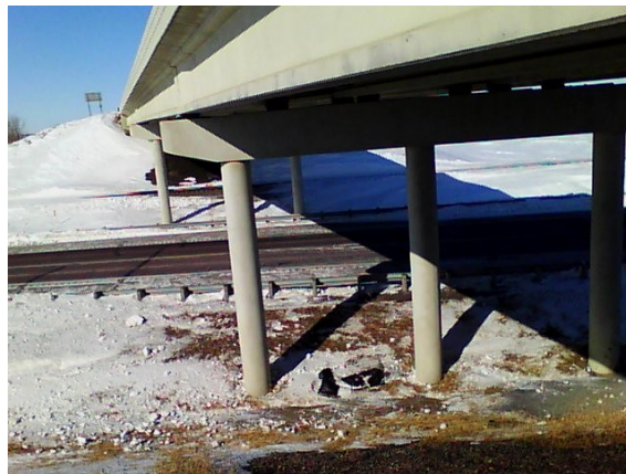
Figure 18: Pavement temperature differential of 28° F caused by shadow under bridge. Differential occurs over a roadway travel distance of approximately 4 feet. MN 23, Florence Bridge location, February 20, 2020. Air temperature 7° F, light intensity 5198 lumen.
