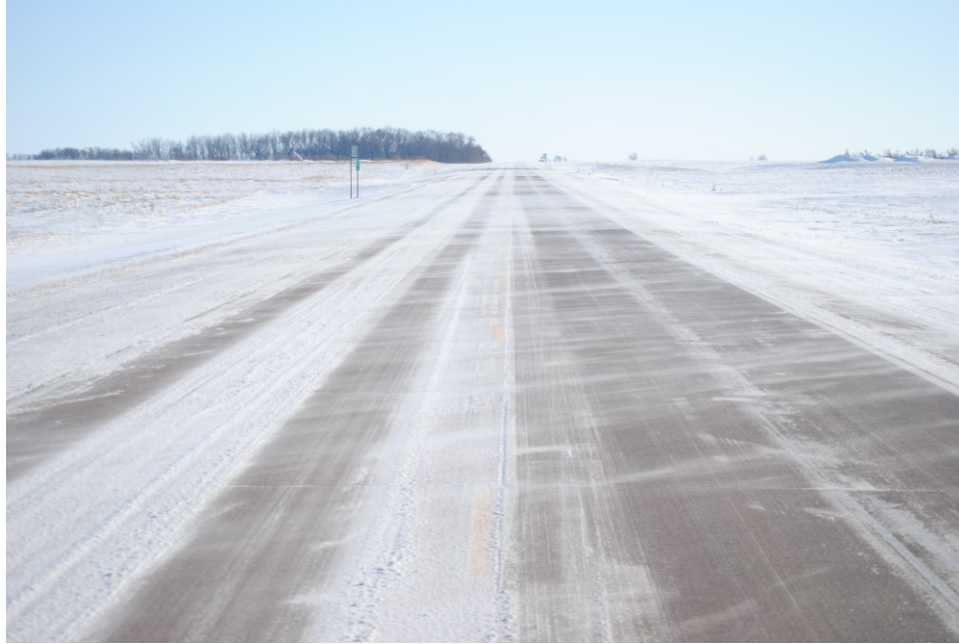
Figure 9: Drifting on roadway, with compaction developing due to vehicle transit through drifting snow at a control site on a clear day. Sanborn location, February 20, 2020.
