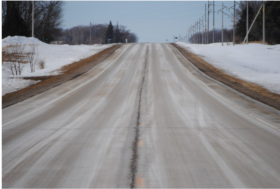
Figure 14: Salt residual on pavement. Rice Lake location, February 25, 2020.
