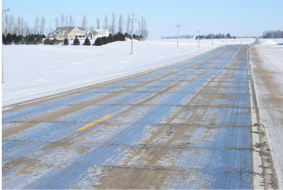
Figure 10: Compaction on roadway. TH 22, 0.5 mile north of Wells Bridge location, February 13, 2020.
