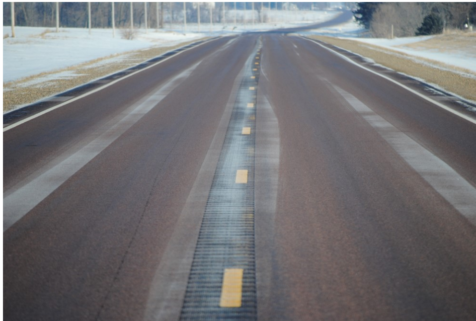
Figure 13: Ice fog-deposited roadway ice visible outside of wheel tracks. Waldorf location, December 19, 2019.
