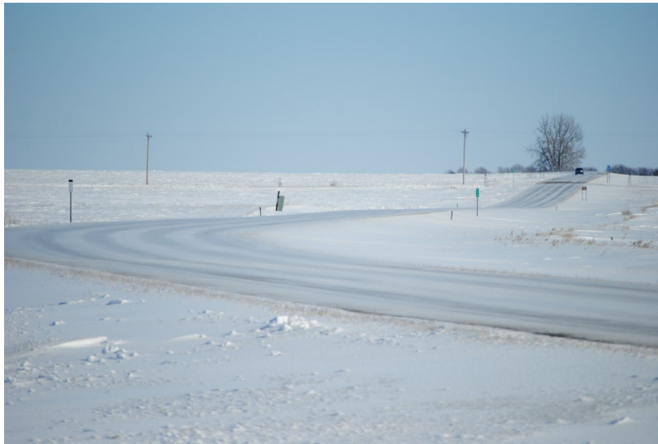
Figure 15: Blow ice on roadway, formed by dry snow drifting across sunlight-warmed pavement, melting then refreezing during deposition. TH 30, 2 miles east of Currie, MN, February 20, 2020
