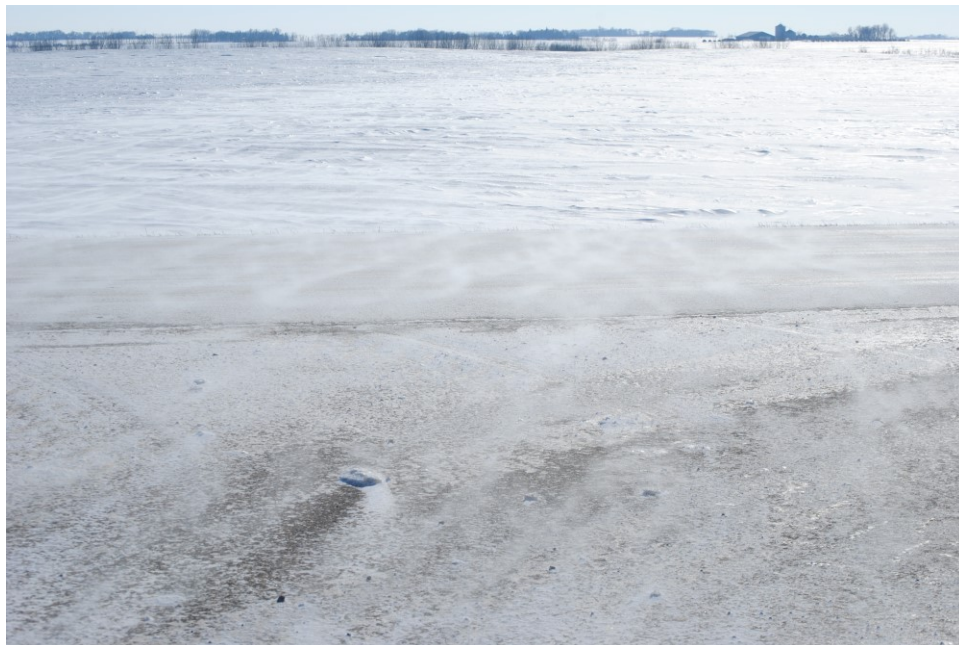
Figure 16: Dry snow drifting across sunlight-warmed pavement forming blow ice on roadway. TH 30, 2 miles east of Currie, MN, February 20, 2020
