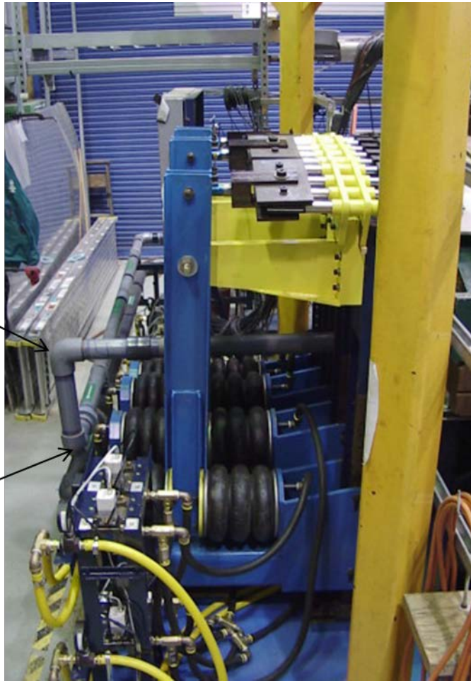
Figure 9. Photo of Adjustment of Water Supply PVC Piping
