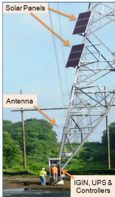
Figure 2: Typical ADLS Site on Susquehanna-Roseland Line on fiber/radio hybrid network.
