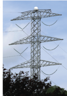
BELOW: HARRIER Utility tower installation
