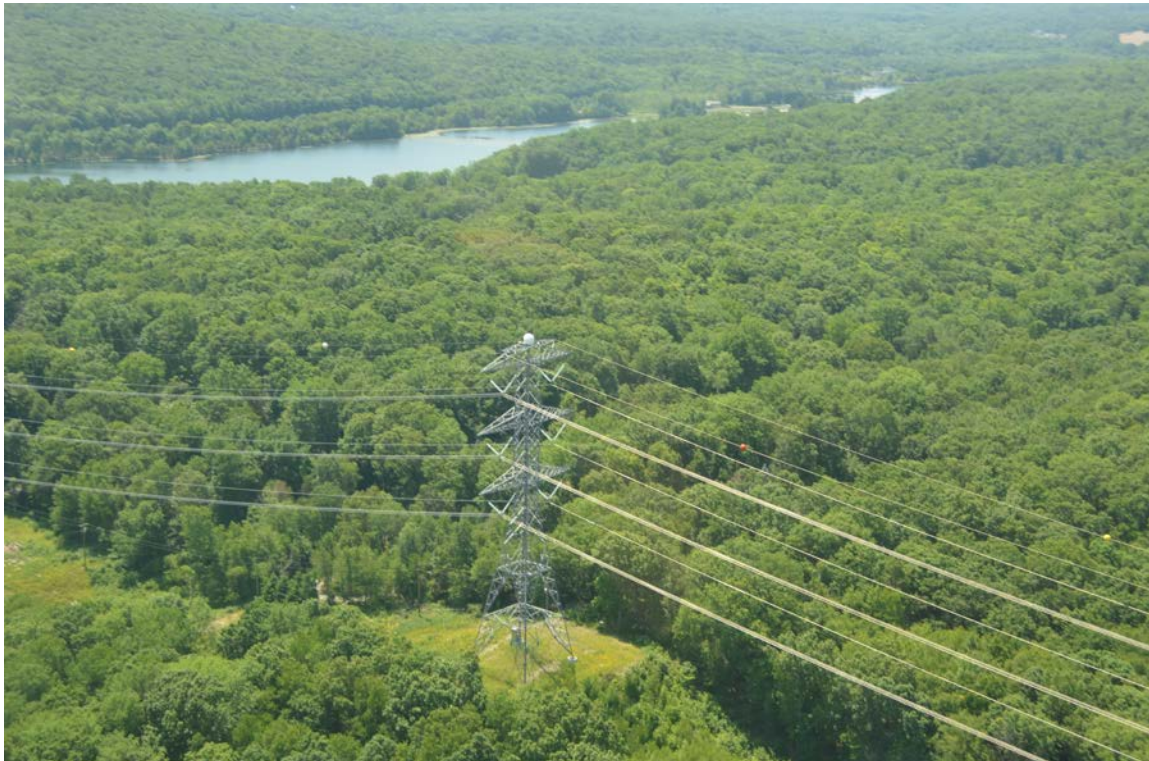
Figure 14. The HSR-02 Installed on Transmission Tower 53/5
