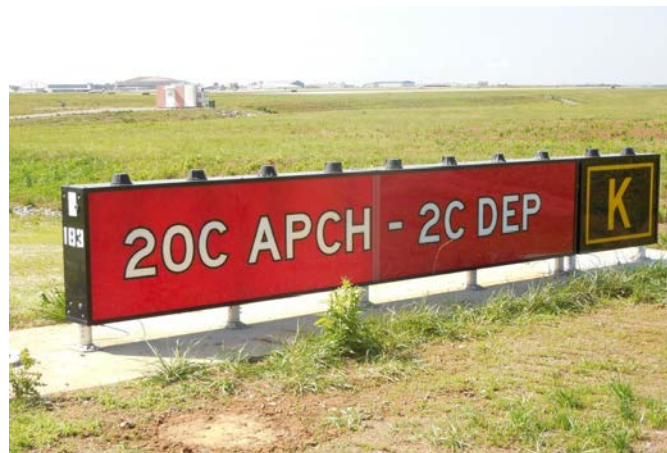
Figure 14. Installed Proposed Signage at BNA
